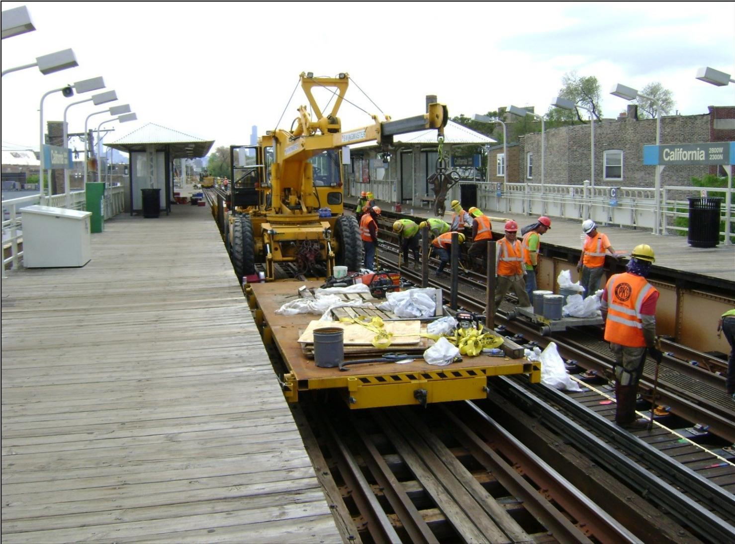
**Clipping Rail to New Plates – SB California Station**
