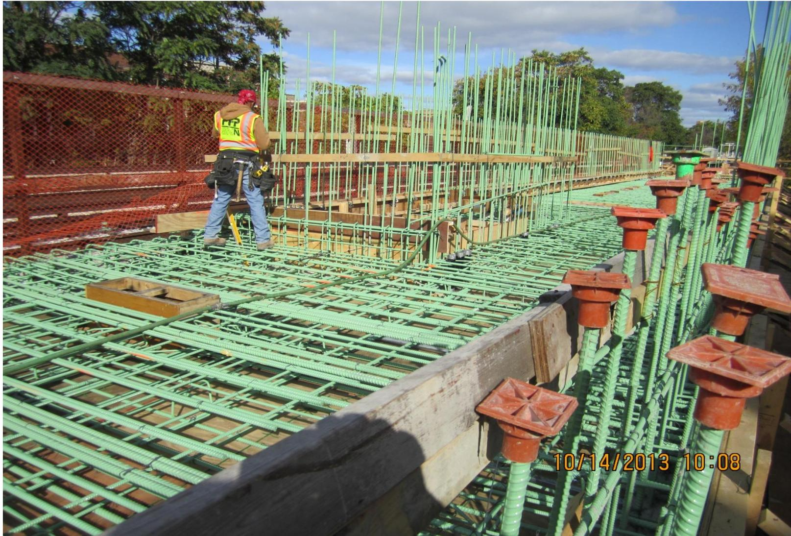
Farwell substation 2<sup>nd</sup> floor rebar installation
