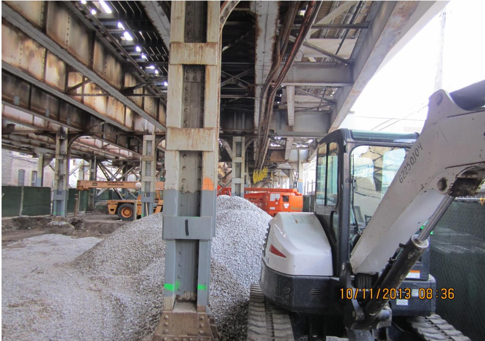
**Armitage Substation excavation and column replacement preparation**
