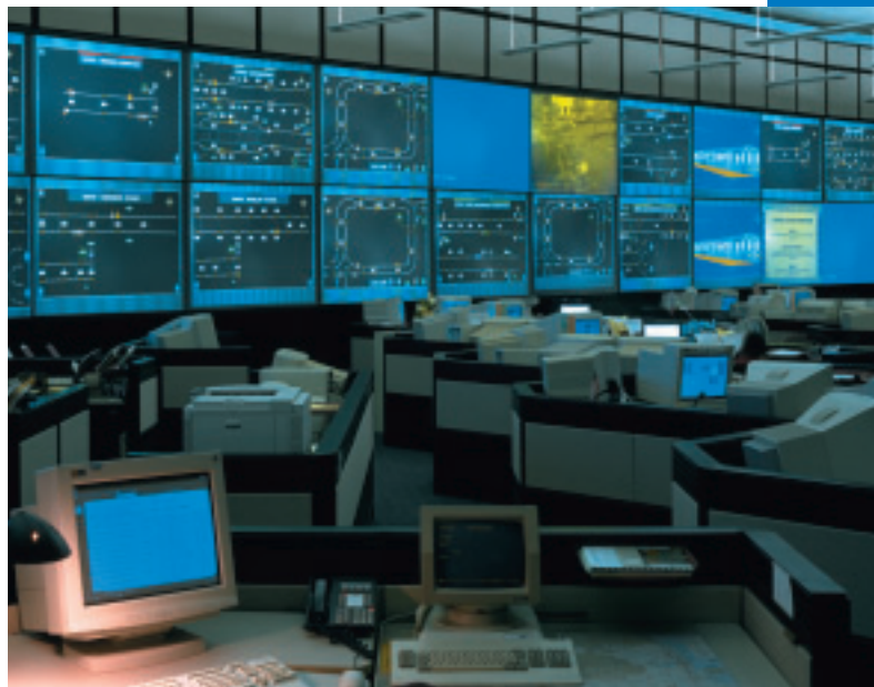
CTA's Control Center constantly monitors trains and buses in service throughout the area.
