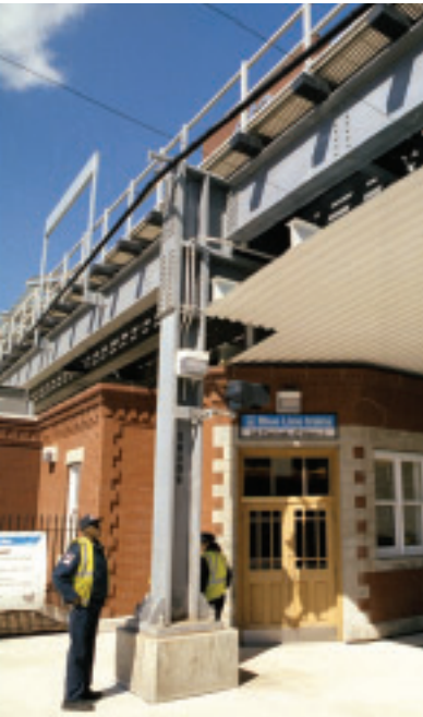
The newly renovated Kedzie station on the Cermak branch of the Blue Line.
