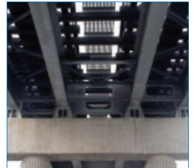
The American Galvanizer's Association (AGA) presented its 2004 Excellence Award to CTA. More than 13,000 tons of structural steel were covered with galvanized zinc, which coats and protects the steel from moisture, rust and corrosion.
