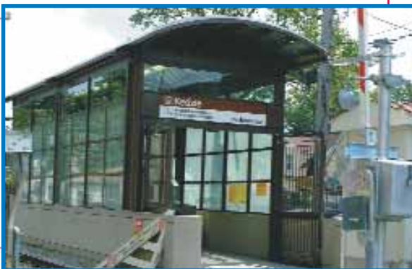
Renovations at the Kedzie Brown Line station include the addition of an auxiliary entrance at Spaulding Avenue.
