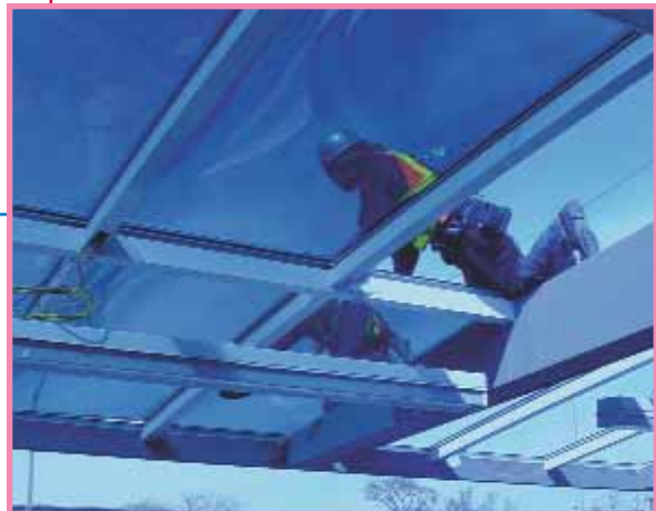
New canopies were installed on platforms as part of the rehabilitation of the Dan Ryan branch of the Red Line. Above, crews complete the installation at 63rd Street station.
