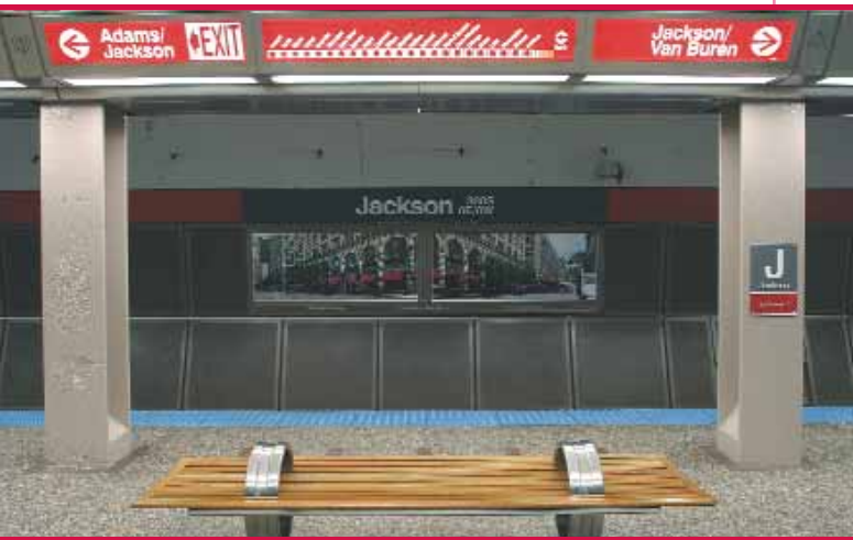
The Chicago Department of Transportation's $16.9 million investment in the reconstruction of the Red Line's Jackson platform includes new lighting, acoustical panels and new street identifier signs.
