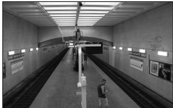
After: When work was completed, riders at the station noticed many improvements, including masonry walls and concrete ceiling repairs, refurbishment of the Kedzie main entrance and Spaulding auxiliary entrance escalators, and deep cleaning and repainting.
