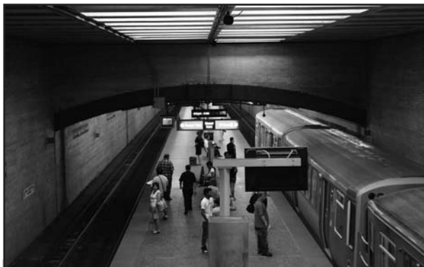
Before: The platform at the Logan Square Blue Line station was dark and in need of repair prior to work under the Station Renewal program being completed.
