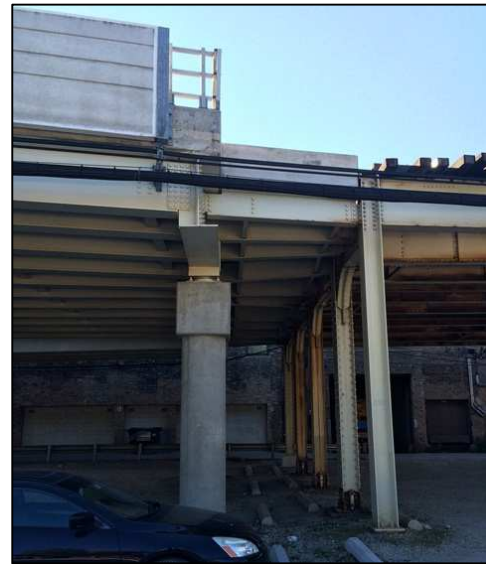
Figure 3-8: Photo Showing Transition between Newer Track Structure (Left) and Original Track Structure (Right) Just North of Belmont Station
