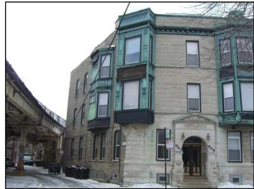
Figure 5-3: Vautravers Building (Facing South)
