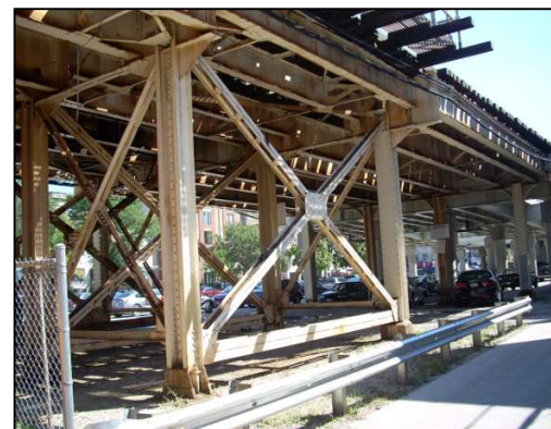
Figure 5-2: CTA Elevated Track Structure
