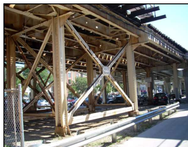
CTA Elevated Track Structure
