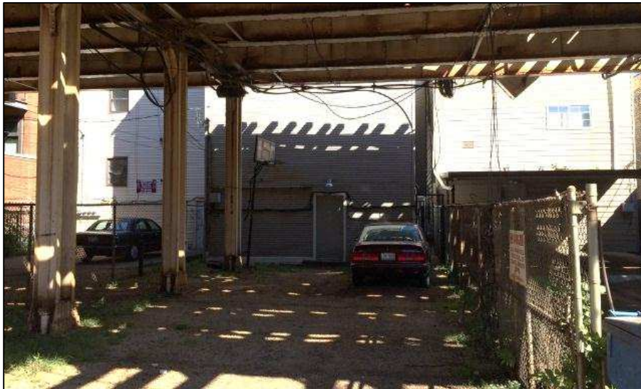
Figure 3-10: Photo of Area beneath Track Structure Used for Parking
