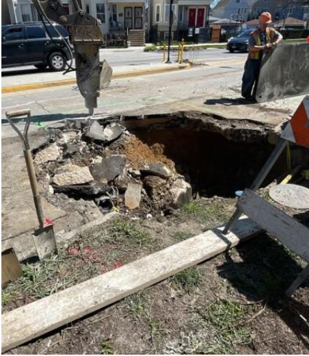
Excavator with breaker
