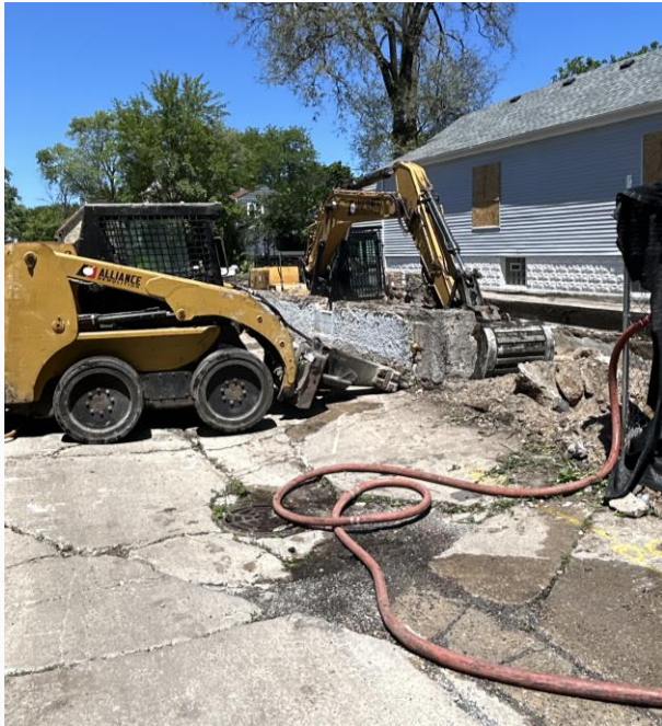
Skid steer with breaker attachment
