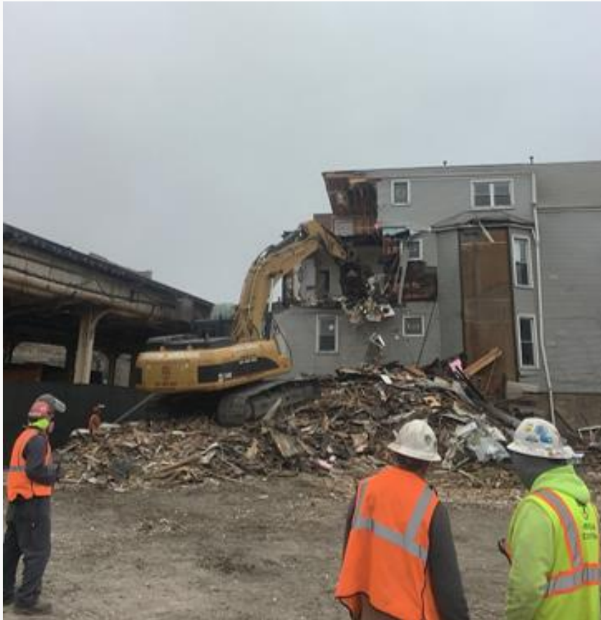
Property demolition for the Red and Purple Modernization (Phase One) Project north of Belmont, 2018
