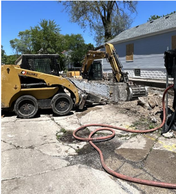
Skid steer with breaker attachment
