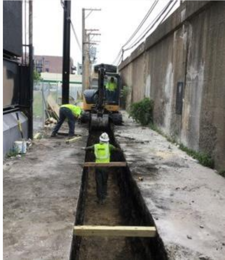
Relocation of utilities underground near Argyle, 2019
