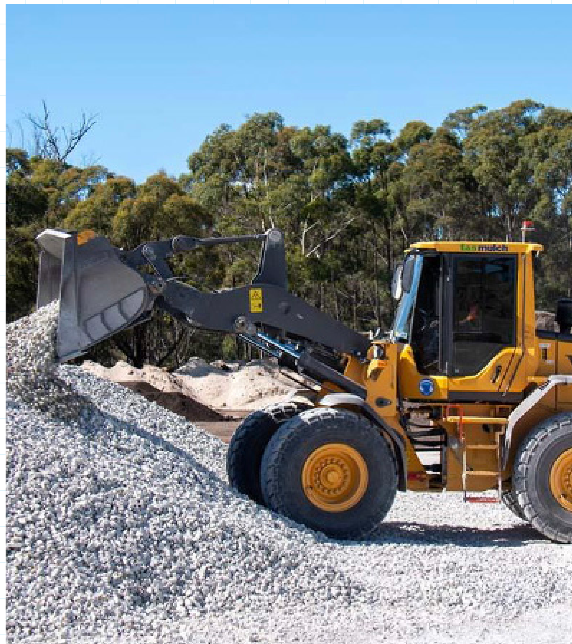
Site Preparation & Roadway Work
