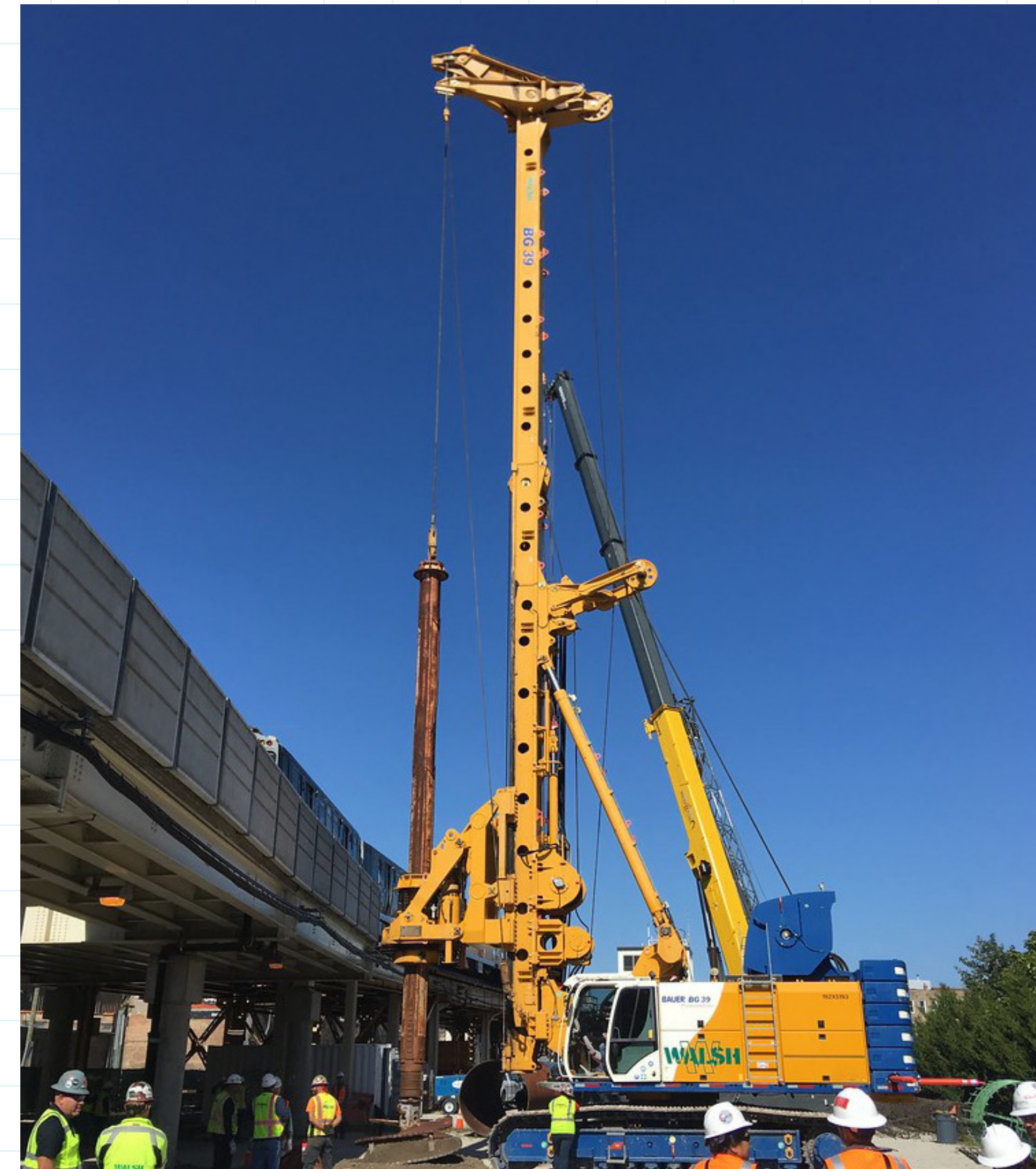
Drilling Deep Foundation for New Track Structure
