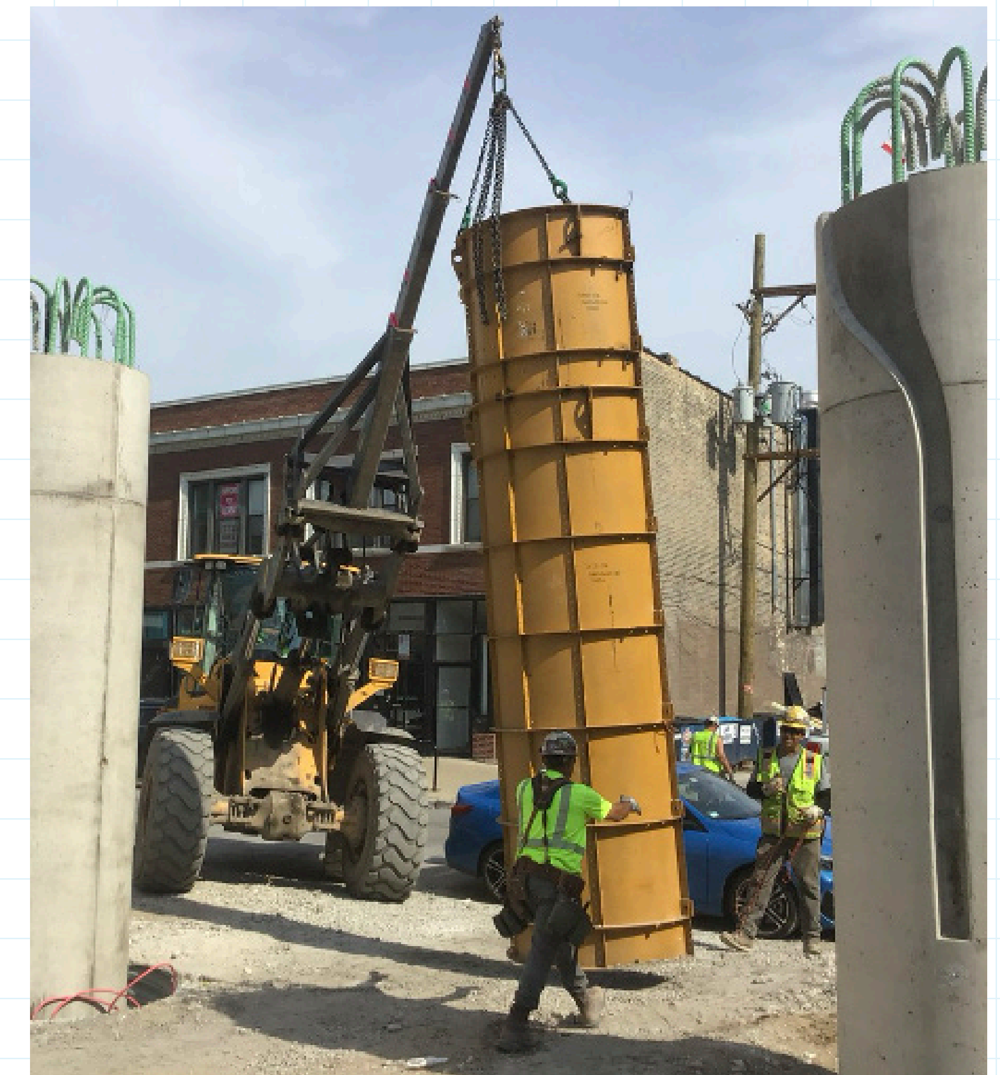
Pouring Concrete for Foundation & Columns
