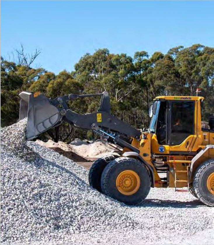
SITE PREPARATION & ROADWAY WORK
