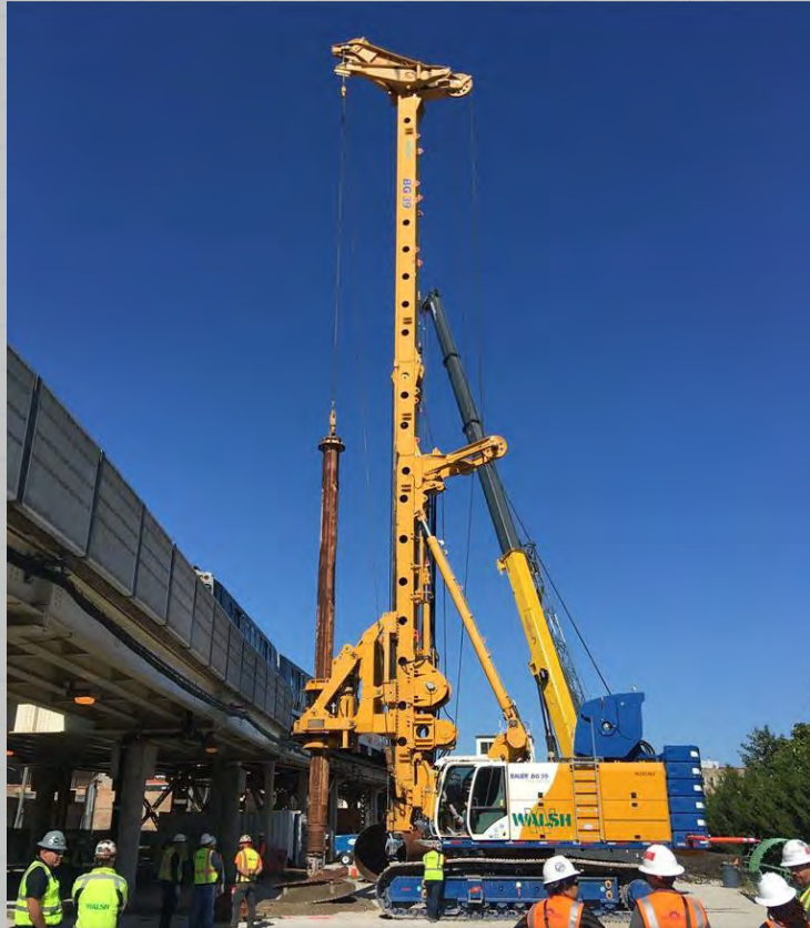
DRILLING DEEP FOUNDATIONS FOR NEW TRACK STRUCTURE
