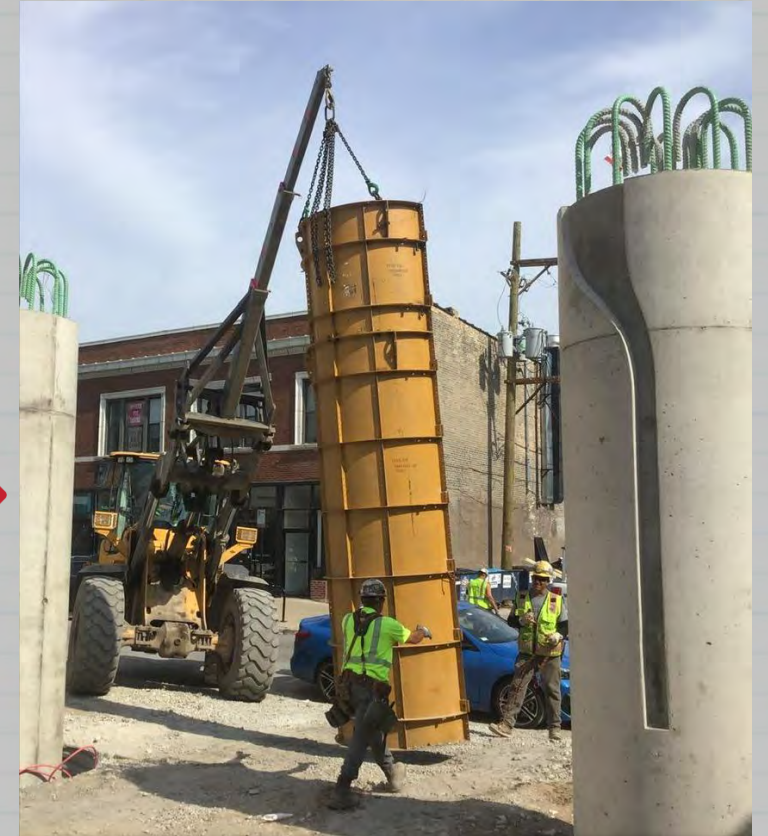
POURING CONCRETE FOR TRACK FOUNDATIONS & COLUMNS
