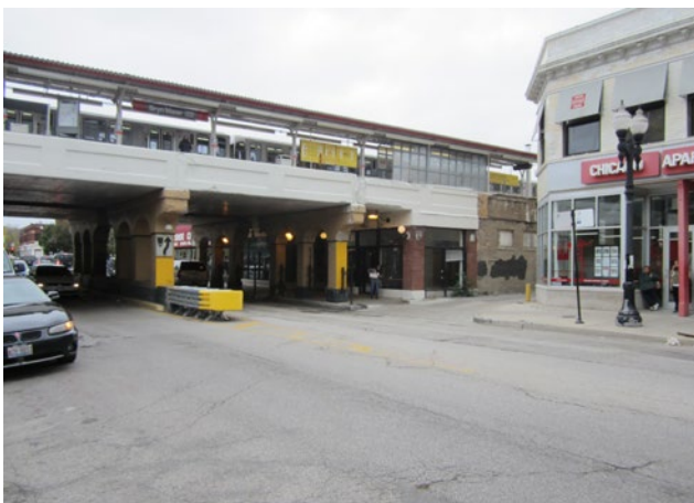
Existing Viaduct at Bryn Mawr Station
