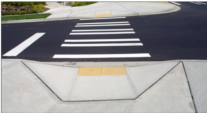
Color contrast crosswalk with curb ramps
