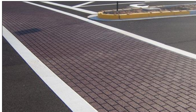
Color contrast crosswalk with tactile surface
