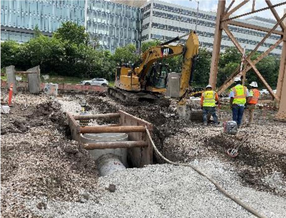
**Drainage structure installation near IMD**
