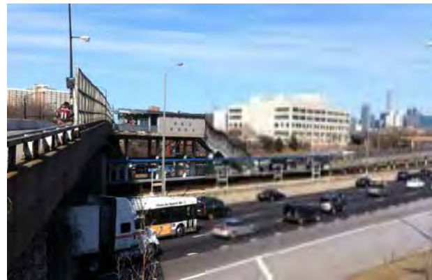
View of stationhouse at Ogden Avenue
