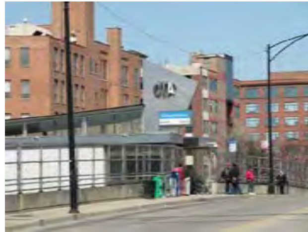
View of east stationhouse at Halsted Street
