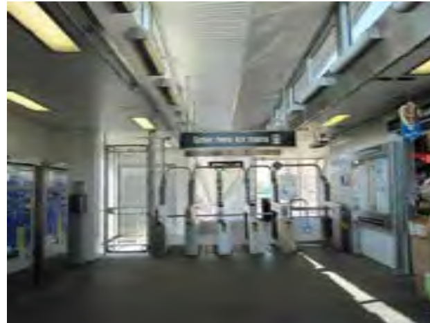
View of interior of east stationhouse at Halsted Street
