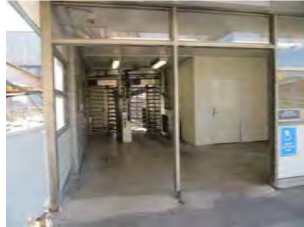
View of stationhouse entry at Paulina Street
