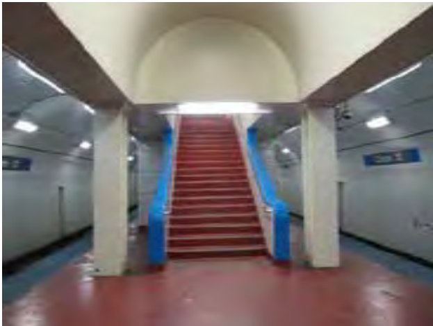
View of exit stair near east end of platform
