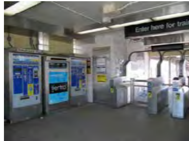
View of interior of west stationhouse entry at Morgan Street
