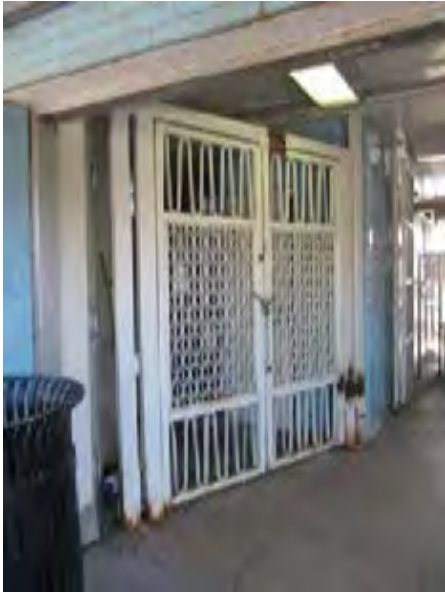
View of secondary stationhouse interior at Loomis Street
