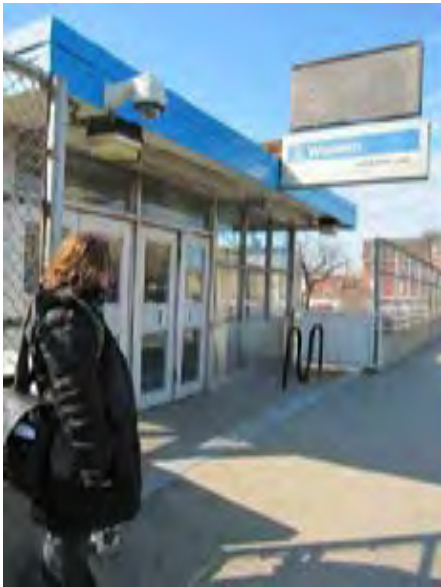
View of main station entry at Western Avenue
