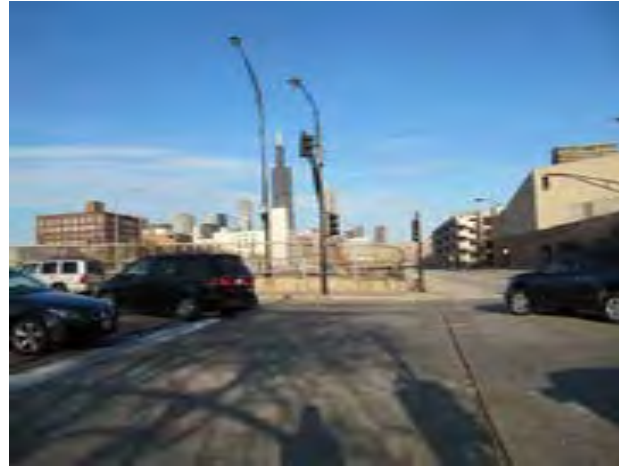
View of non-compliant curb ramp at Racine Avenue on approach to station. Note that there is no pedestrian crosswalk identified with stripping or signals
