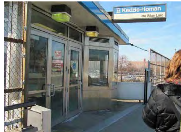
View of newer compliant entry doors at Kedzie Avenue Stationhouse
