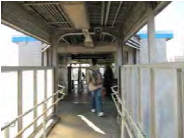
View of entry ramp at Homan Avenue stationhouse
