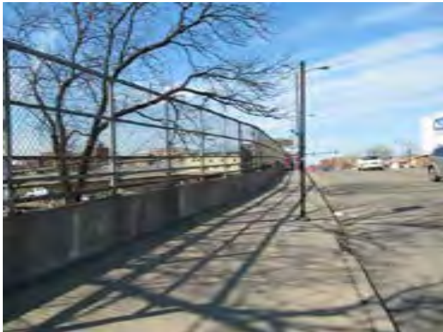
View of sidewalk along Western Avenue on approach to station
