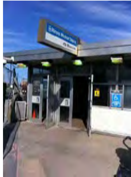
View of stationhouse entry at Ogden Avenue
