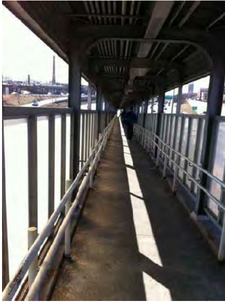
View of entry ramp at Kedzie Avenue stationhouse
