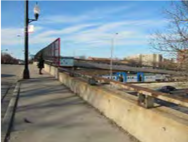
View of sidewalk along Loomis Street on approach to station
