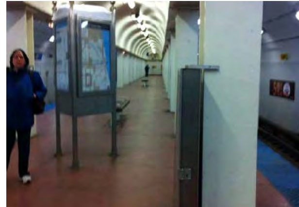
View of west end of platform showing long dead end area without means of egress.
