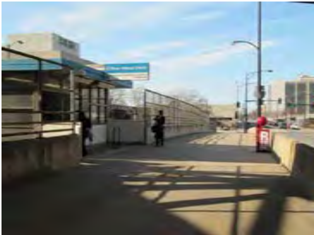
View of stationhouse entry at Paulina Street
