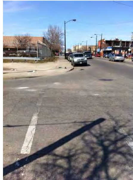
View of non-compliant curb ramp at Kedzie Avenue on approach to station. Note that the pedestrian crosswalk is not well identified with striping.
