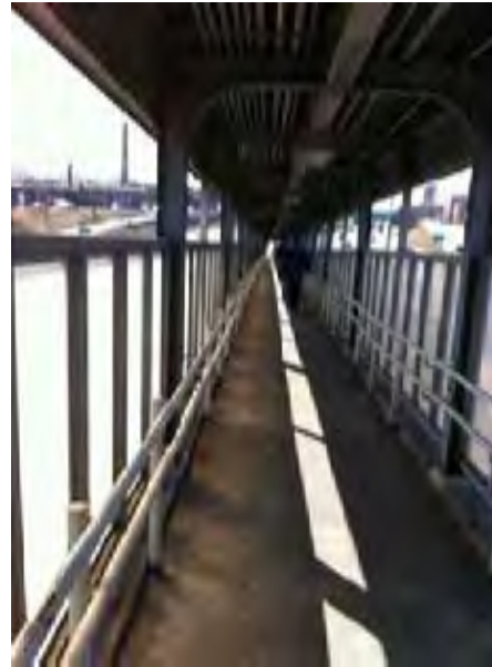
View of exit ramp at east end of platform
