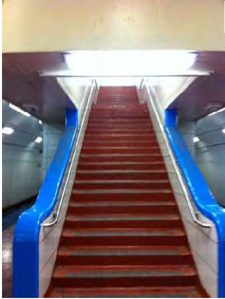
View of stair from platform up to paid area at Clinton station
