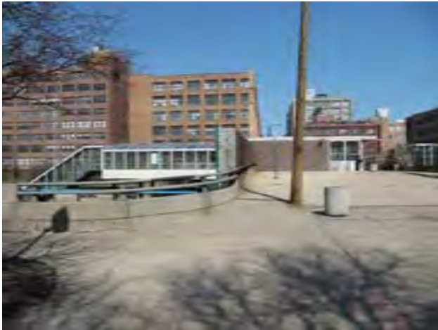
View of center stationhouse entry at Peoria Street
