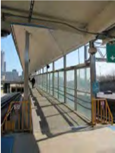
View of ramp exit at east end of platform
