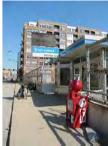
View of west stationhouse entry at Morgan Street
