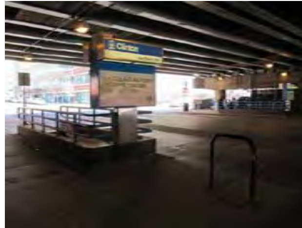
View of 1 of 4 station entries at Clinton Street
