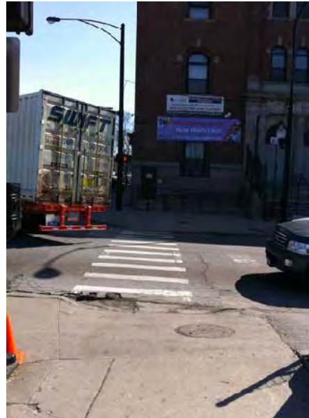
View of non-compliant curb ramp at Western Avenue and Congress intersection on approach to station. Note that the road within the crosswalk is also in need of repair
