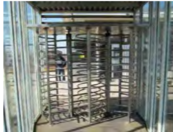
View of roto-gate exit at top of stair near center of platform
