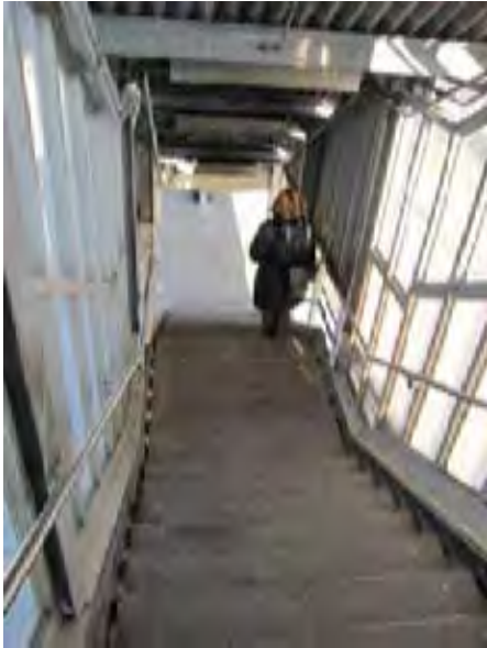
View of station entry stairs at Ogden Avenue stationhouse
