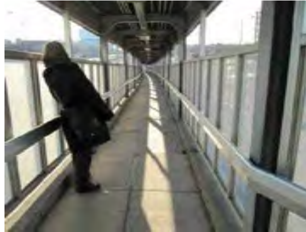
View of ramp at Racine Avenue entry
