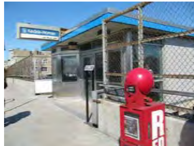
View of stationhouse entry at Homan Avenue
