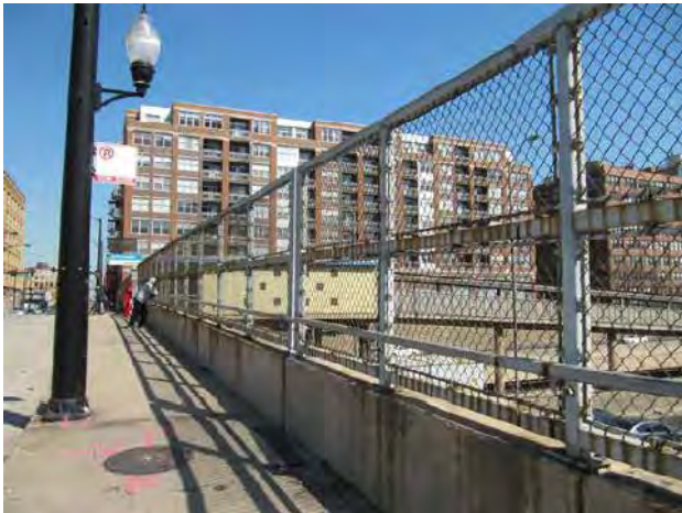
View of approach along Morgan Street to Morgan stationhouse.
