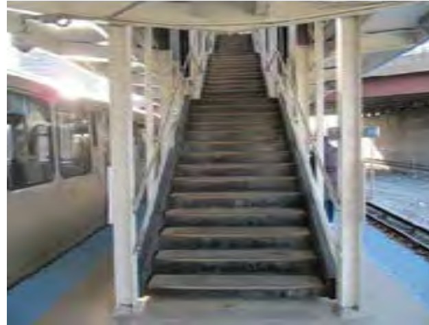
View of exit stair at center portion of platform
