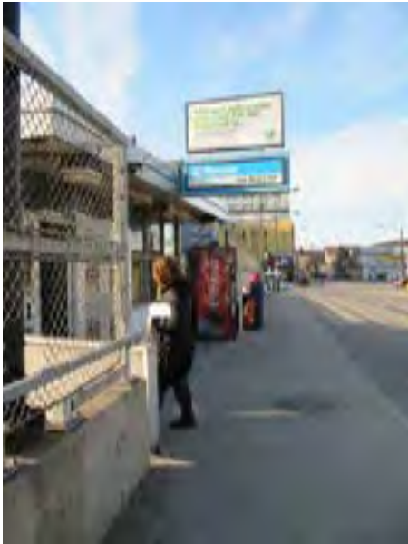
View of main station entry at Racine Avenue
