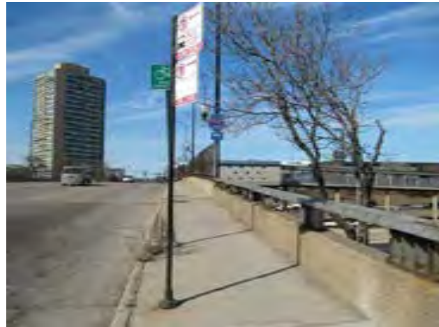
View of sidewalk along Damen Avenue on approach to Damen stationhouse.
