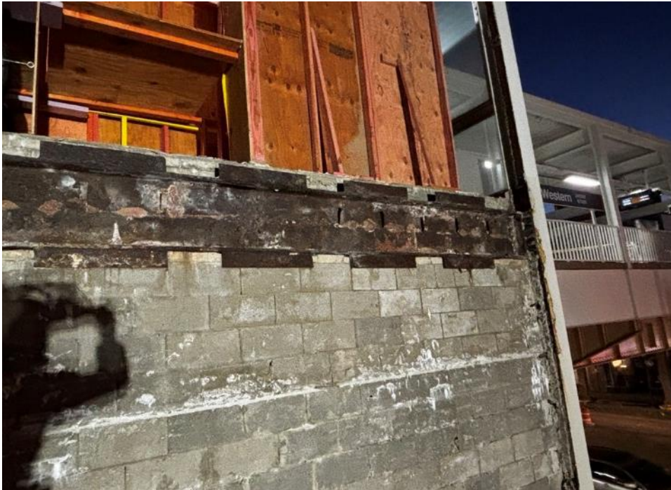
North Wall Structural Steel and CMU
