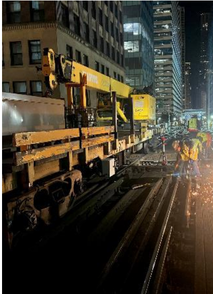
Cutting out the old quadrant castings at Tower 18.
