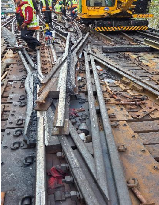
Removal of the frog and addition of a straight rail at LaSalle Crossover
