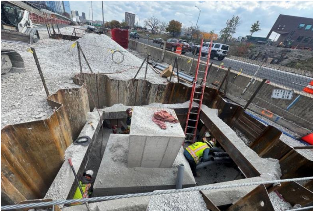
Loomis Electrical Sending Pit and Tie-in
