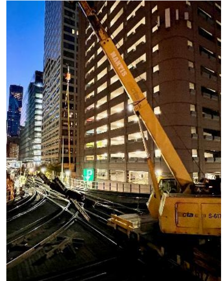
Cutting out the old quadrant castings at Tower 18.
