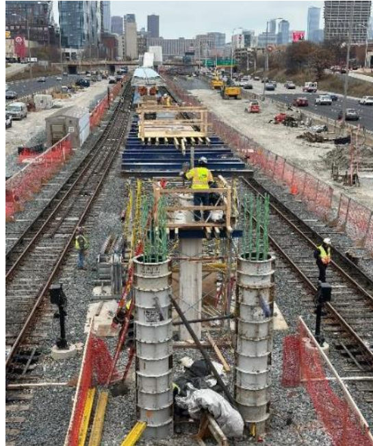
Loomis Stationhouse Columns Rebars and Forms
