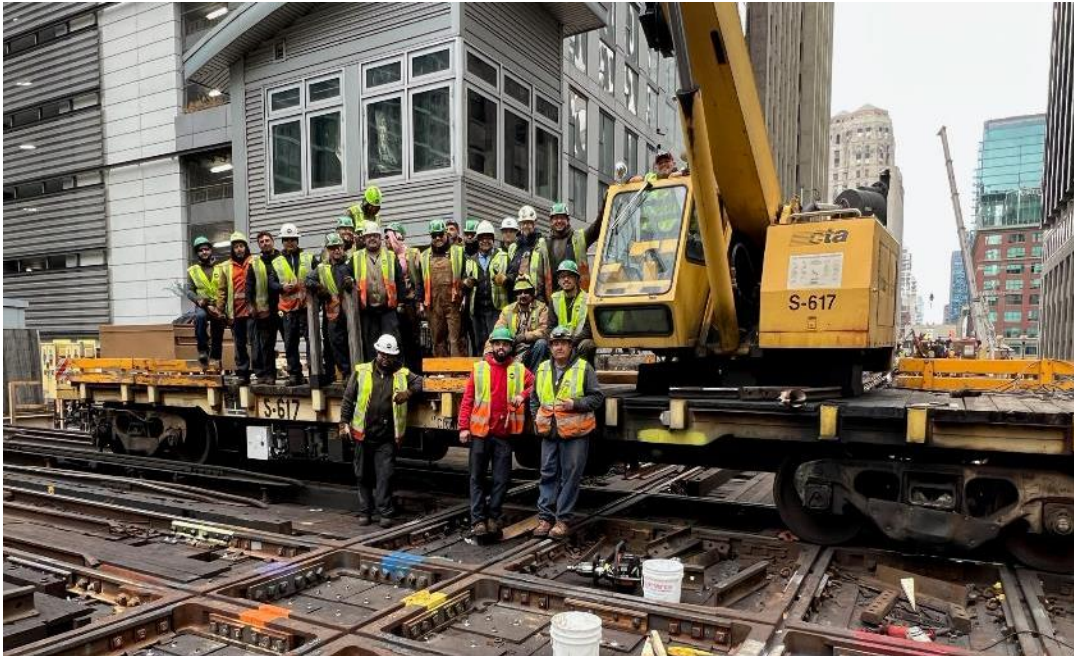
The Track casting crew at Tower 18, castings installed
