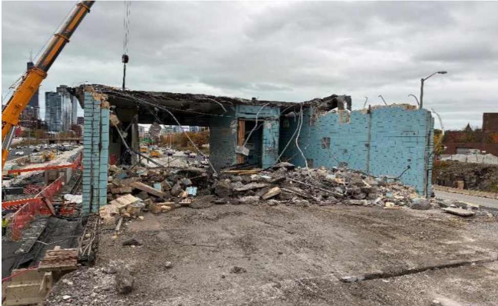
Loomis Stationhouse Demolition
