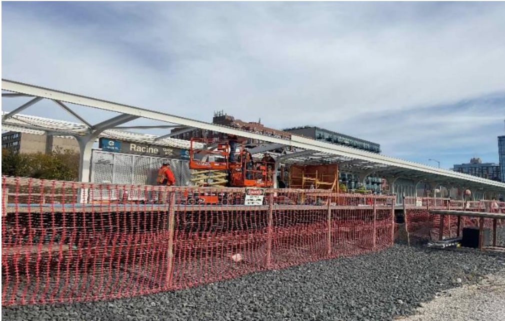
The Loomis End - Platform Purlins Installation
