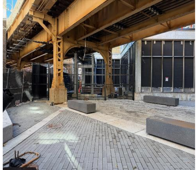
Fencing Installation at Damen
