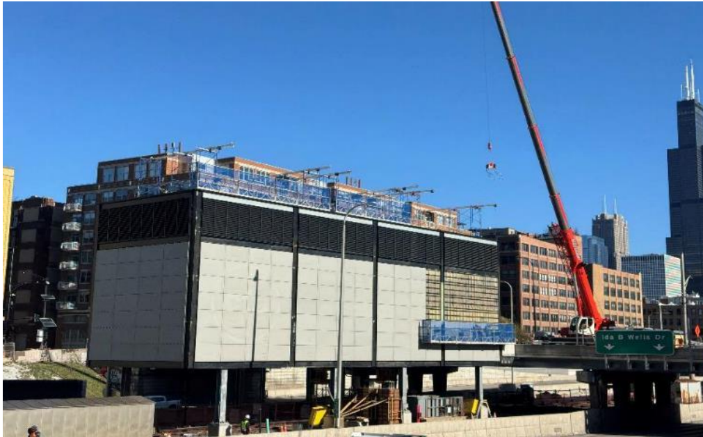
The HPCP at Morgan Substation South Wall
