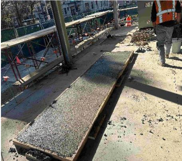
Communications/Electrical Room Housekeeping Pad and Underslab Utilities Installation
