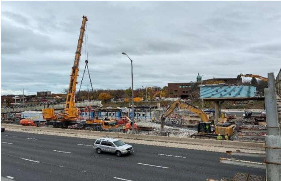
Loomis Ramp Demolition and Removal
