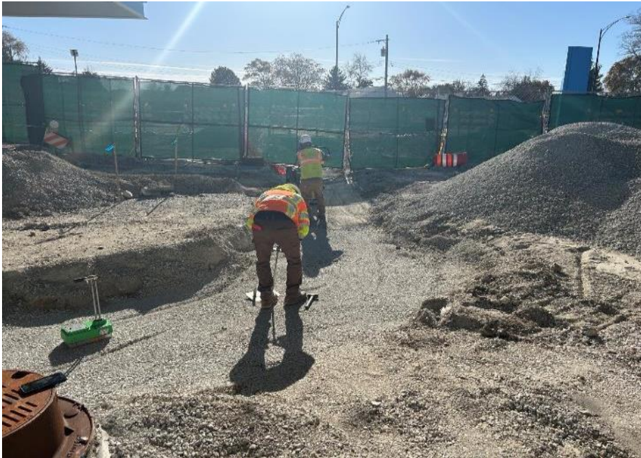
Performing Density Tests on Trench Backfill
