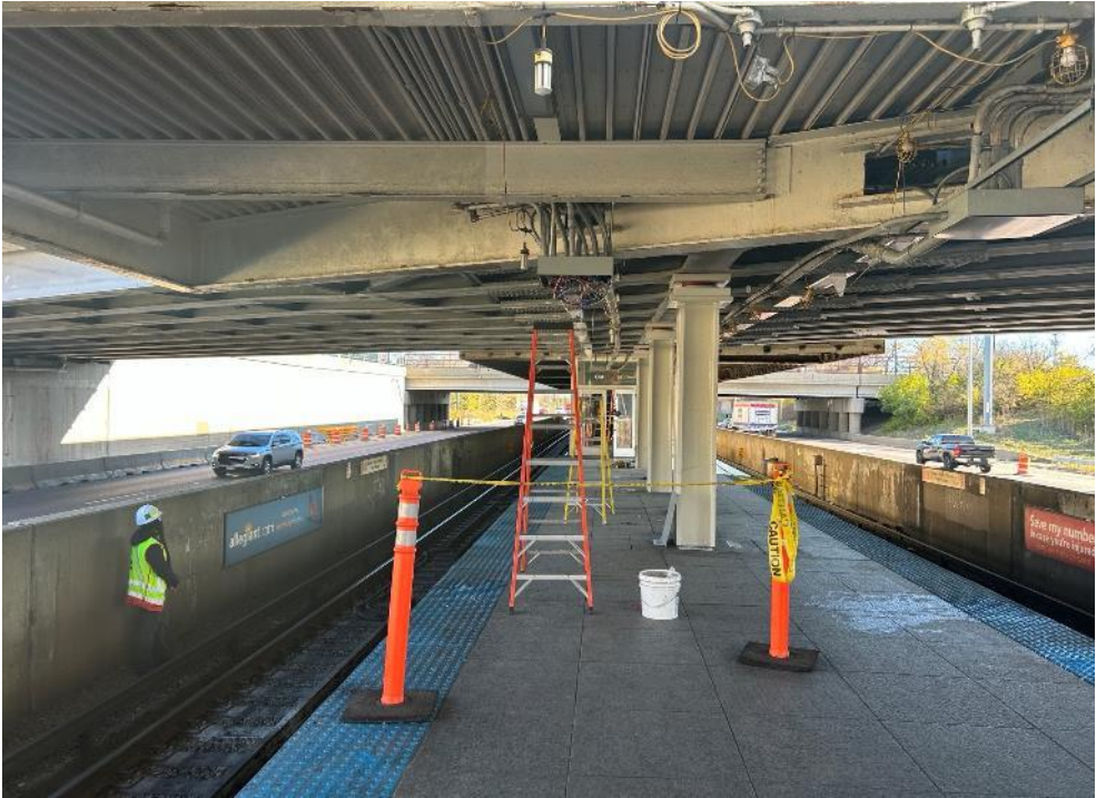
Pulling Wire Under Bus Bridge
