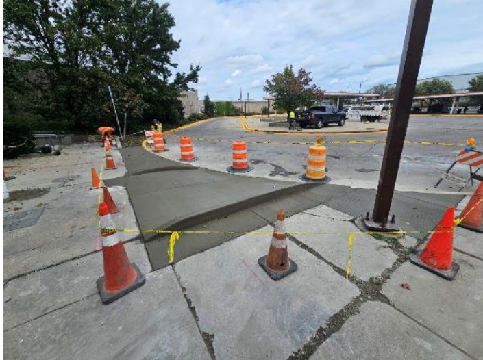
Kedzie Orange Line – Curb Repair & Ramp Installation
