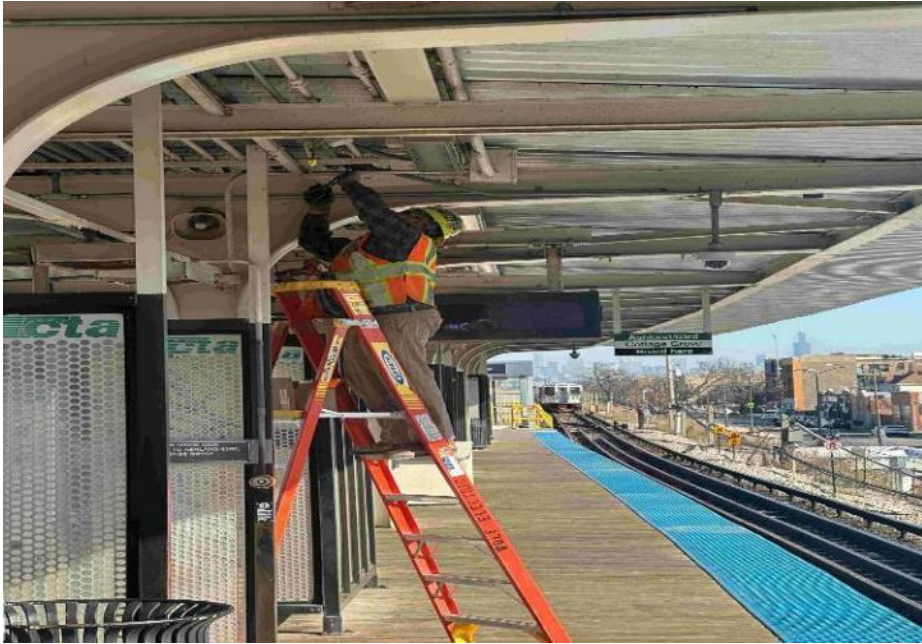
Continued Platform Level lighting installation
