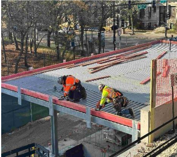
Communications/Electrical Room steel framing and roof deck installation
