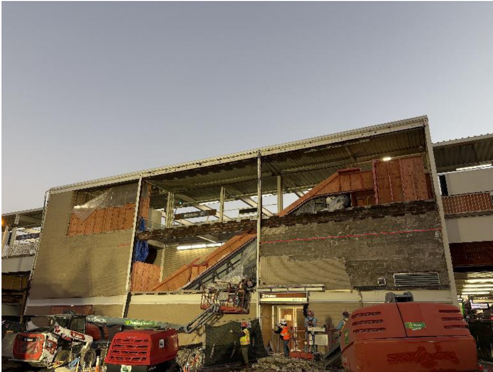
Demolition of North Wall Masonry
