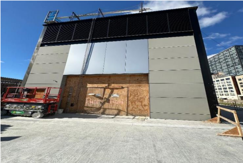
The HPCP at Morgan Substation Main Entrance
