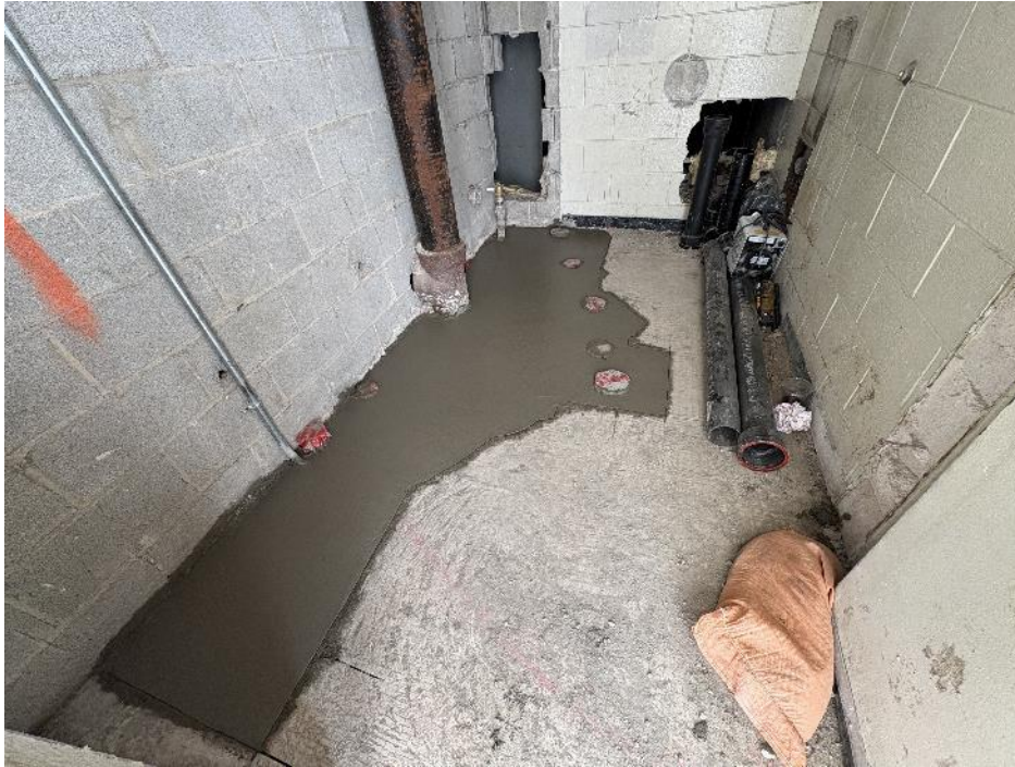
Pouring Floor for Bus Washroom
