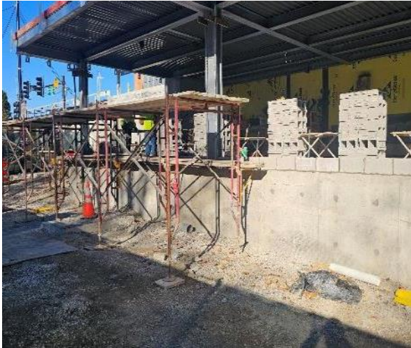
Communications/Electrical Room Masonry wall installation
