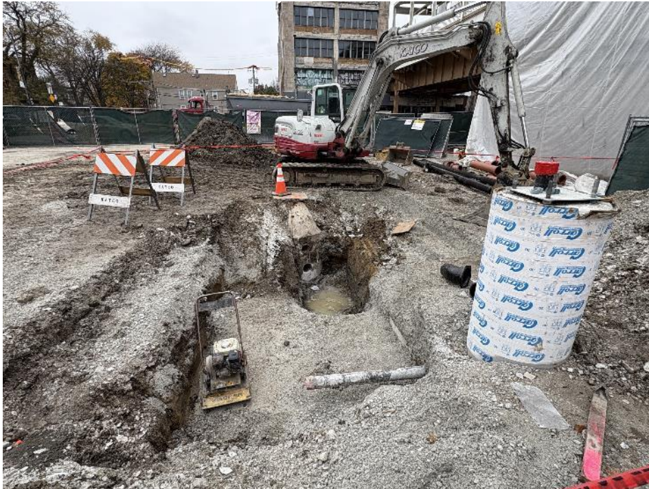
Excavation for New Sewer Pipe
