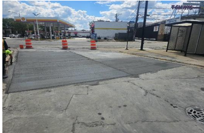
36 th & Kedzie BTA – Concrete Repair
