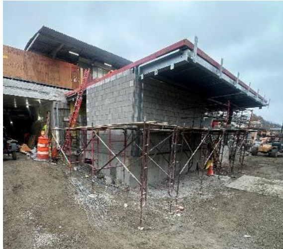
Communications/Electrical Room Masonry wall installation
