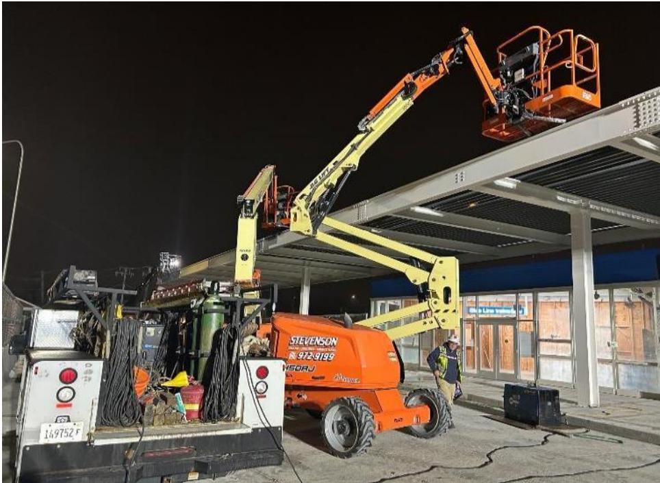
Installing Corrugated Decking at Canopy
