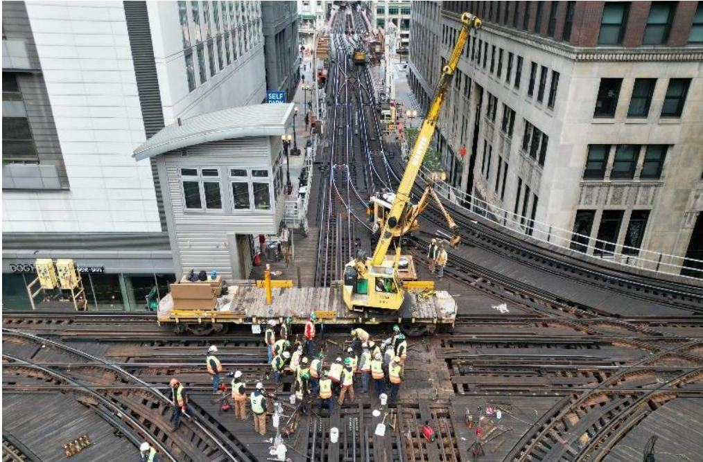
Complete removal of the old castings at Tower 18.
