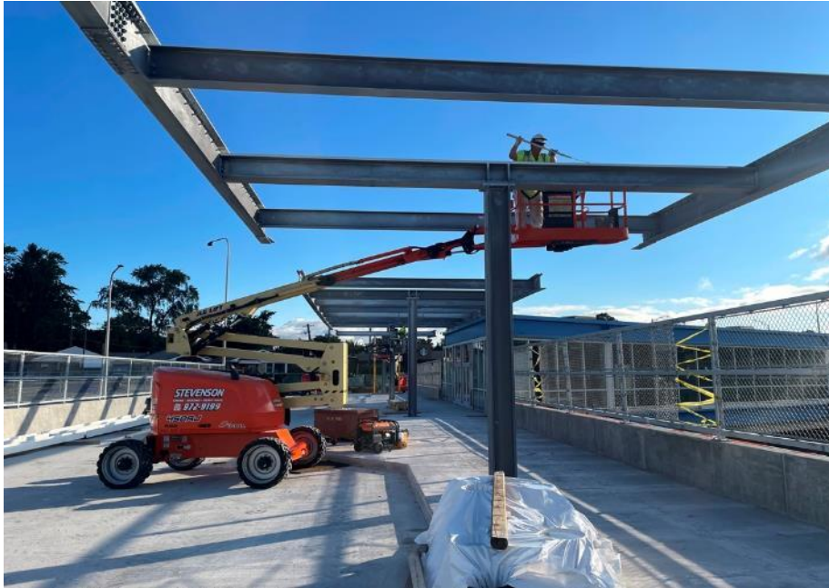
Painting Bridge Canopy Steel
