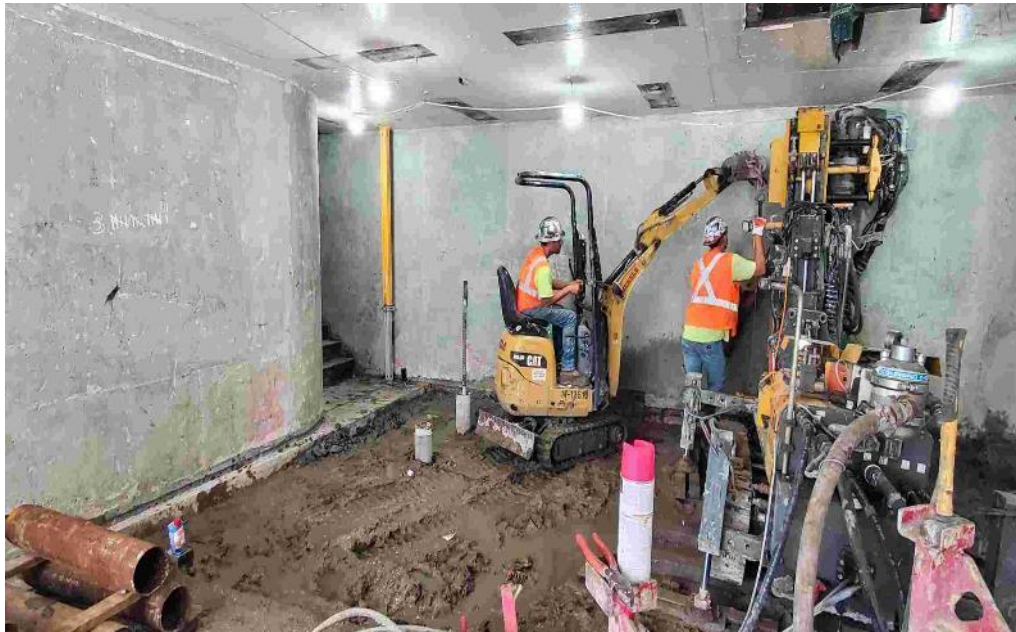
Micropile Drilling at Austin Stationhouse Elevator Location
