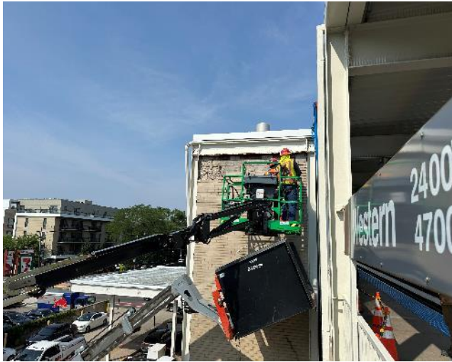
Masonry Demolition At Track Level
