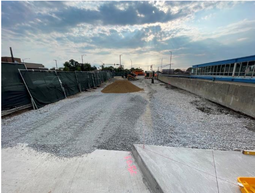
Grading for the North Approach Slab
