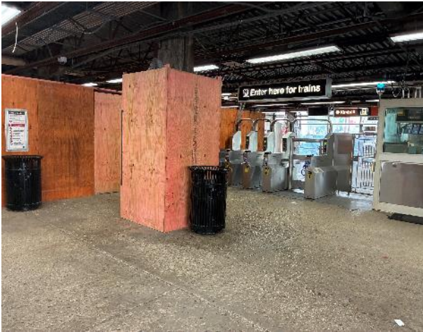
Columns Enclosed for Repair Work
