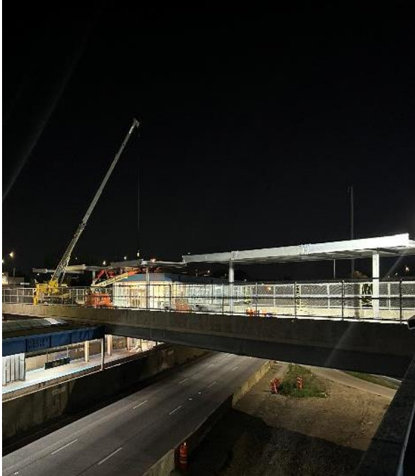
Installing Bridge Canopy Steel
