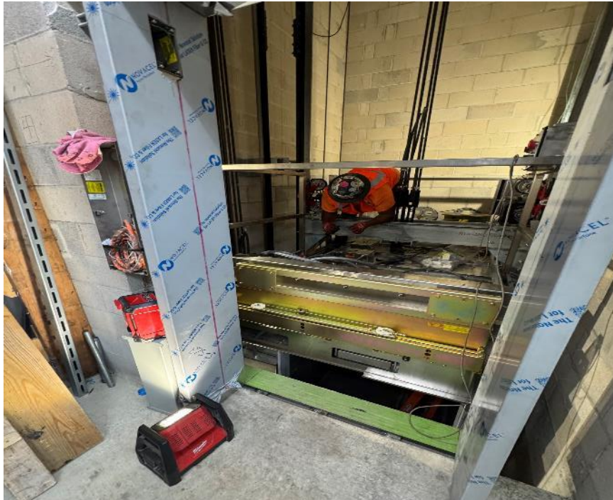
Racine Elevator Installation
