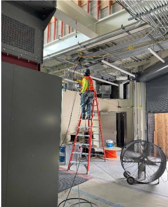
Barry Communication Cable Installation
