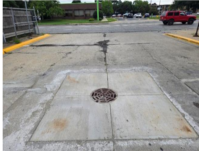
Pulaski/104 th - BTA Sunken Manhole Repair
