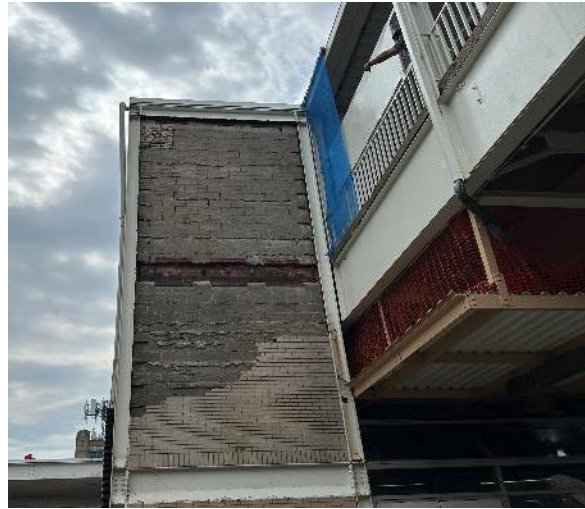
Masonry Demolition At Track Level
