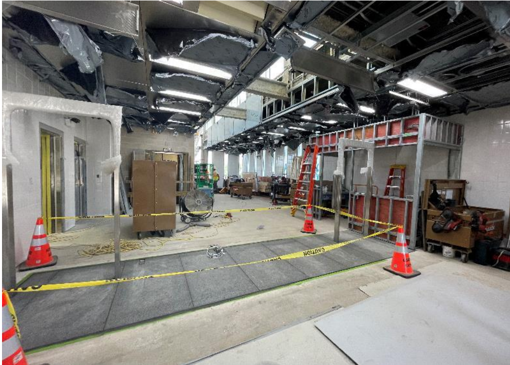
Racine Stationhouse Fare Array Granite Flooring
