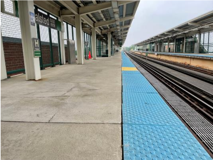
Halsted/63 rd Green Line – SB Platform Tactile Replacement
