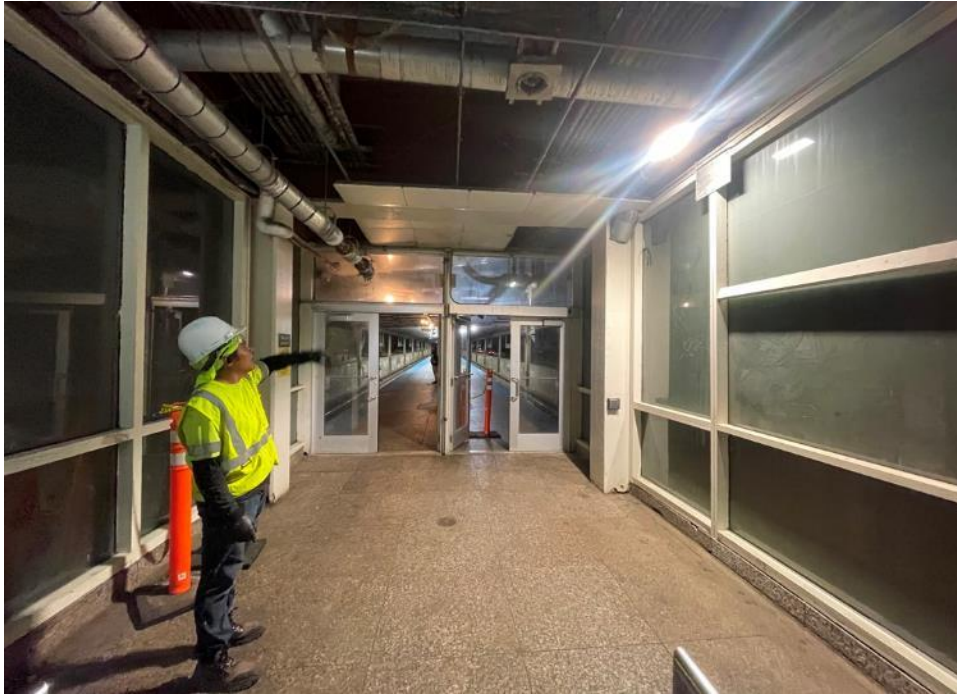
Removal of Station Ceiling
