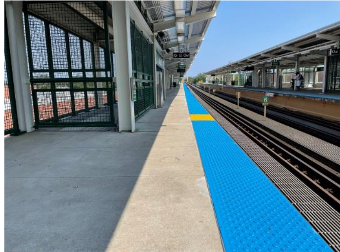
Halsted/63 rd Green Line – SB Platform Tactile Replacement
