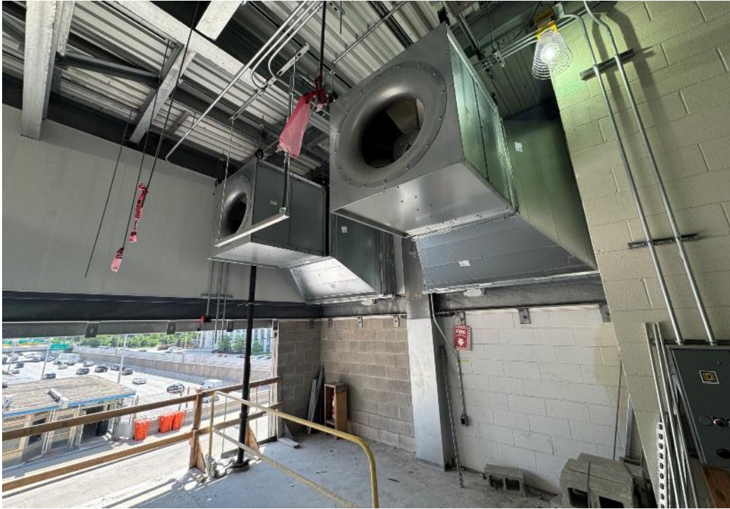
Morgan Substation Exhaust Fans Installation
