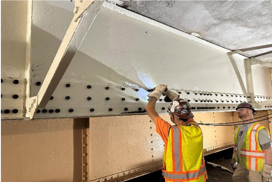
Ironworkers Torquing Bolts Below Platform
