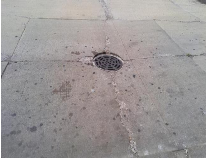
Pulaski/104 th - BTA Sunken Manhole Repair
