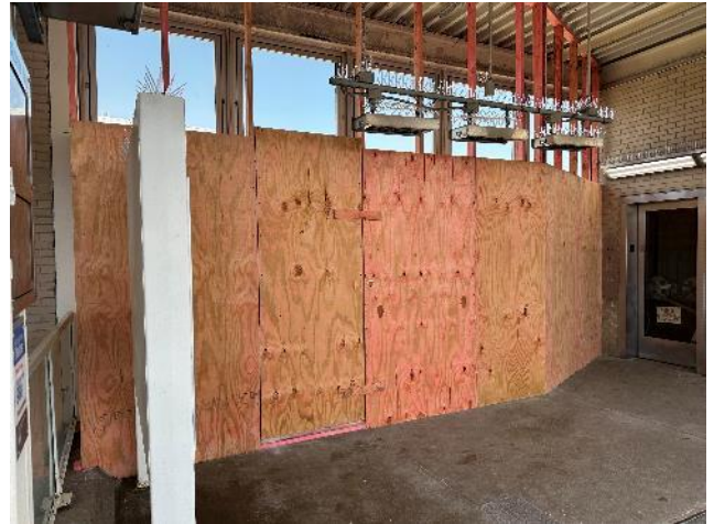
Barricade for Masonry Demolition
