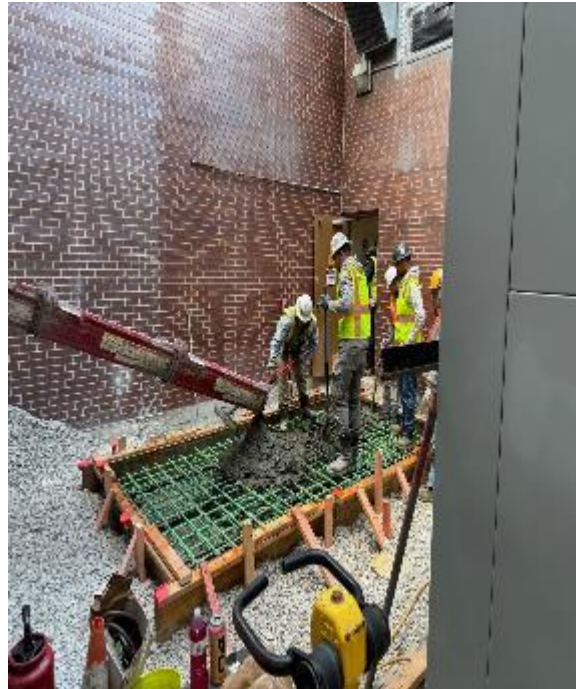
Installation of Switchgear Leveling Channels and Transformer Pad at Haymarket
