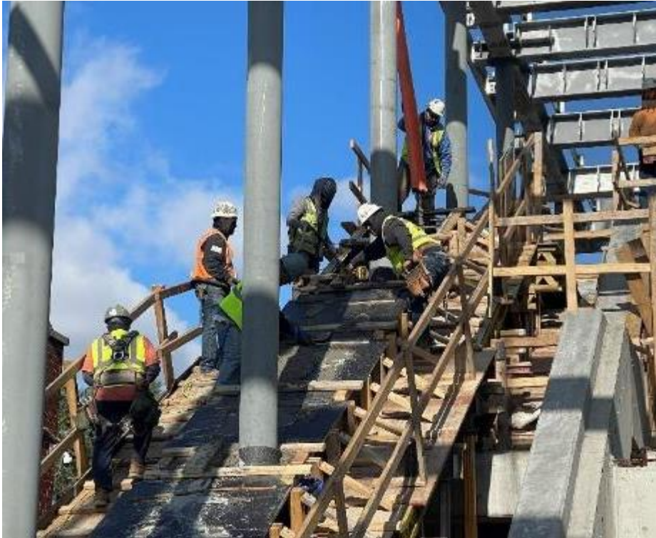
Pouring Concrete at West Exterior Wall
