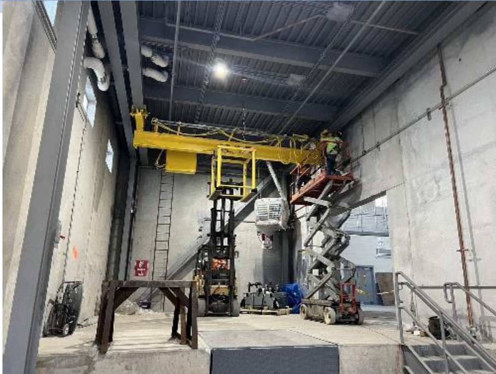
Loading Dock – Crane Installation
