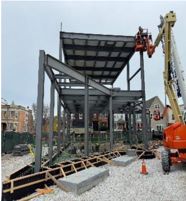
Structural Steel Erection and Forming Stem Wall at Barry
