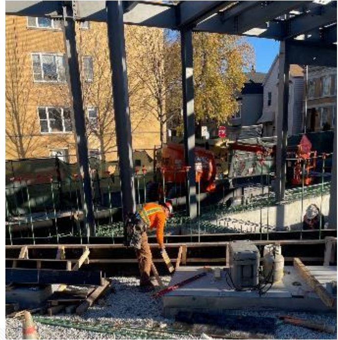
Structural Steel Erection and Forming Stem Wall at Barry
