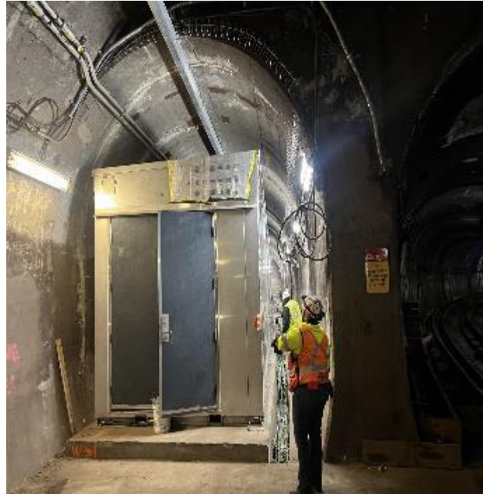
Canal Tie-House Installation
