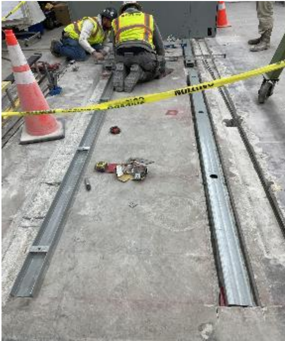
Installation of Switchgear Leveling Channels and Transformer Pad at Haymarket
