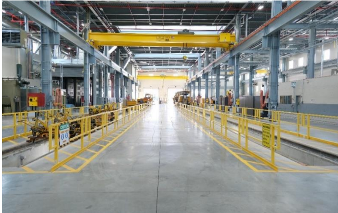
Interior view of the new 63rd Non-Revenue Rail Maintenance Vehicle Shop.
