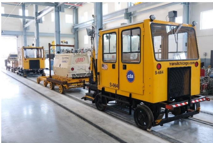
The 63rd Non-Revenue Maintenance Vehicle Shop is a new, state-of-the-art facility designed to accommodate the maintenance of over 125 pieces of power and way equipment and other rail-mounted non-revenue vehicles.
