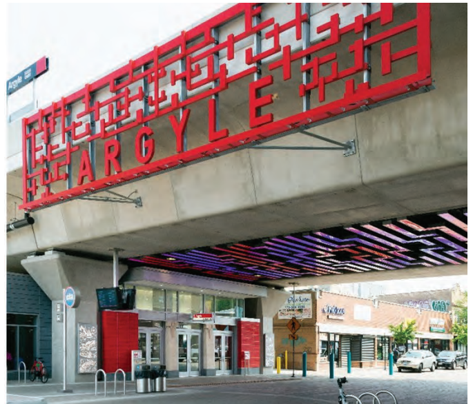
Argyle was one of four Red Line stations that re-opened this July after being completely rebuilt and made fully accessible as part of RPM Phase One work.
