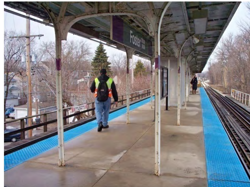
Foster - despite restrictive beams, path compliant
