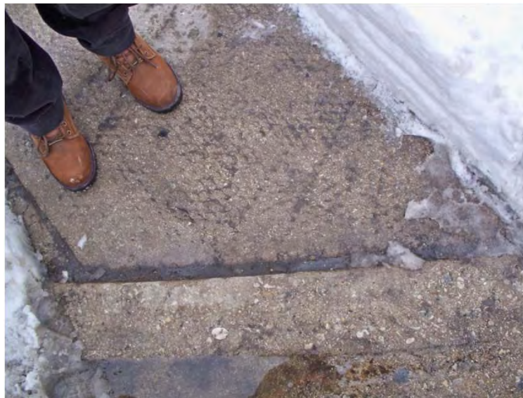
Curb ramp at Austin
