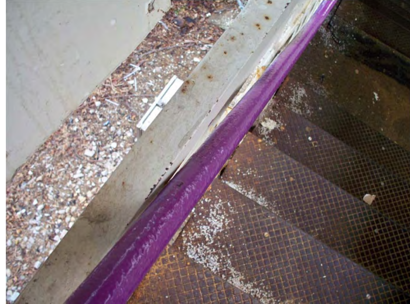
Dempster Station – Space between handrail and wall less than 1.5”
