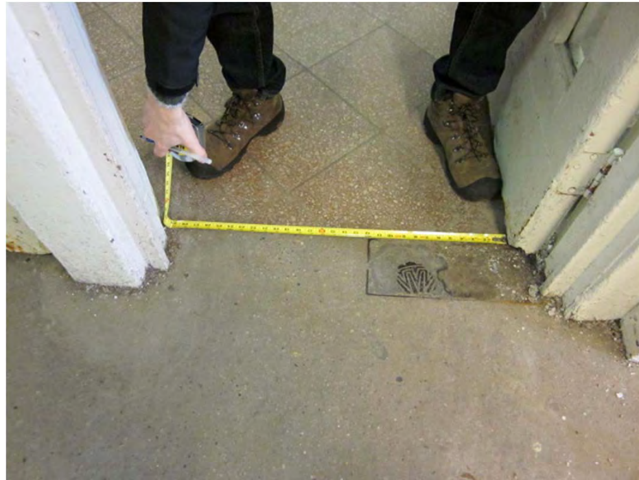
Entrance door at Morse
