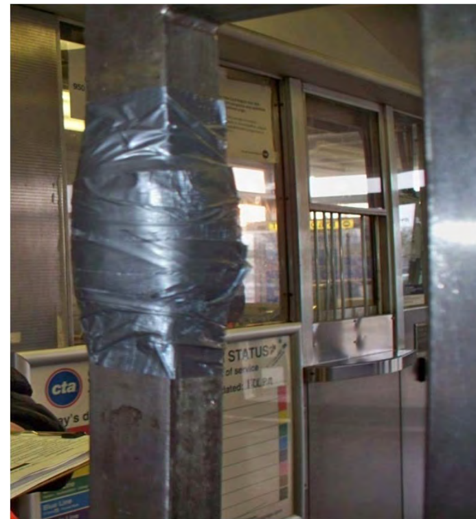
Oak Park accessible gate taped to close
