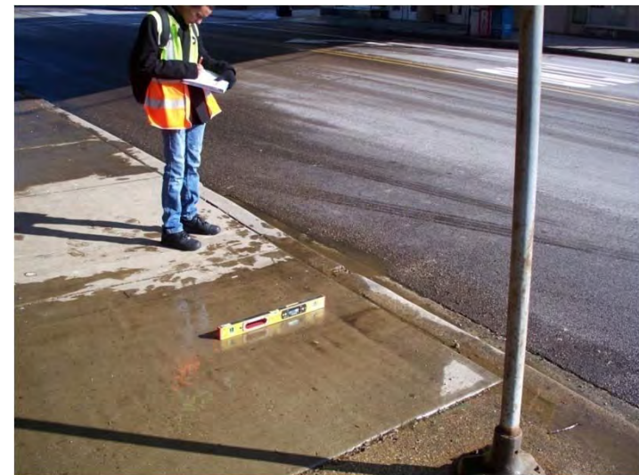
Central Station - Central Ave. across from station - slope of boarding area
