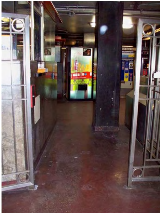
Monroe/State north mezzanine support beam prevents full access to gate
