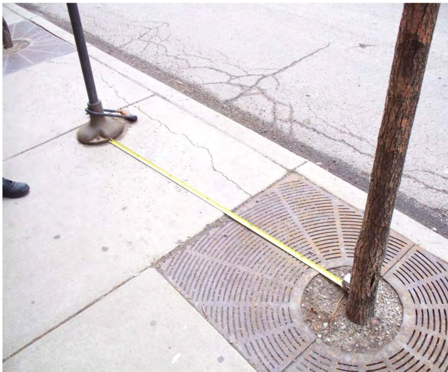
Main Station - Northeast corner of Chicago and Main - bus boarding area
