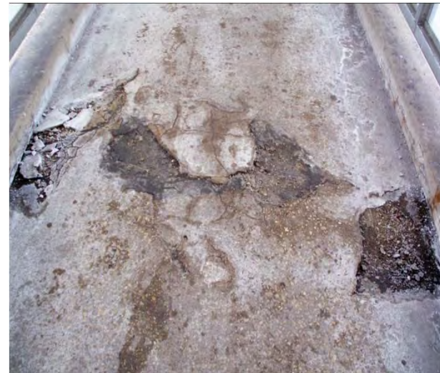
Cicero ramp - gaps greater than 1/2"
