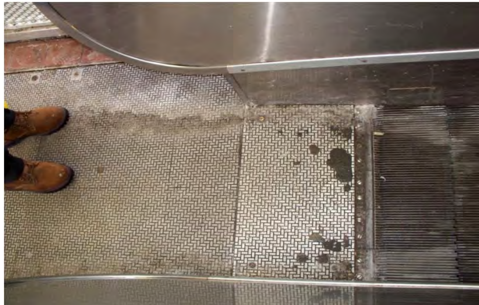
Escalator at Austin (26" clearance).
