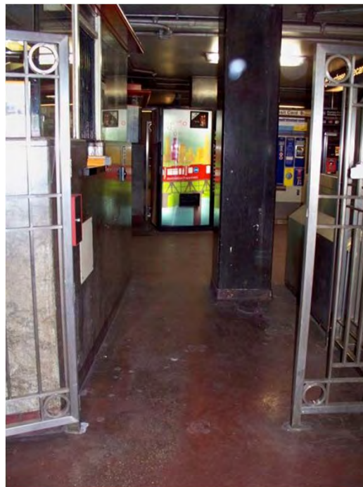
Monroe/State North mezzanine support beam prevents wheelchair access to gate
