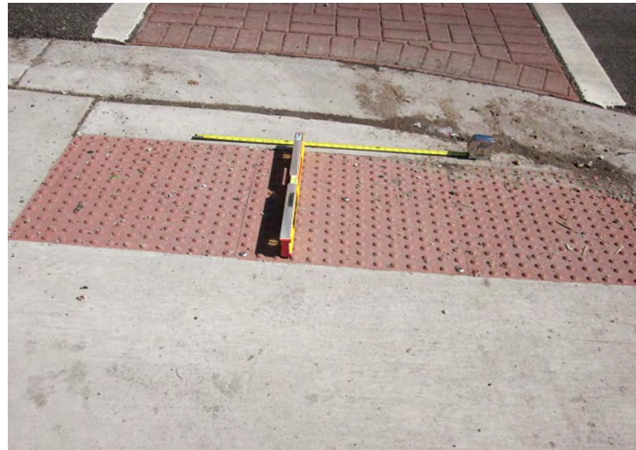
Compliant curb ramp at Morse
