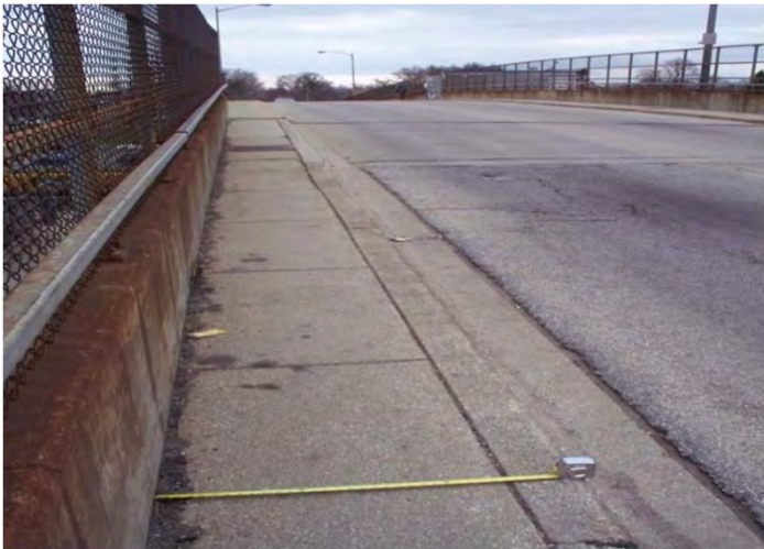
Harlem Avenue exterior accessible route
