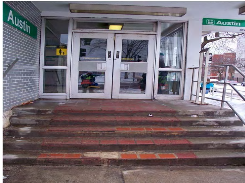
Station entrance at Austin
