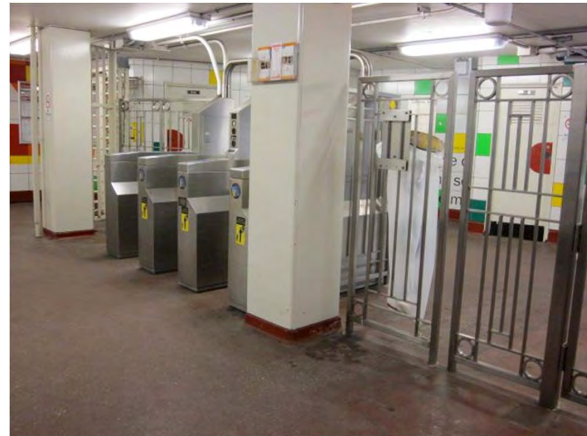
Harrison/State Gate at main entrance available to people with disabilities
