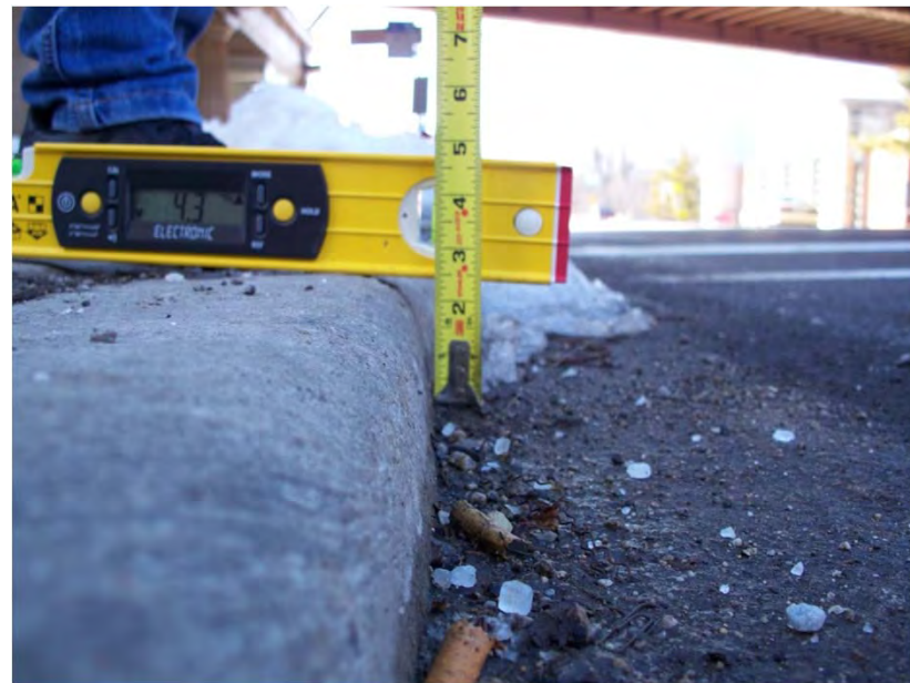
Central Station - abrupt transition
