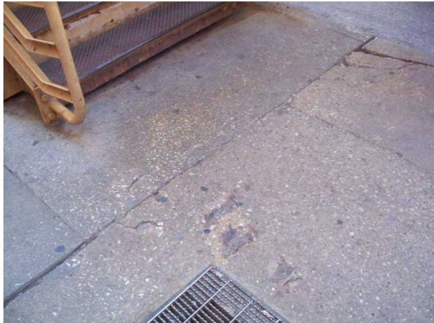
Gaps at Randolph/Wabash
