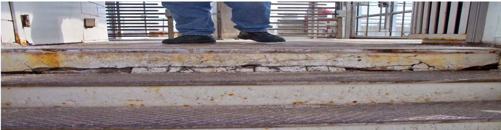
Oak Park secondary entrance (East Avenue) top step crumbling
