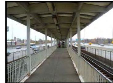
5 Existing Walkway at Unattended North Auxiliary Entrance / Exit
