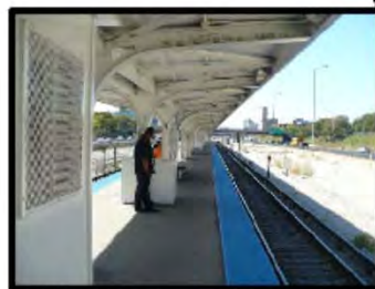
Existing Platform Looking West
