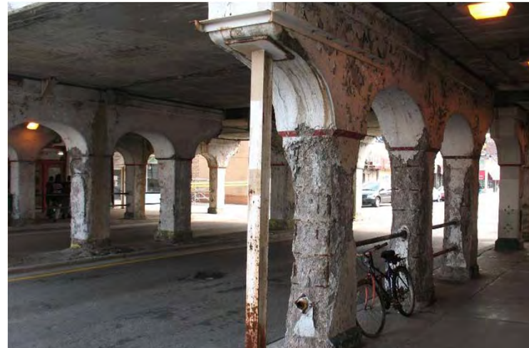
Poor structure condition requires temporary measures
