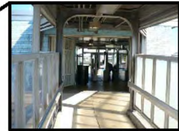
Existing Station House at Racine
