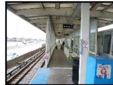
4 Existing Stairs and Escalator
