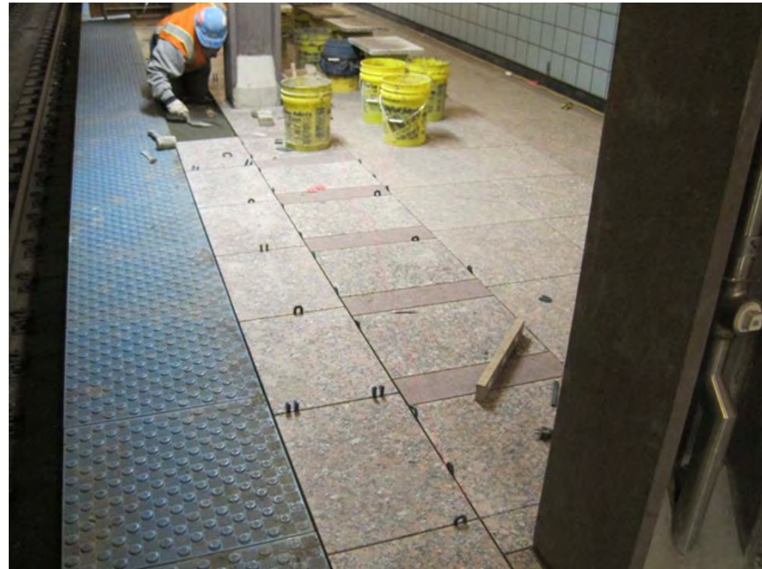
Grand Subway Station
