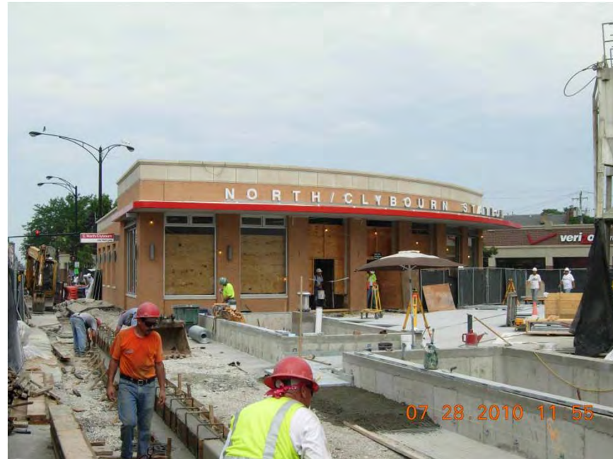
North / Clybourn Station
