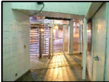
2 Existing Unattended Pulaski Auxiliary Station House
