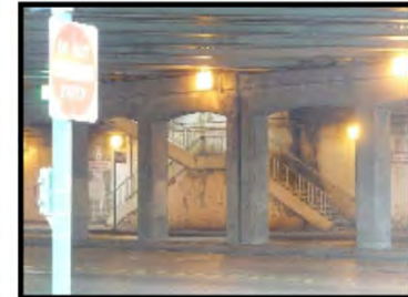
4 Existing Unattended South Auxiliary Entrance / Exit
