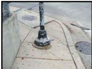
6 Existing Non-Compliant Sidewalk Ramp
