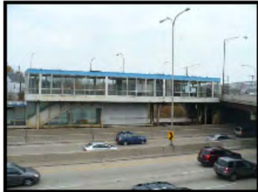
5 Existing Station House
