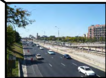
Existing Ramps and Platform
