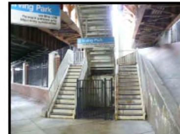
6 Existing Stairs at Unattended North Auxiliary Entrance / Exit
