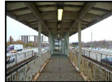
5 Existing Unattended South Stairs & Fare Control
