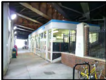
1 Existing Station House
