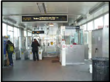
2 Existing Station House Fare Array
