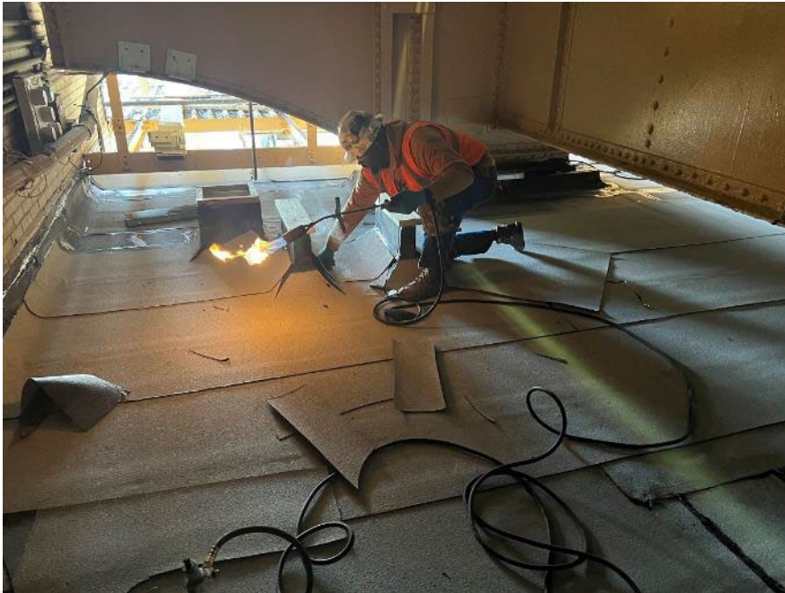
Station House – Install Roofing around Equipment Curbs
