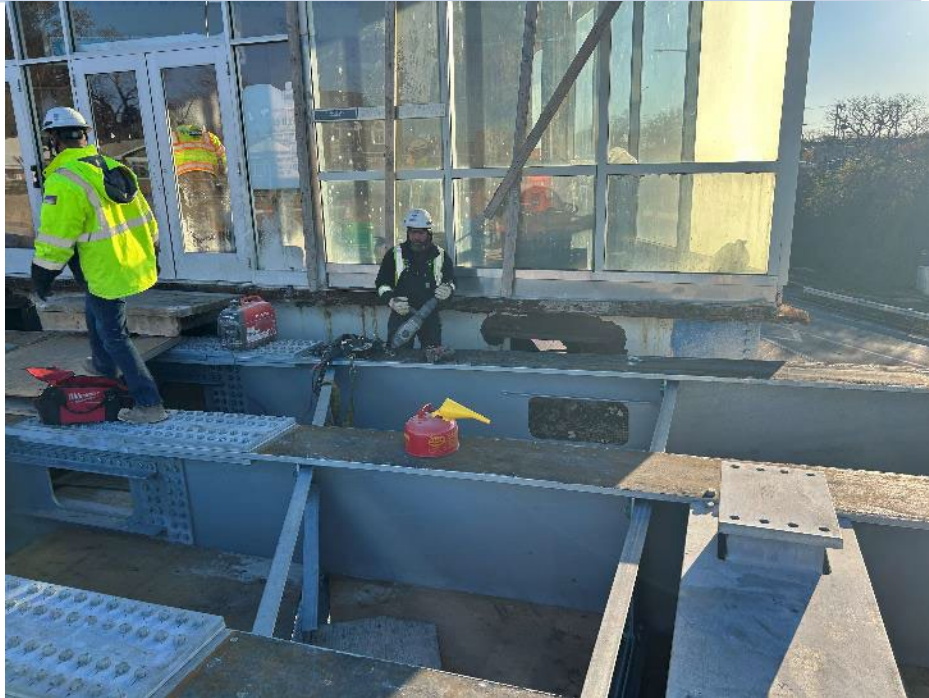
Preparing Existing Station House Beam for Repair/Paint
