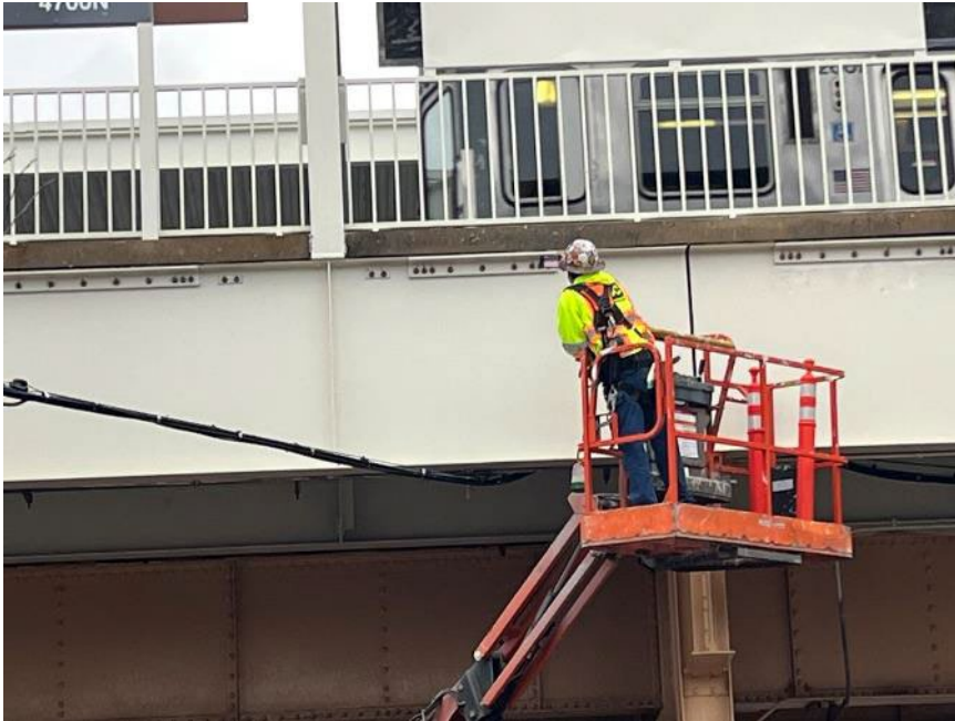
Inspecting Bolts for New Angles at Platform Level
