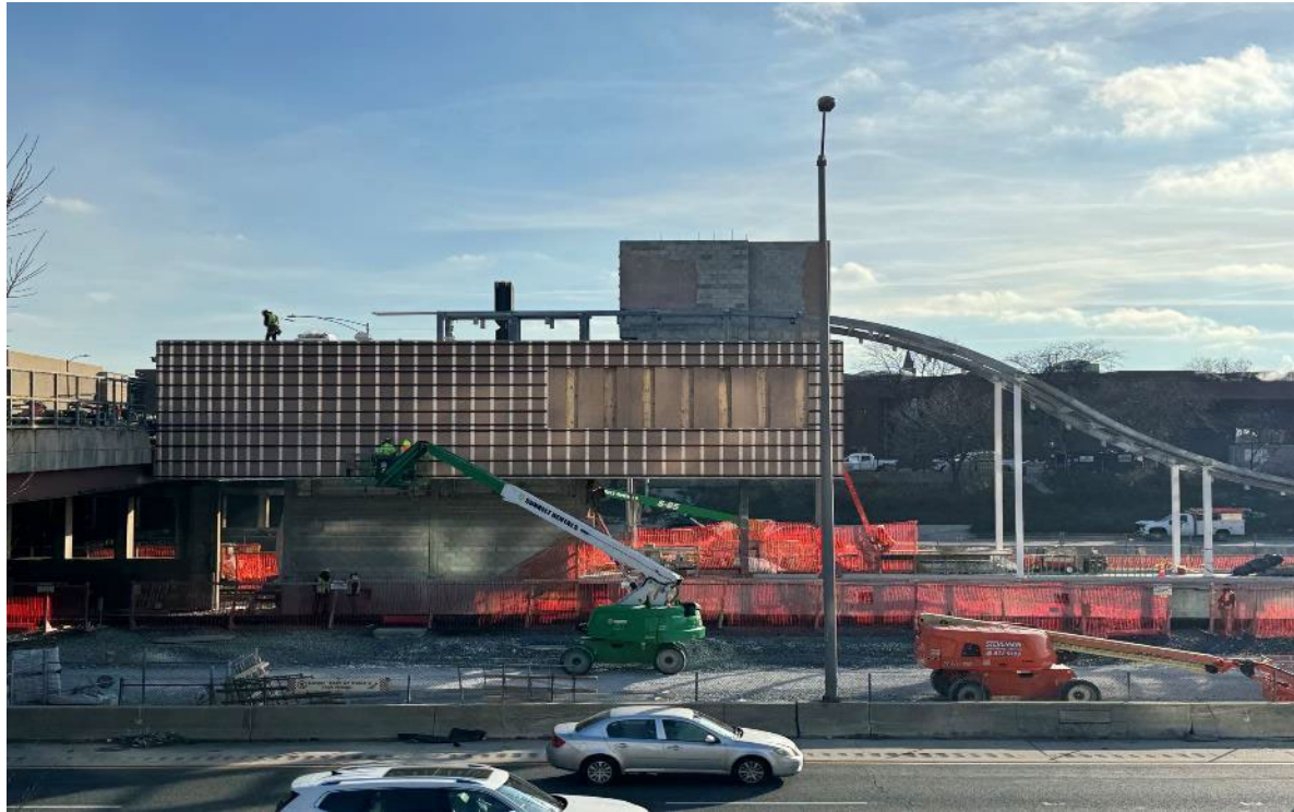
Racine Stationhouse Looking South
