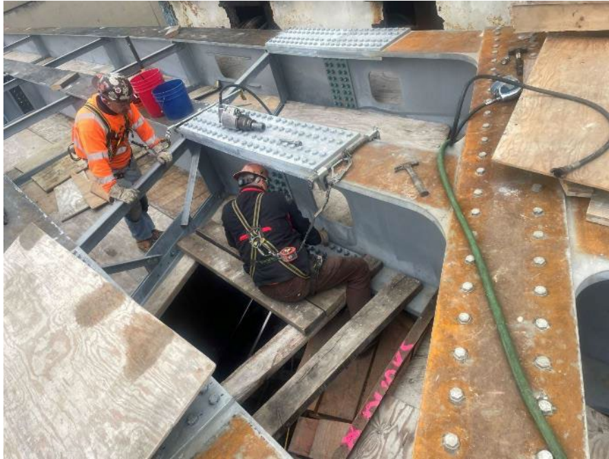
Ironworkers Torquing Bolts at Splice Plate
