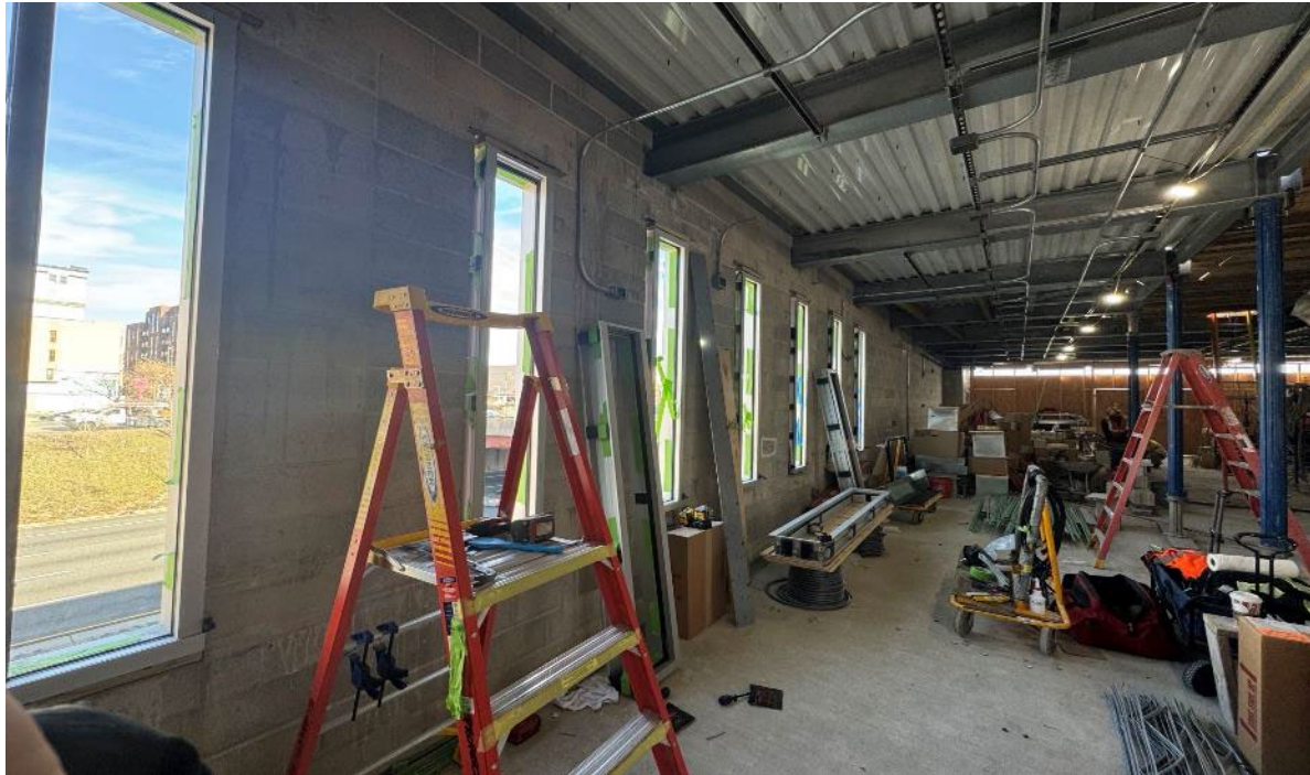
Racine Stationhouse Windows
