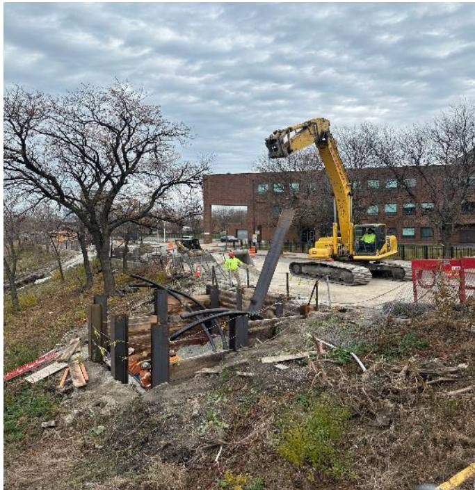
Removing ERS Whalers from Sanitary & Electrical Pits
