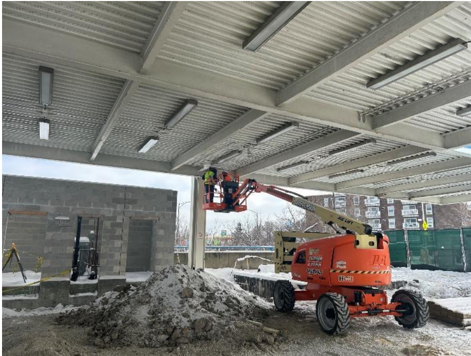
Electricians Installing Canopy Conduit
