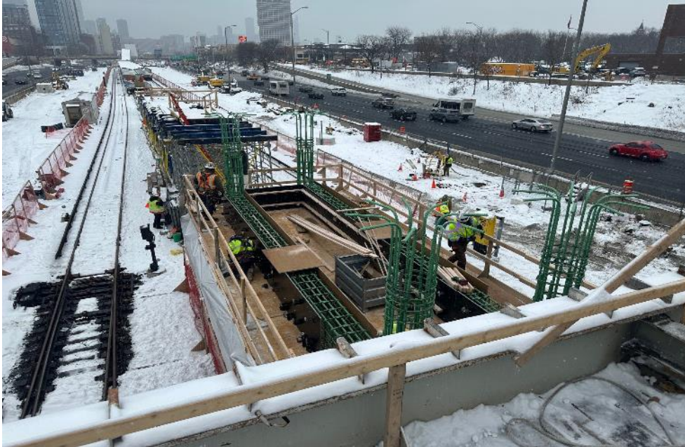
Loomis Stationhouse Beams Rebars & Forms
