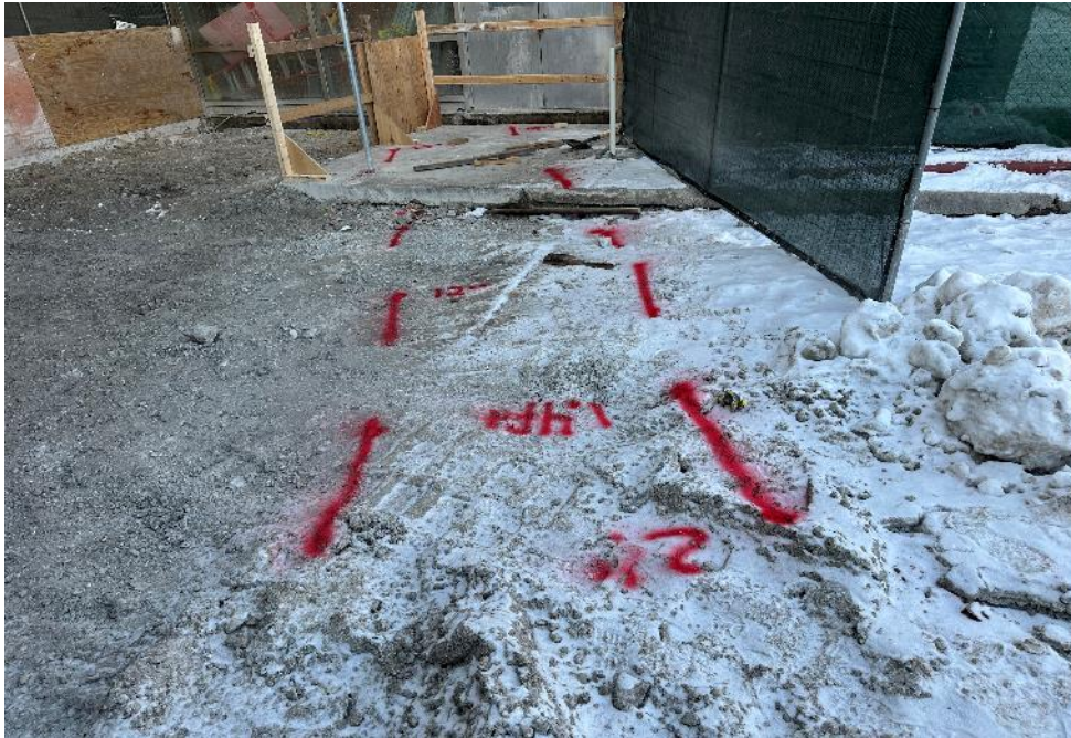
Locating Power for New Duct Bank
