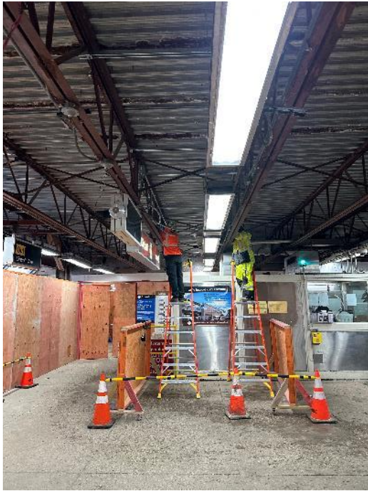
Running Conduit from New Electric Room
