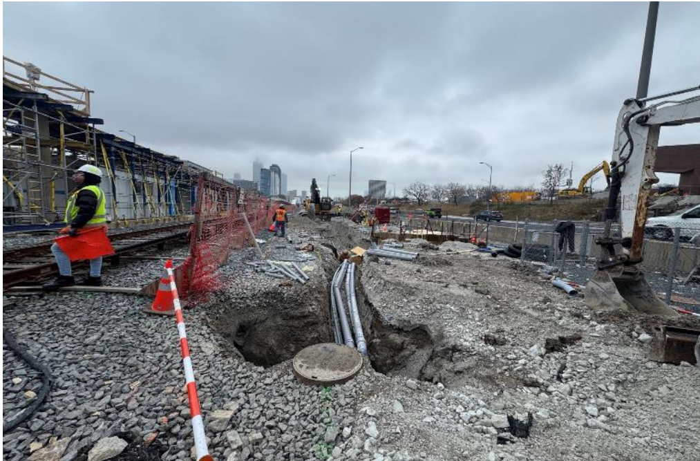
The Loomis End – Directional Drill Electrical Tie-in
