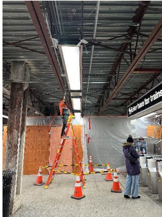
Running Conduit from New Electric Room
