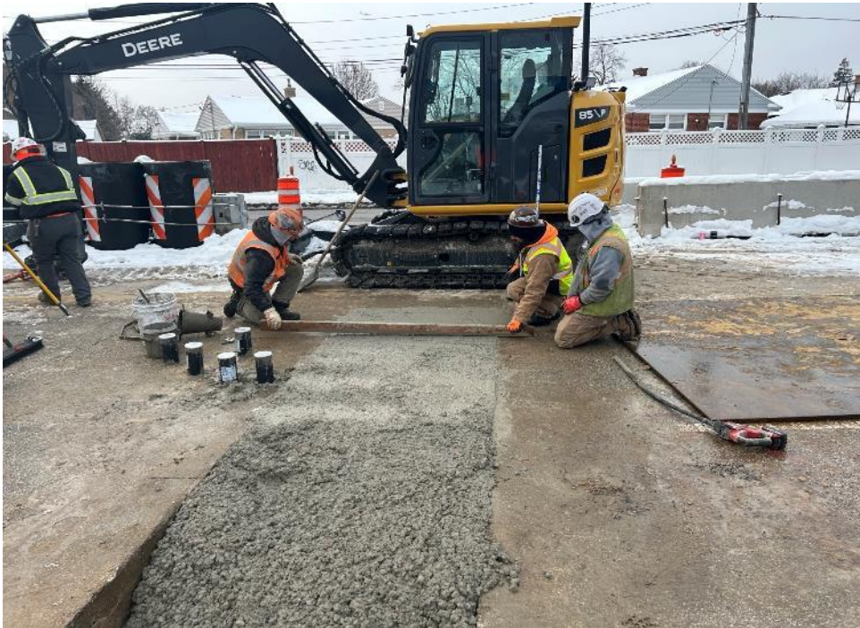
Patching Concrete Pavement at Higgins
