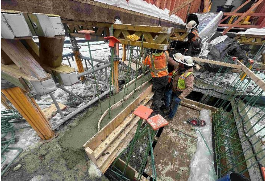
Retaining Wall Support Beam Installation at Elevator Shaft
