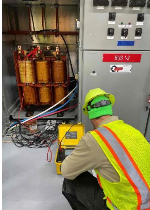
Barry Aux Transformer Testing
