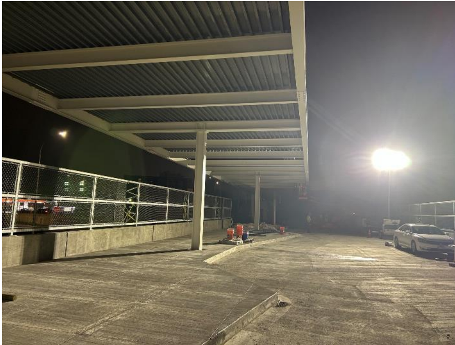
Completed Decking at New Bus Canopy
