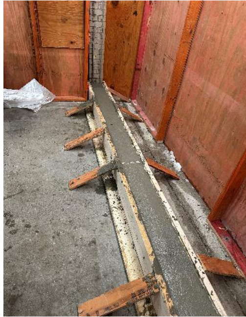
Forming and Pouring Station Storefront Curb
