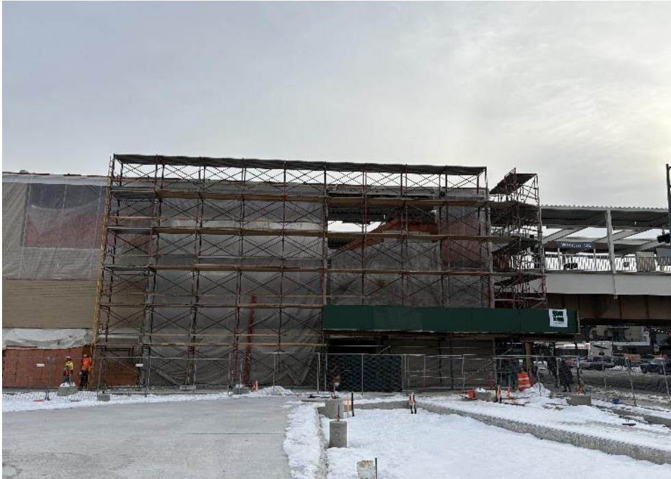
North Wall - Erection of Masonry Scaffold
