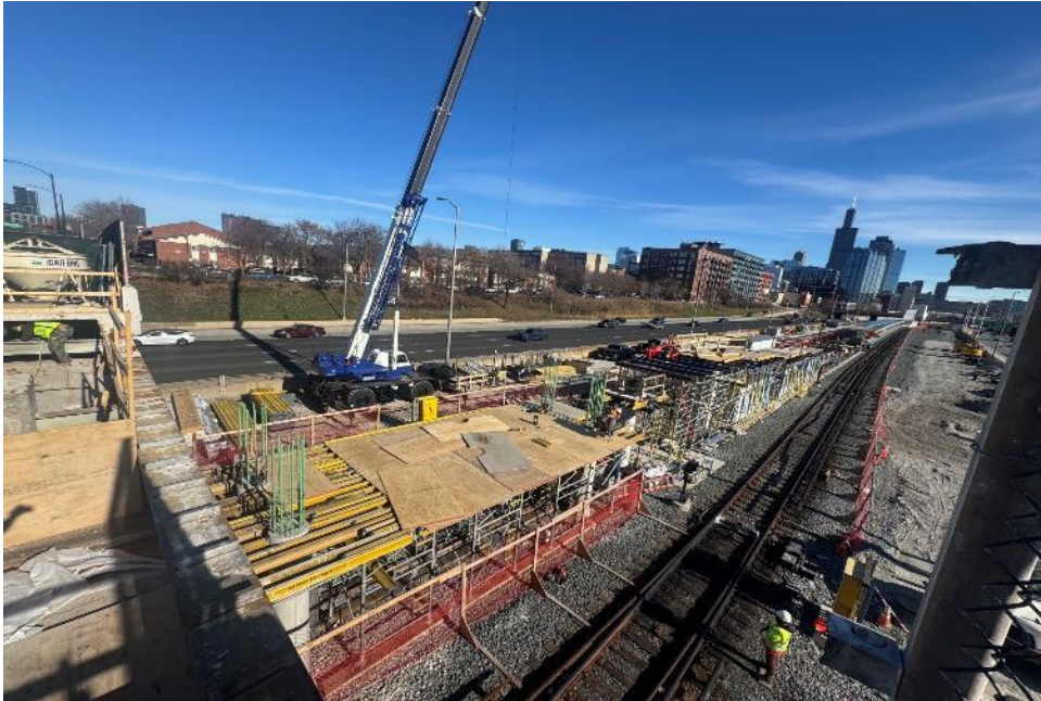
Loomis Stationhouse Deck Installation
