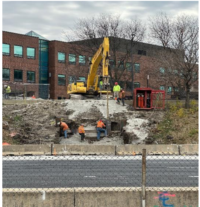
Removing ERS Whalers from Sanitary & Electrical Pits
