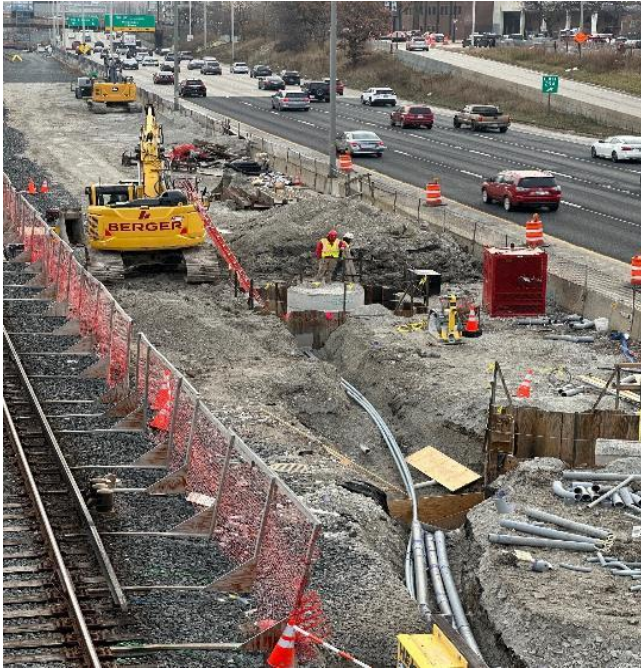
The Loomis End – Electrical Ductbank Work
