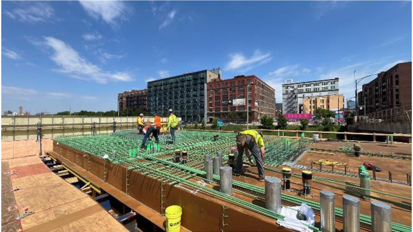
Racine Stationhouse Rebar Detailing on Deck and around Elevator Shaft
