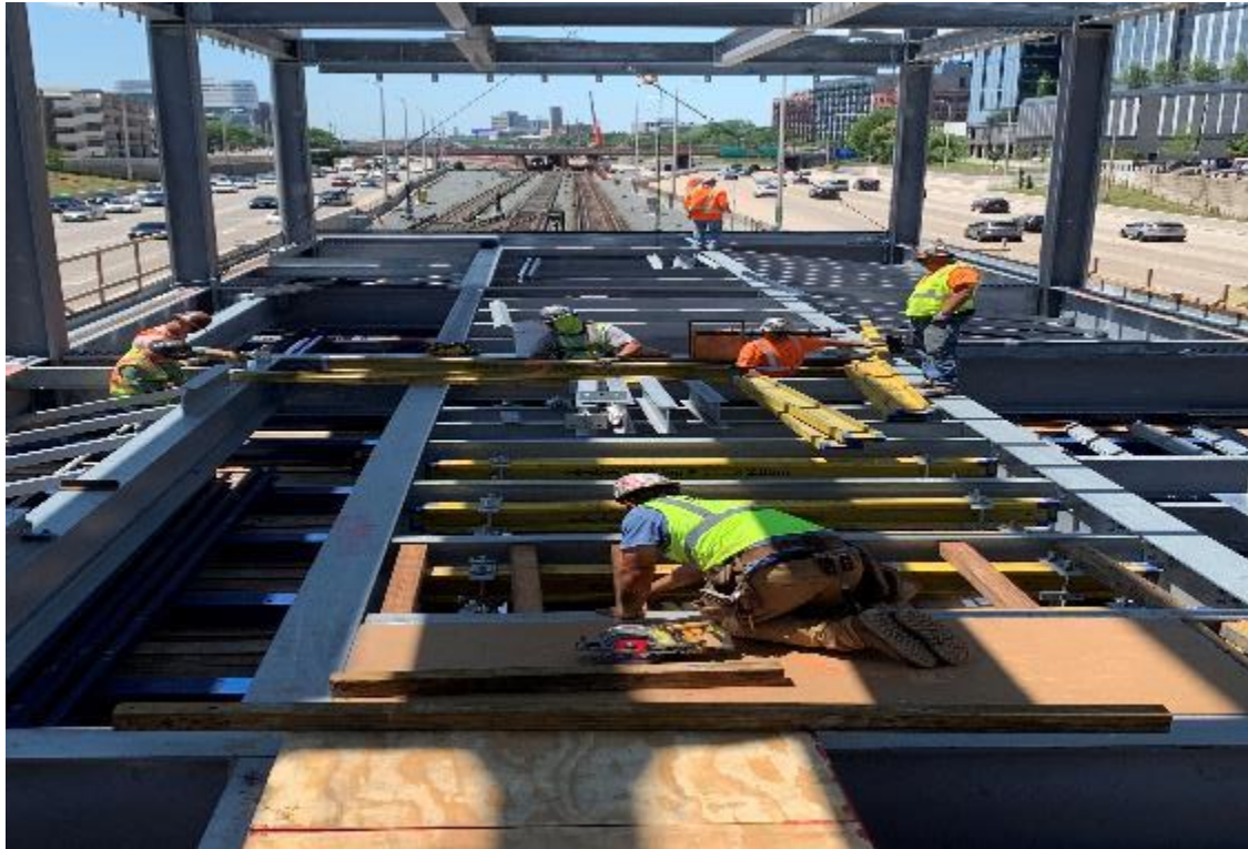
Morgan Substation Bridge Level Structural Steel Detailing and Form Work
