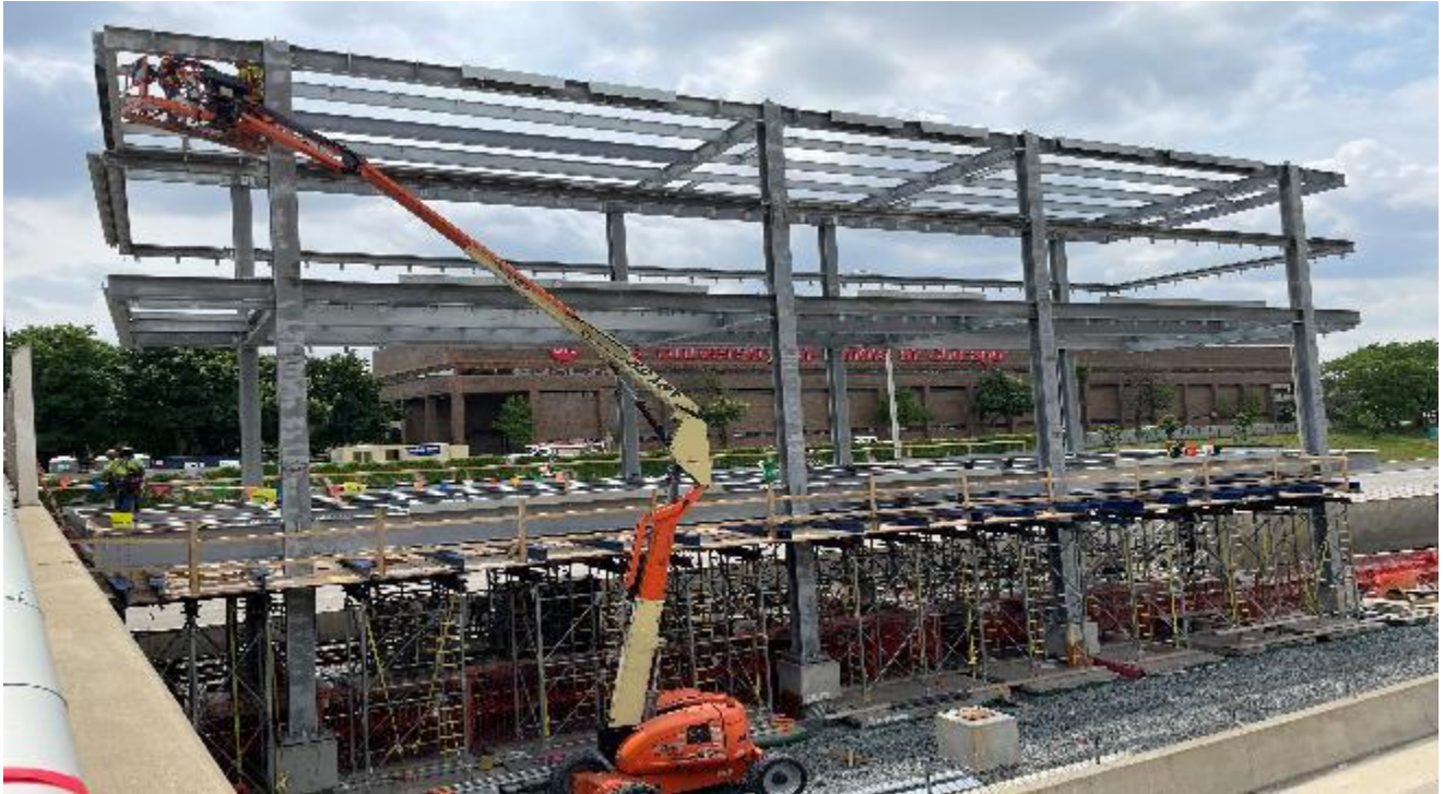
Morgan Substation 2 nd Level Structural Steel Detailing
