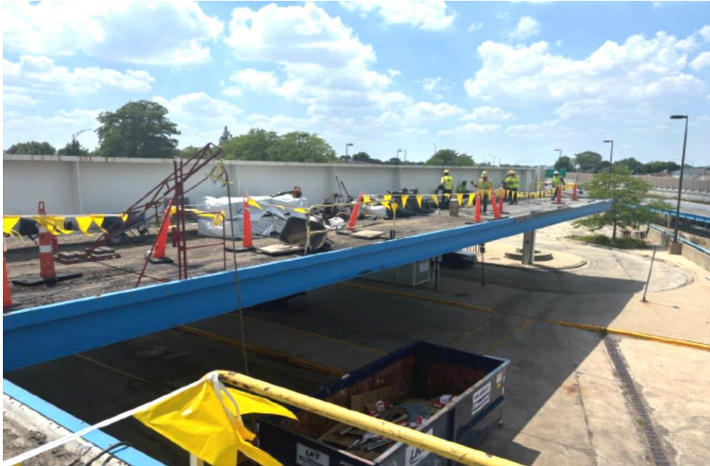
Bus Canopy Roof Replacement - Mobilization
