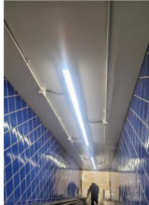
Chicago/Blue – Ceiling repairs and LED lighting
