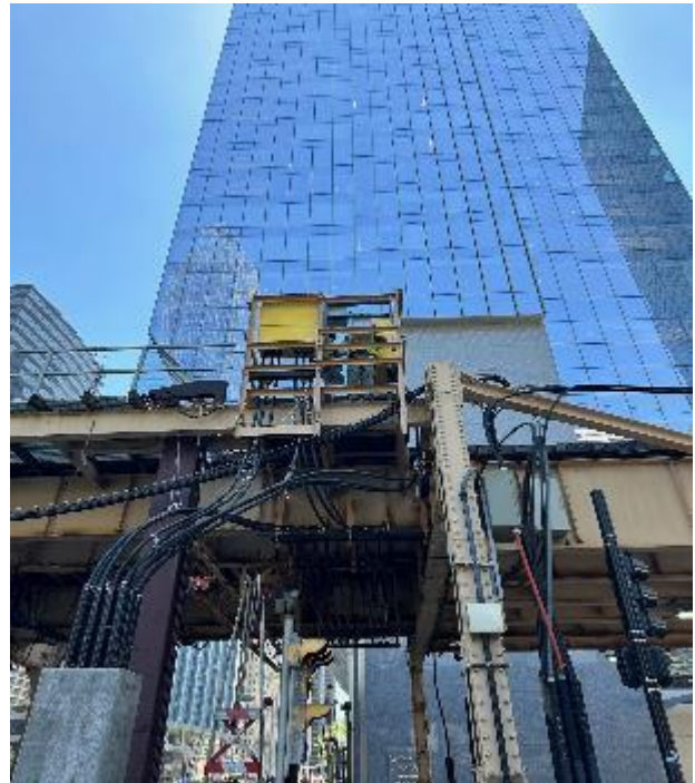
Section Gap and Cable Installation at Haymarket Substation
