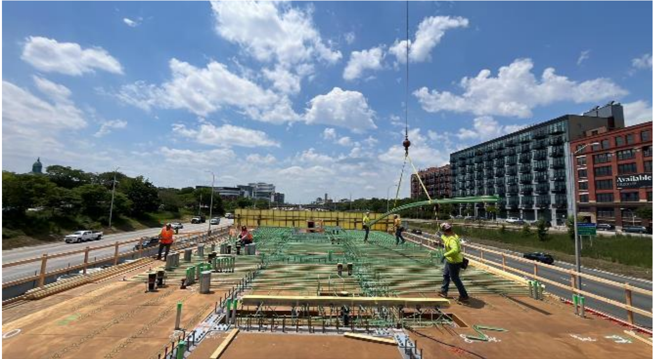
Racine Stationhouse Looking West, MEP, Rebar, and Form Work
