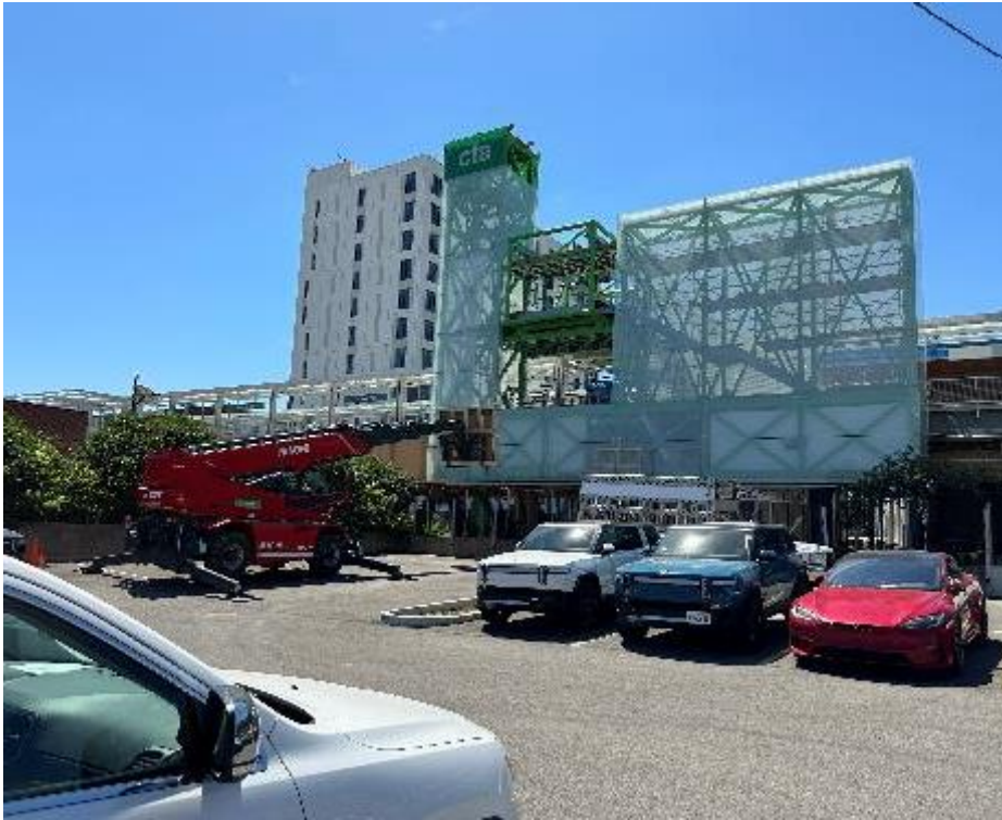
North Tower and Stair Enclosure from North
