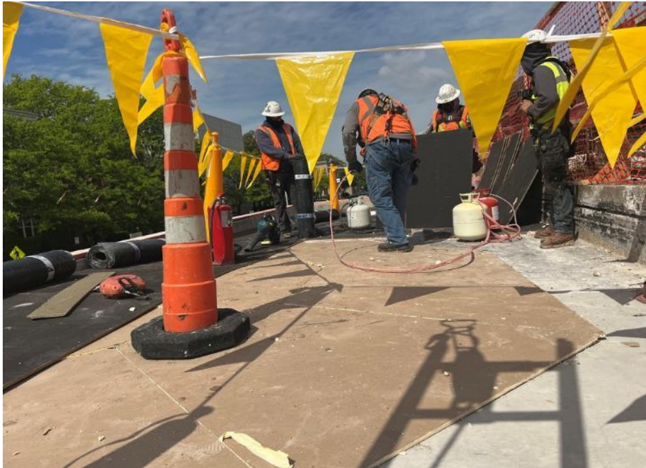
Installation of Roof at Mason Stationhouse
