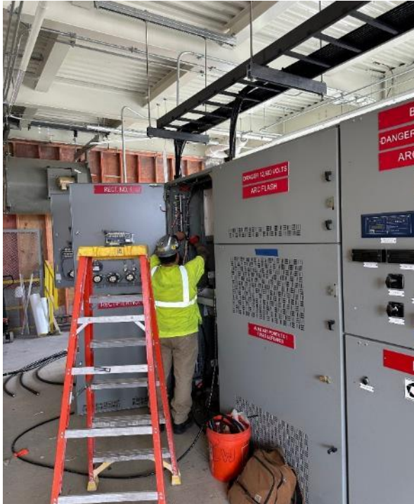
Control Cable Install and Testing at Barry
