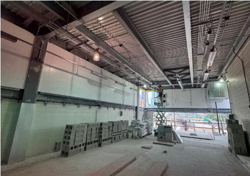
Morgan Substation Equipment Lighting Installation
