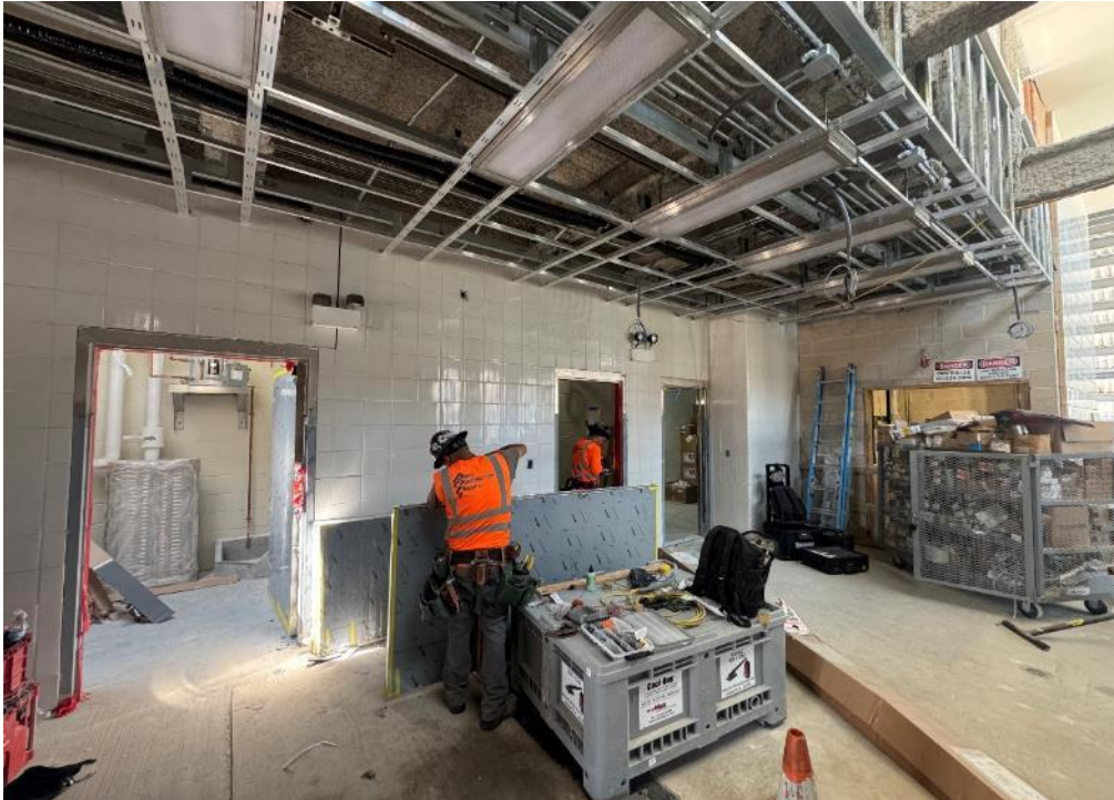
Racine Stationhouse Interior Doors
