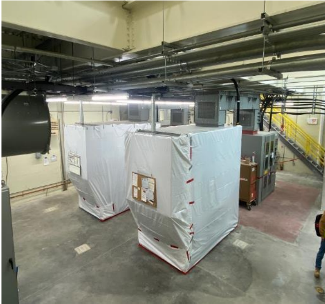
Prep for Traffic Coating Install at Damen
