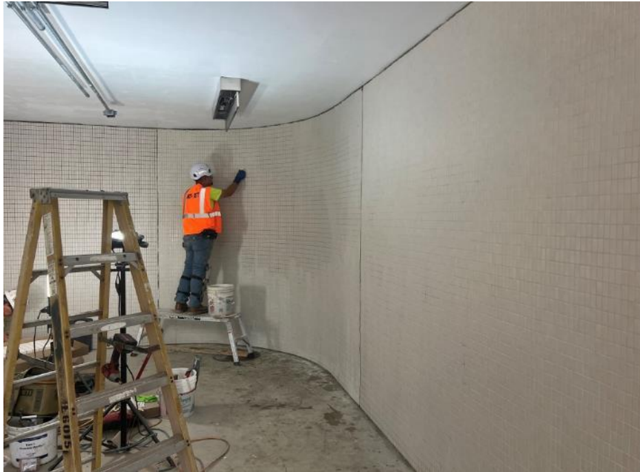
Installation of Ceramic Wall Tile
