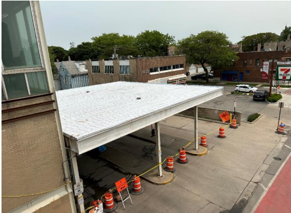
Completed Temporary Roof at Bus Canopy
