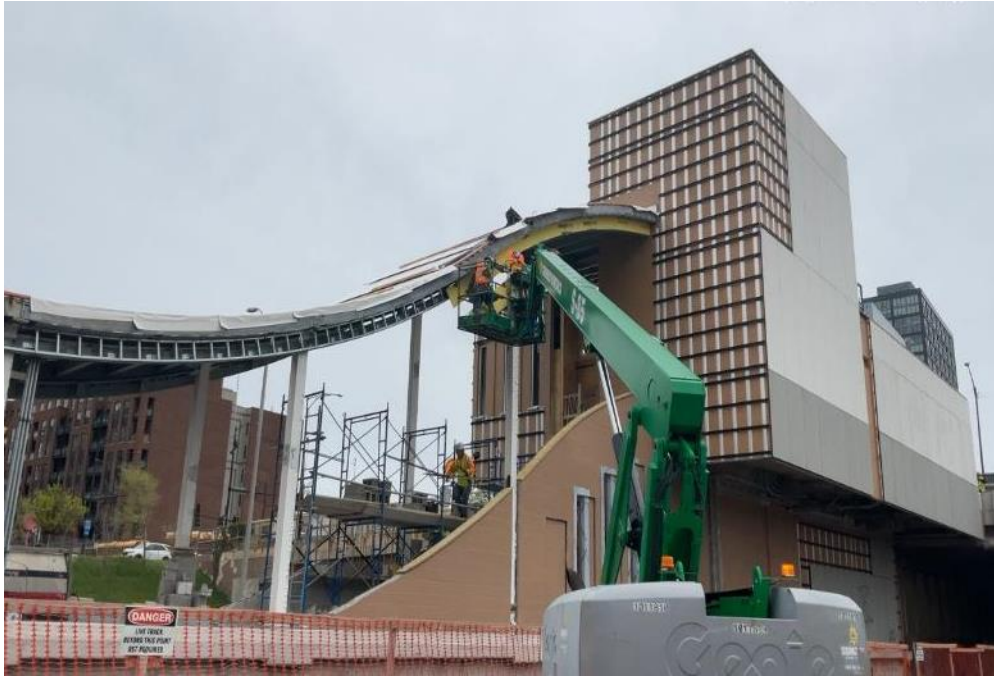
Racine Stationhouse Stairway Roofing Progress
