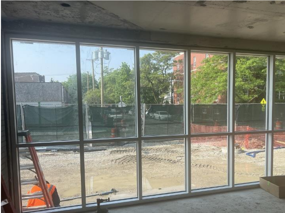
Installation of Storefront at Mason Stationhouse
