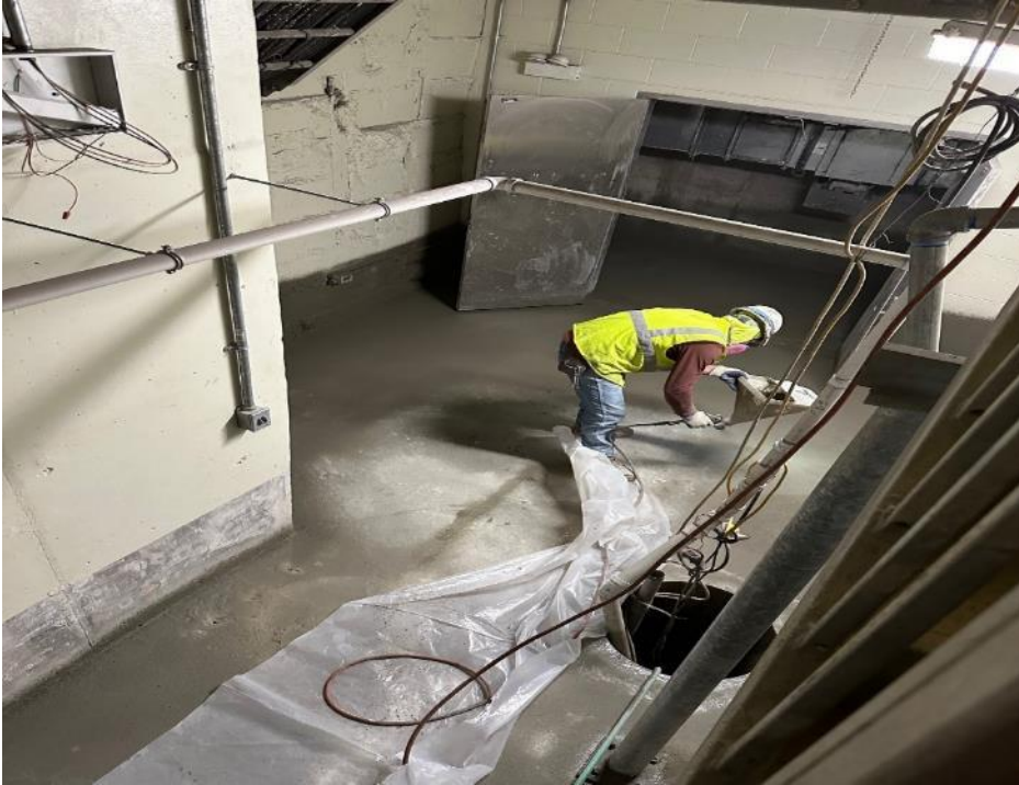
Waterproofing Install at Barry Subvaul
