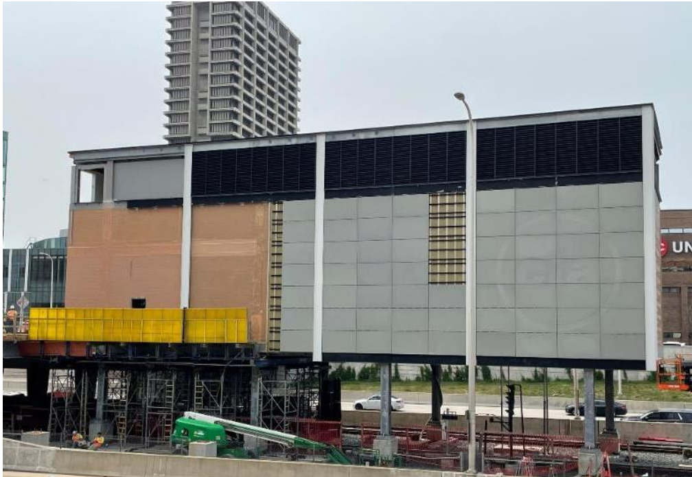
Morgan Substation Exterior
