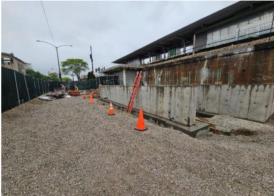
Installing Foundation Walls at Austin Stationhouse Addition
