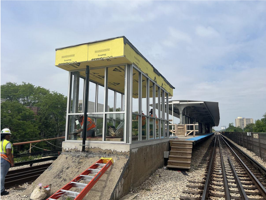
Newly Installed Aluminum Storefront at Mason Stationhouse Stair
