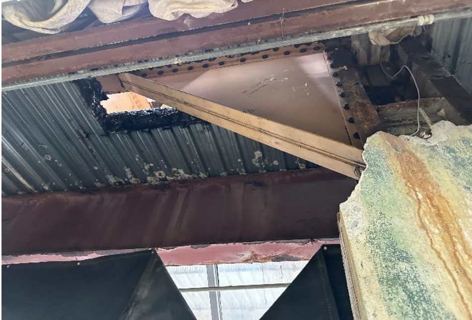
New Column Steel Installed
