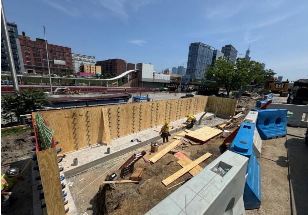
Racine Electrical Receiving Pit Progress
