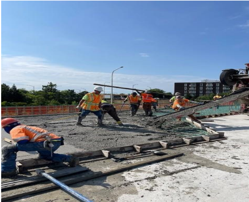
Backfill and Compactions Near South Abutment
