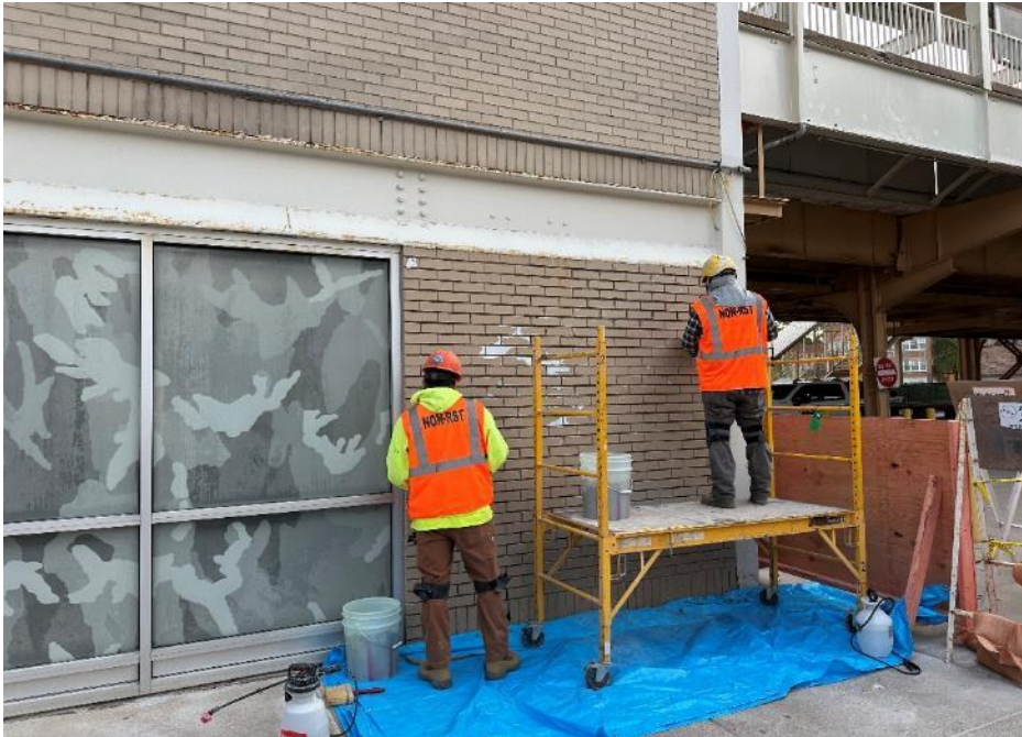
Station South Exterior - Tuckpointing Masonry
