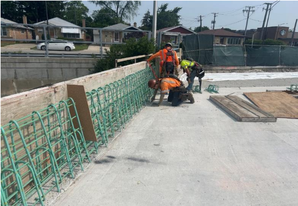
Installing Rebar and Formwork for Parapet Wall
