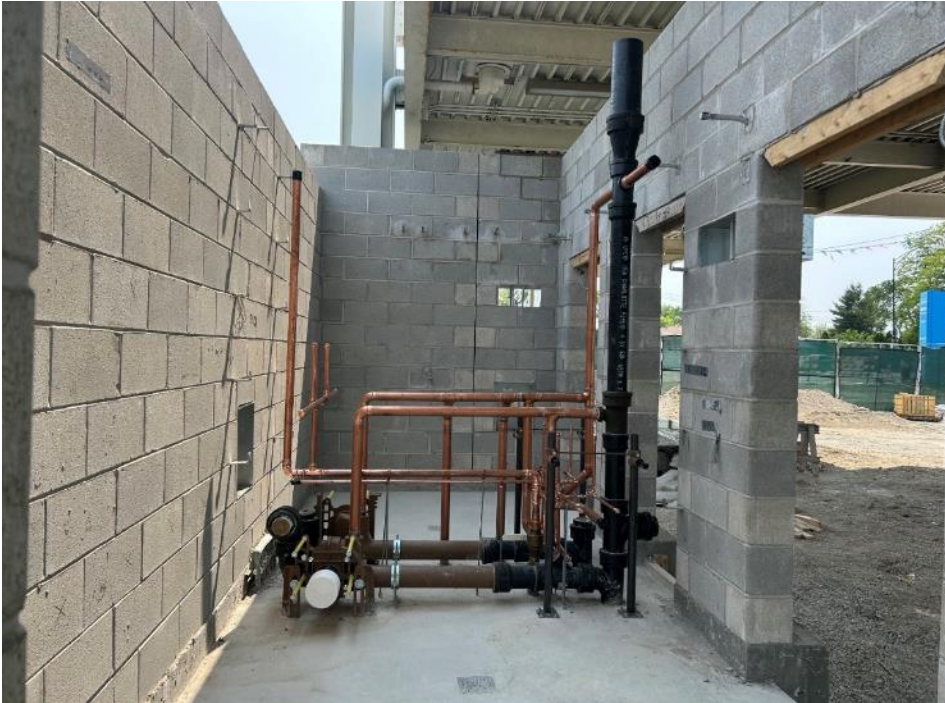
Plumbing Installed For Bus Washrooms
