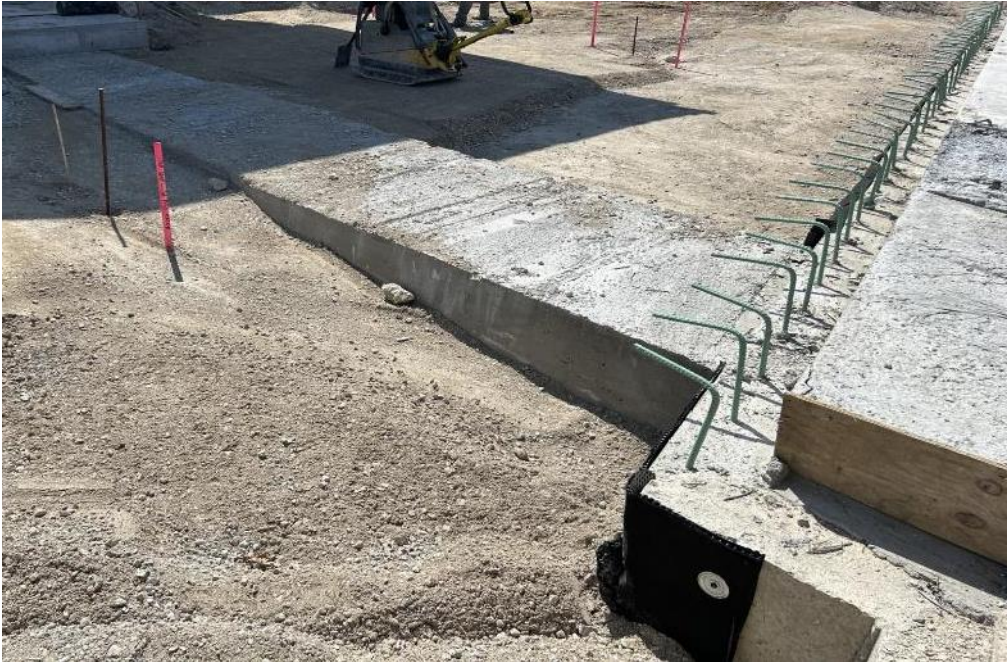
Installing Duct Bank, Electrical Manhole to Bridge Deck
