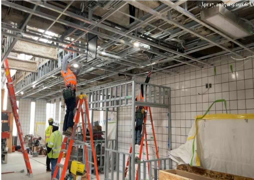
Racine Stationhouse Interior & CA Kiosk
