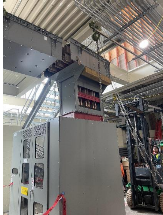
Traction Power Equipment Installation at Barry
