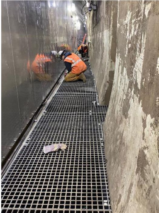
Permanent Foot walk Install at Canal Tie-House
