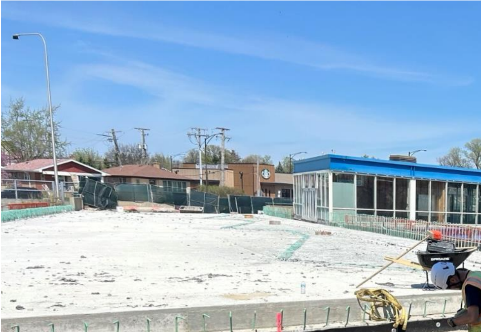
Completed Bridge Deck Pour
