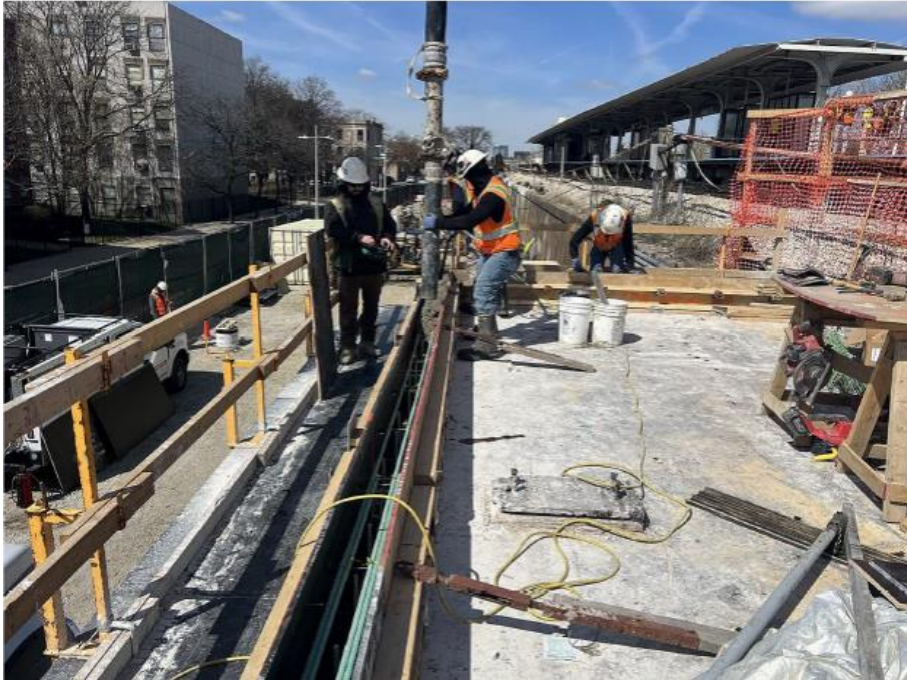
Pouring Roof Slab Extension at Mason Station
