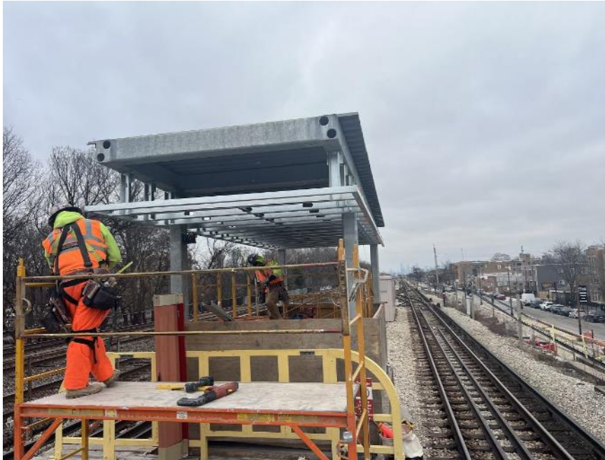
Installing Light Gauge Metal Framing at Mason Stairs
