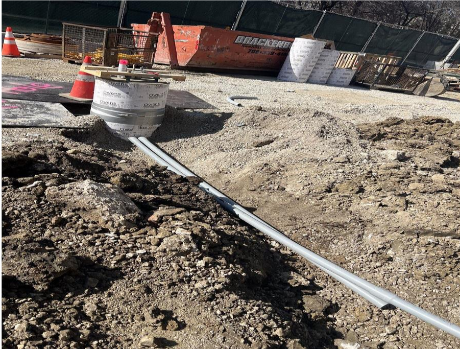
Installation of Street Light Pole Footings and Conduit
