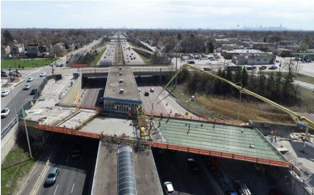
Aerial View of Bridge Deck Pour
