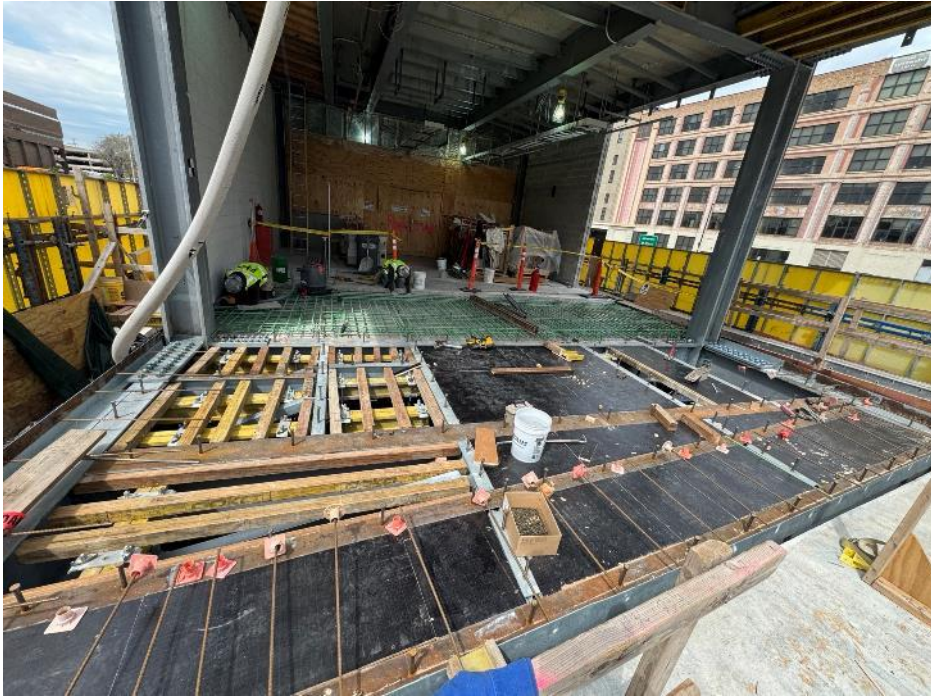
Morgan Substation Entrance Forms & Rebar Installation
