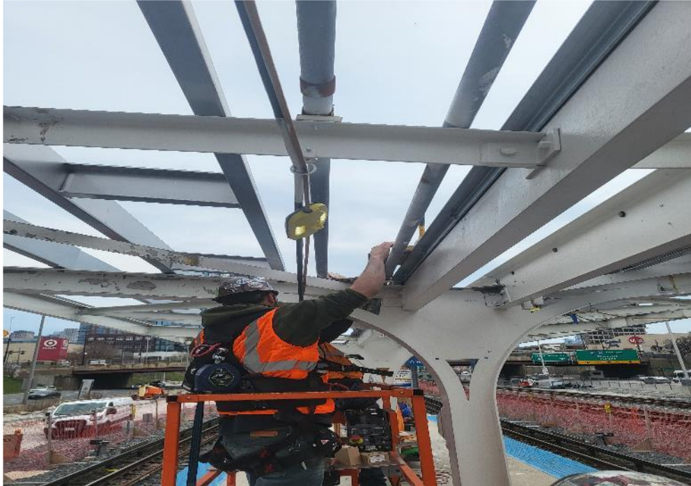
Racine Platform Canopy Purlin Installation
