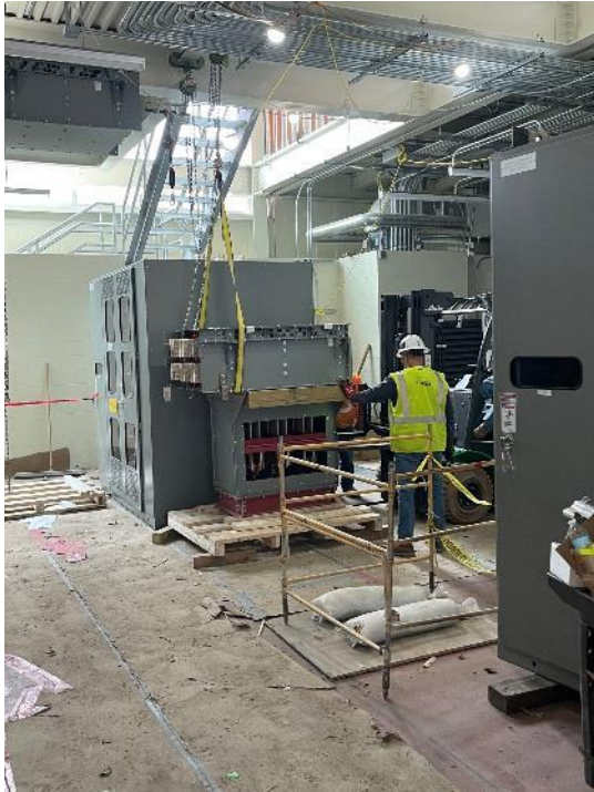
Traction Power Equipment Installation at Barry
