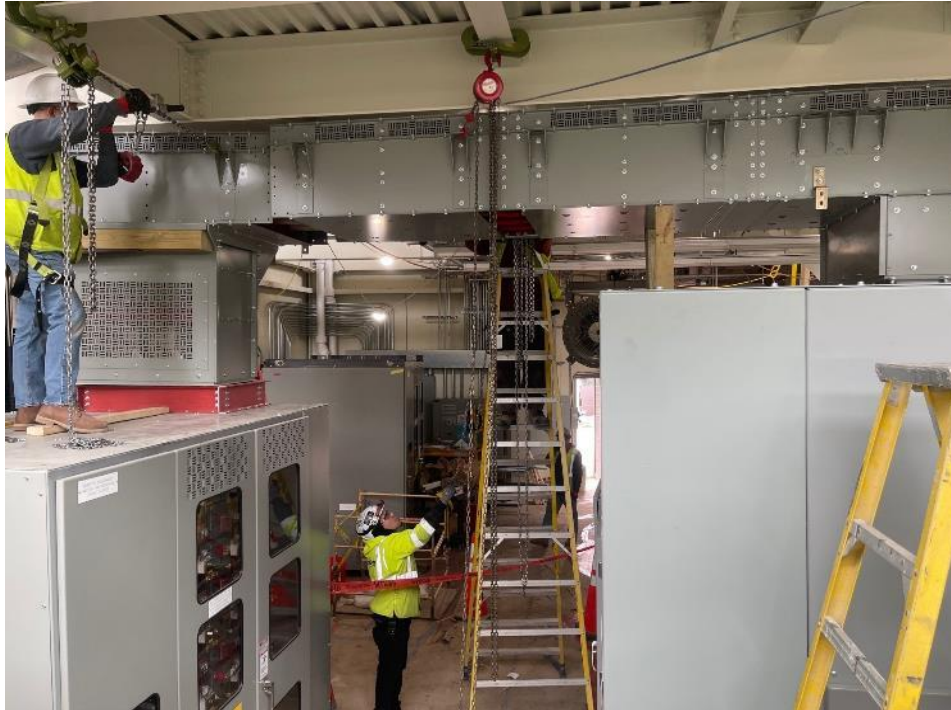
Traction Power Equipment Installation at Barry
