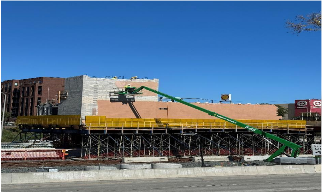
Racine Stationhouse South Wall Construction
