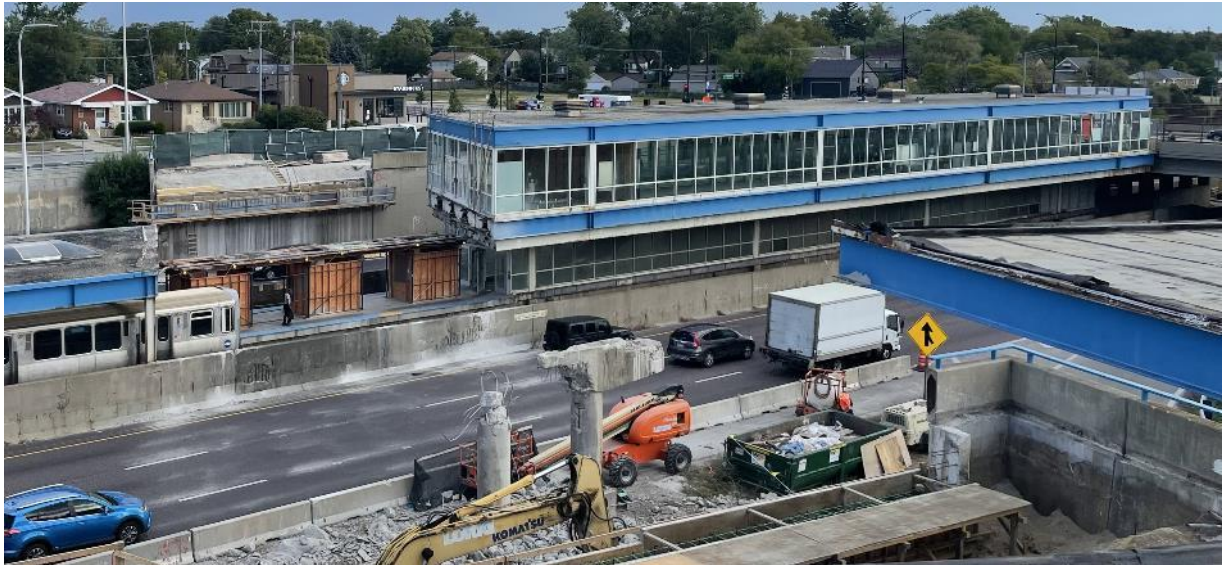
View of Station Looking North
