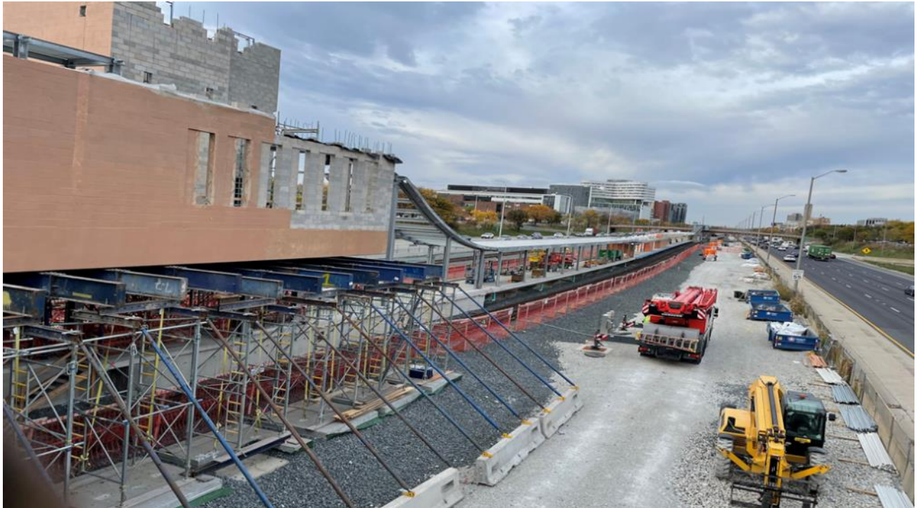
Racine Stationhouse North Wall Construction
