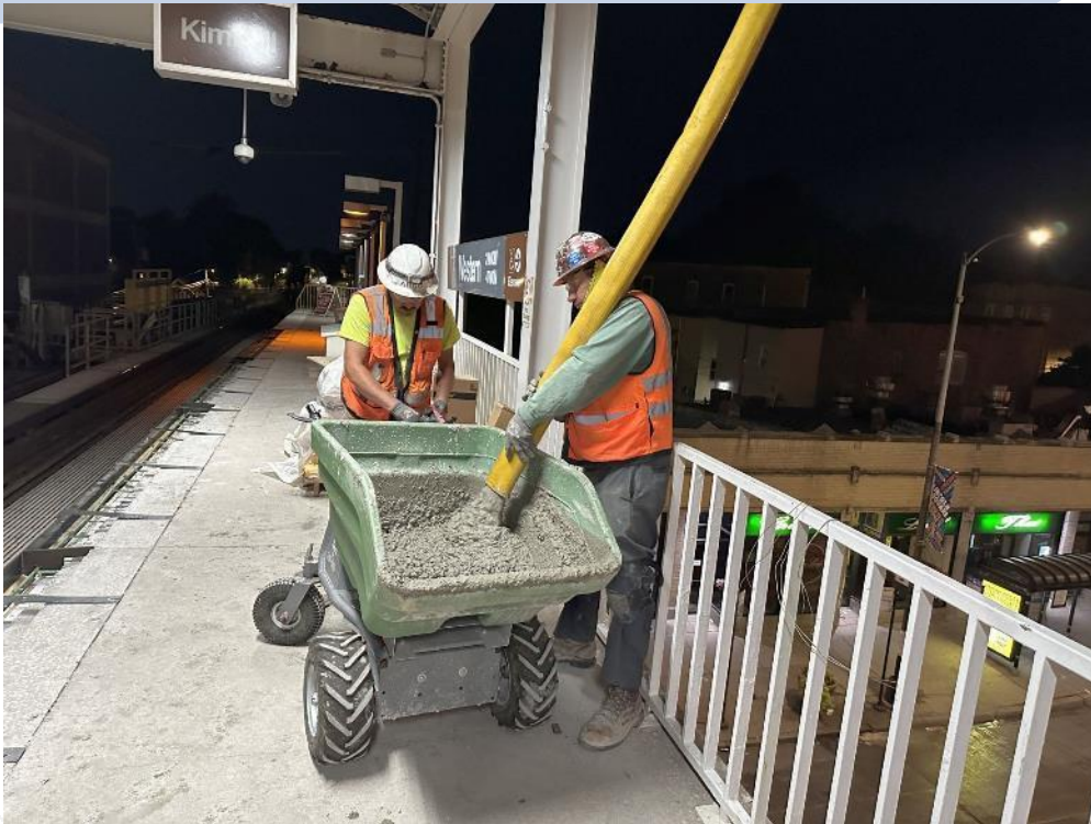
Pumping Concrete to Buggy from Western Avenue Median
