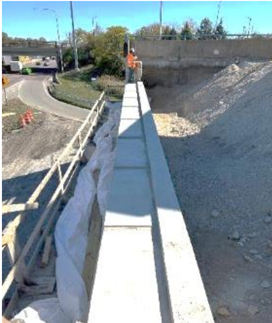
South Abutment Poured
