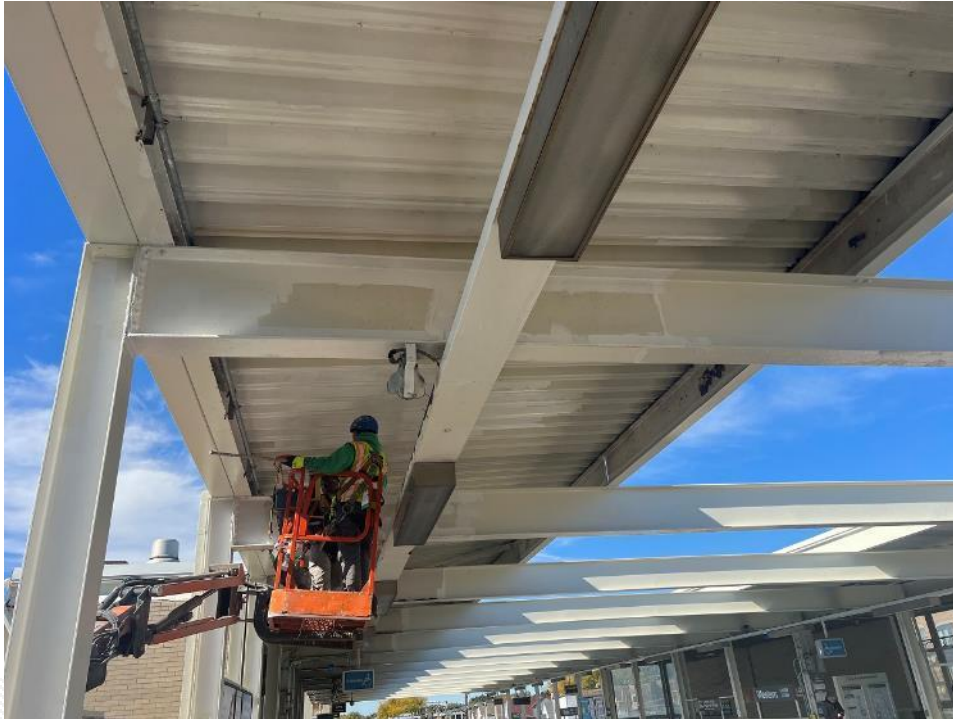
Inbound Platform – Painting Canopy Steel
