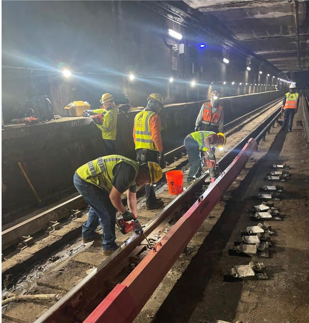
**Contractor Removing Old Fasteners and Plates.**
