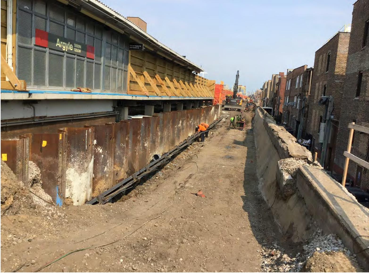
**LBMM – Soil Anchor Installation and Excavation**
