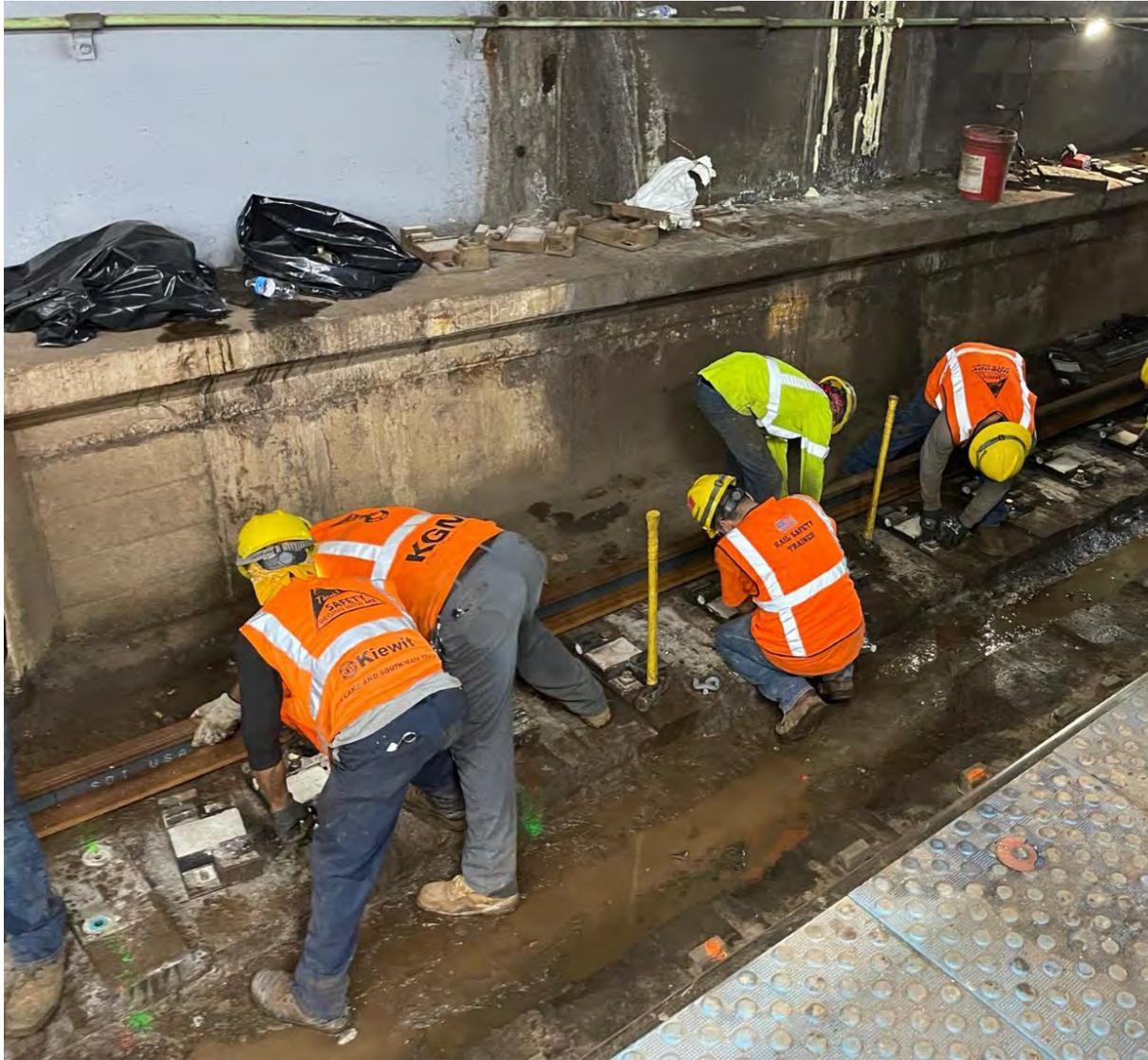
**Contractor Installing New Rail, Plates, and Fasteners**
