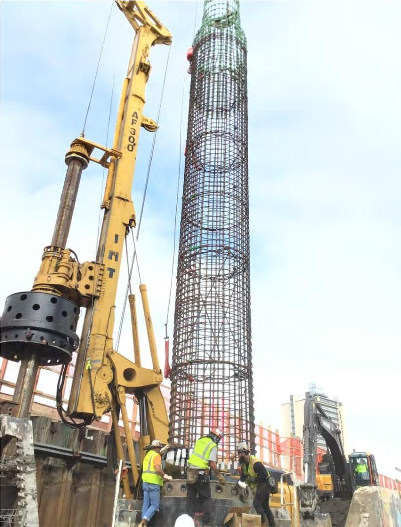
**LBMM – Caisson Rebar Cage Installation**
