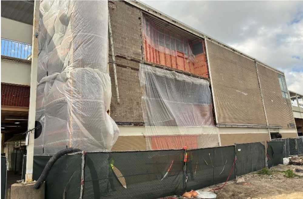
Masonry Demolition North Wall
