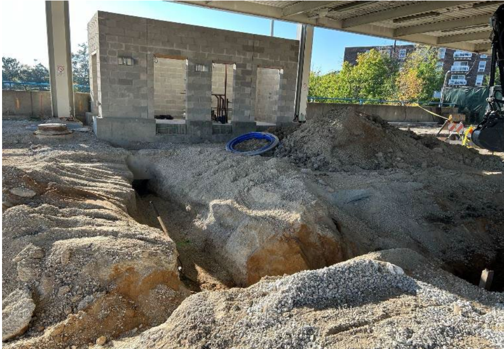
Trench for new water service at Washroom
