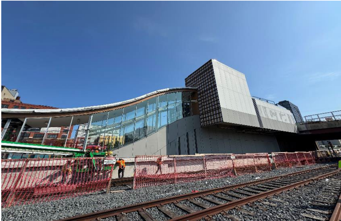
Racine Stationhouse & Stairway Looking North
