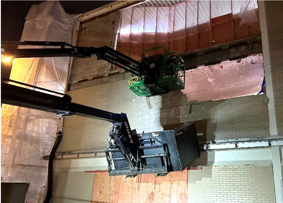
Masonry Demolition North Wall
