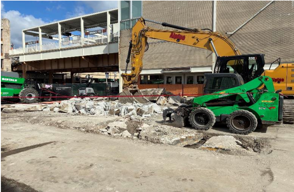
Bus Canopy Foundation Demolition
