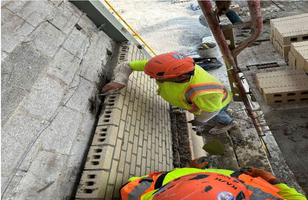
Masons Replacing Face Brick on Exterior Wall
