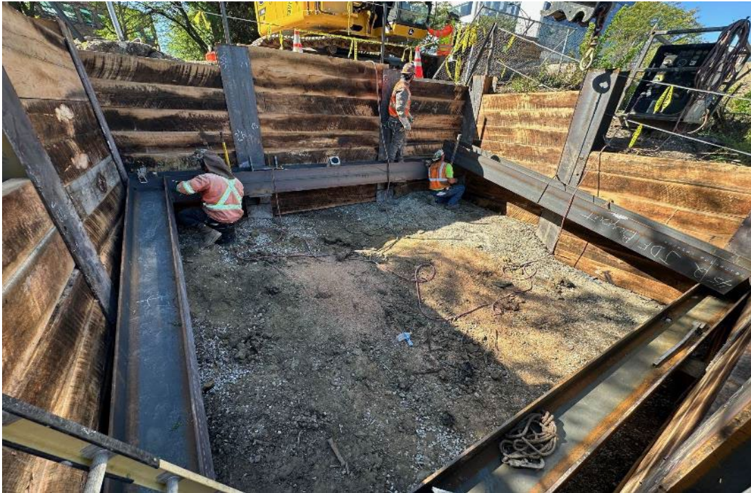
Loomis Sanitary Receiving Pit ERS Installation
