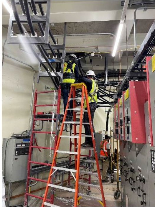
Barry Cable Installation
