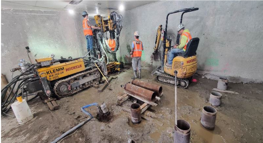
Micropile Drilling at Austin Stationhouse Elevator Location
