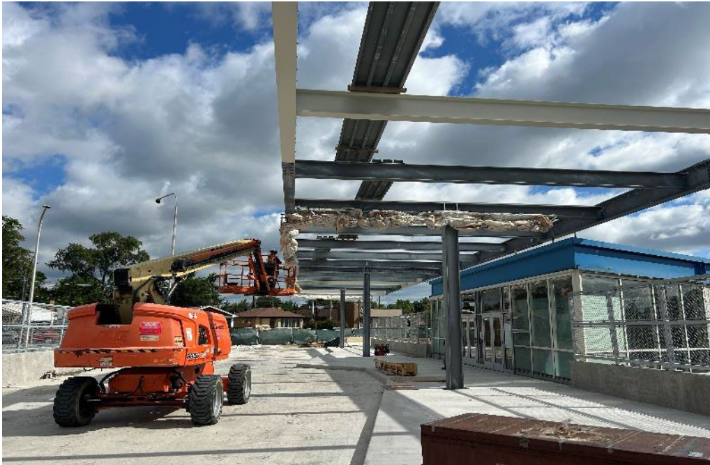
Installing Overspray Protection on Bus Canopy
