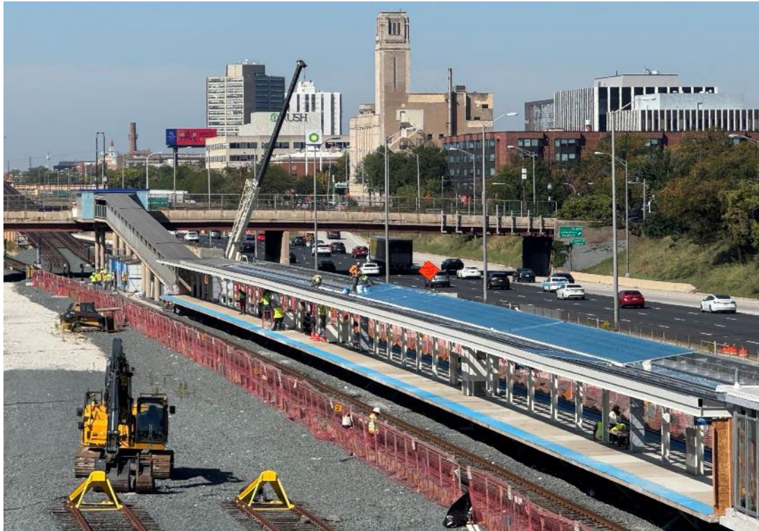
Racine Platform Canopy Roof Panels
