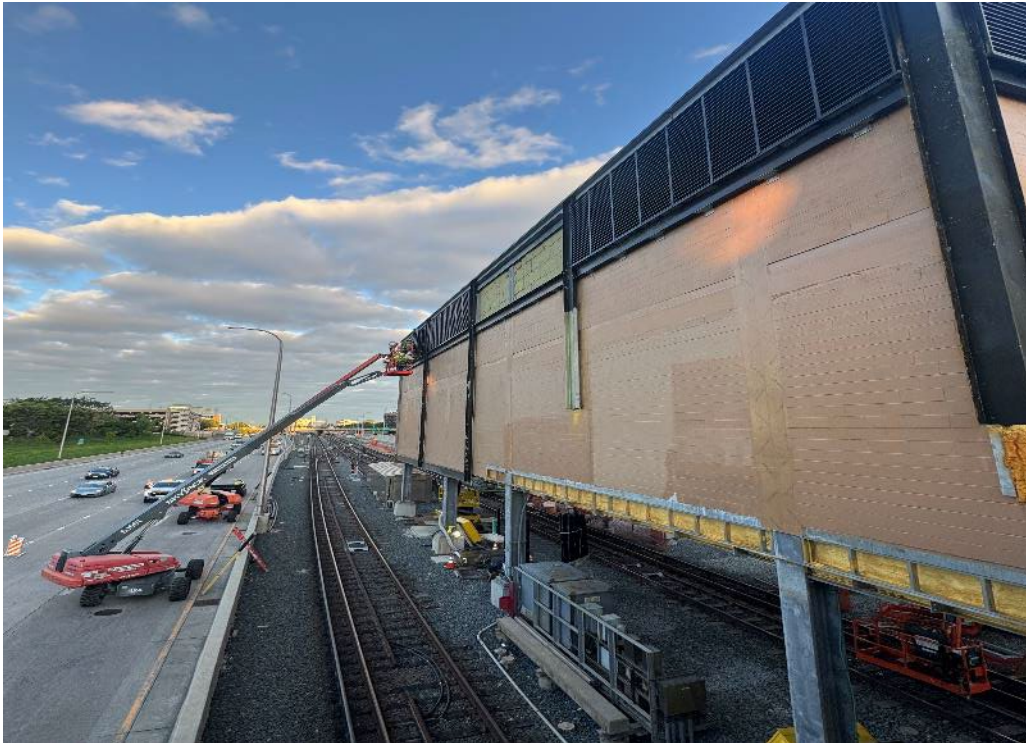
Morgan Substation Louvers – South Wall
