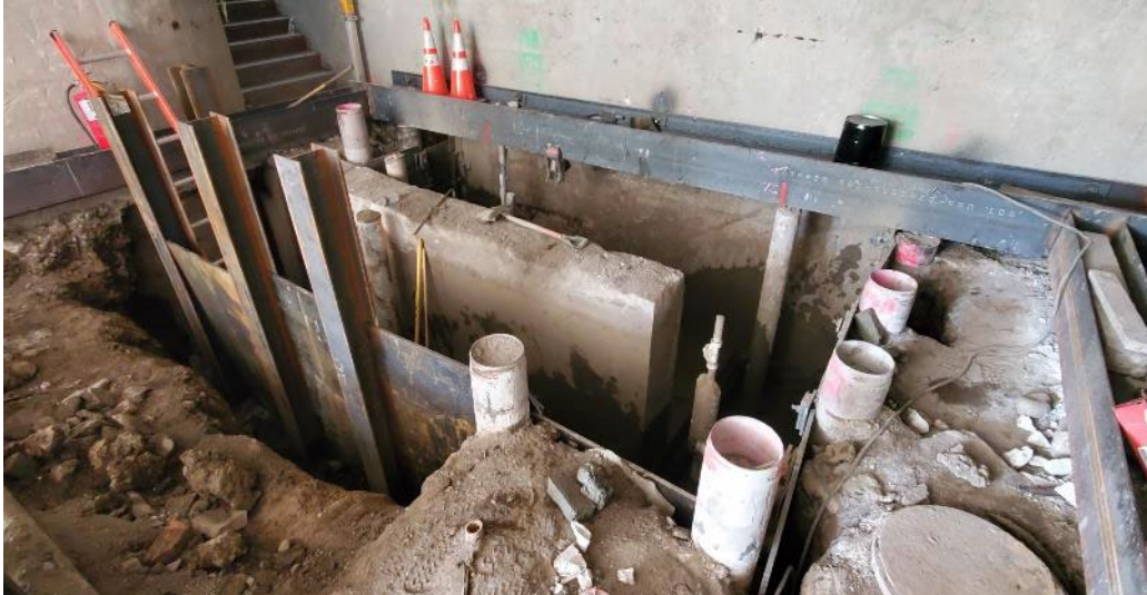
Micropiles Installed at Austin Stationhouse Elevator Location
