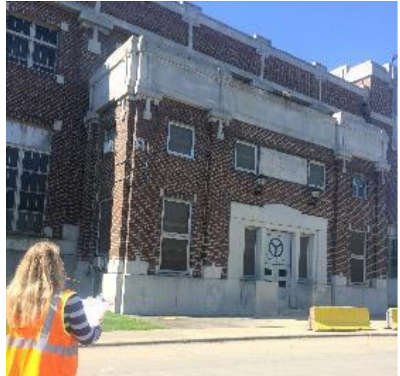
Pictured: Field survey work near the Historic Roseland Pumping Station.
