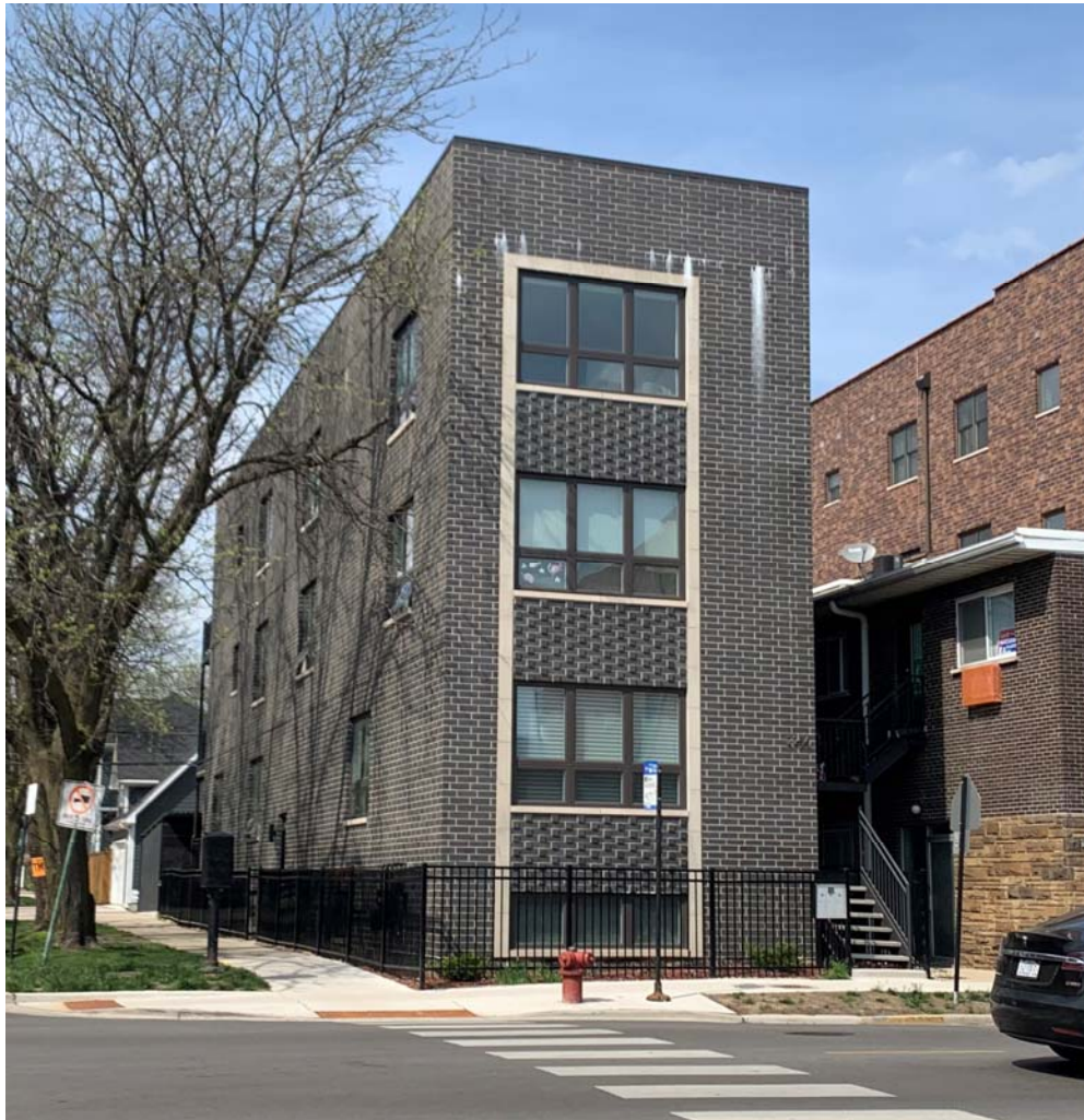
Housing – Foster Avenue
