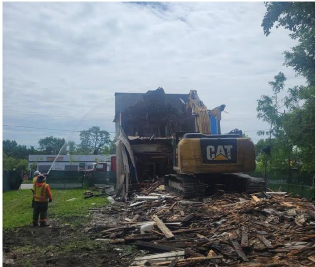
Property demolition where new Red Line track will be built
