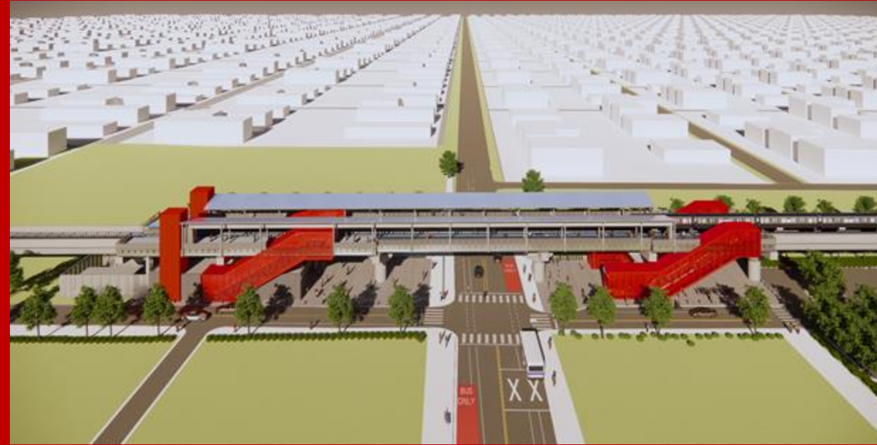
103rd Street Red Line Station
