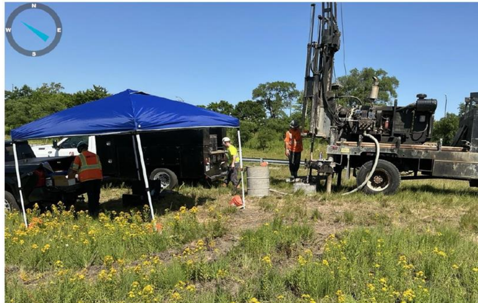
Soil boring work ahead of drilling new foundations for future track
