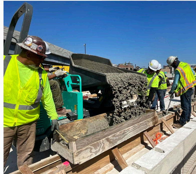
Concrete pour, RPM Phase One Project
