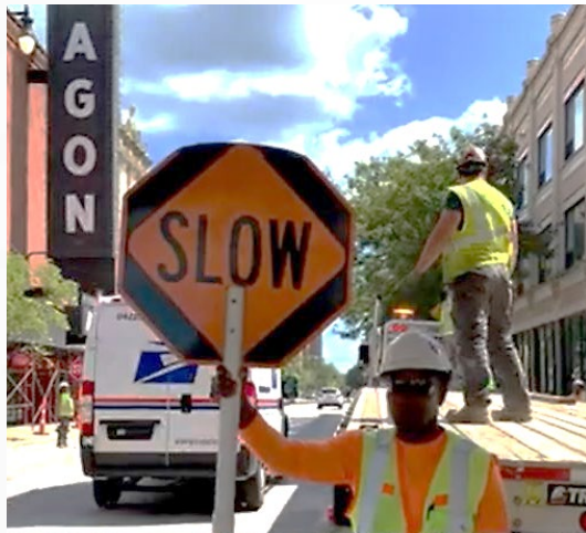
Top, Allstate Concrete Cutting; bottom, Air & Wellness Safety Training, RPM Phase One Project
