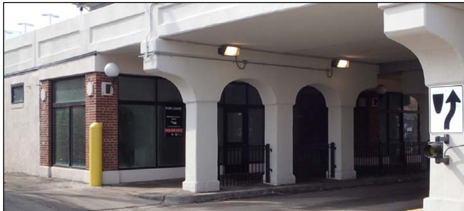
Figure 6-4: Photo of CTA-Owned Retail Building at Argyle Station
