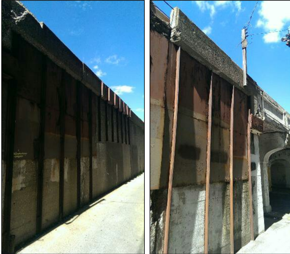
Figure 4-10: Embankment Wall on East Side of Track near Balmoral Avenue (left) and Embankment Wall on East Side of Track near Winona Street (right) with Shoring/Plating Repairs for Structural Support
