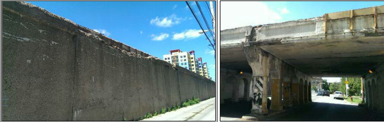
Figure 4-8: Photos of Deteriorating Structures; Balmoral Avenue Viaduct and Embankment Wall Facing Northwest (left); Winona Street Viaduct Facing West (right)
