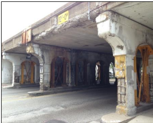
Figure 1-6: Photo Showing Current Condition of Deteriorating Concrete Viaduct Requiring Shoring at Hollywood Avenue
