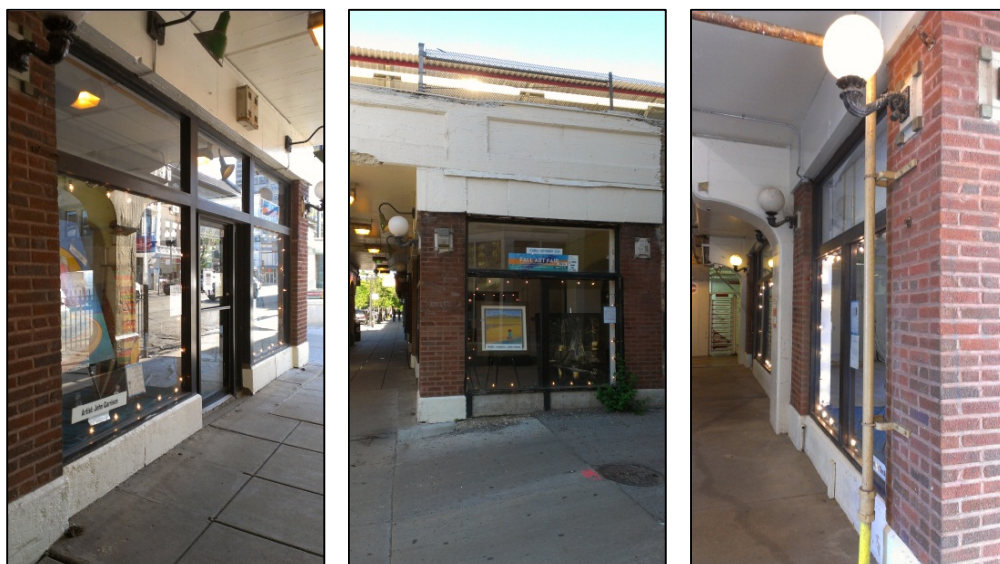
Figure 6-5: Photos of CTA-Owned Retail Building at Bryn Mawr Station
