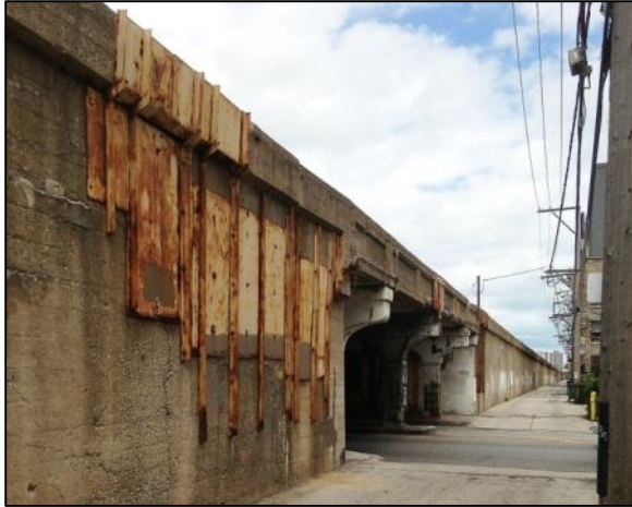
Figure 1-5: Photo Showing Current Condition of Embankment Wall at Hollywood Avenue
