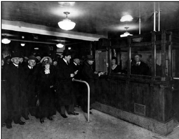
Figure 4-4: Lawrence Station Opening, February 1923
