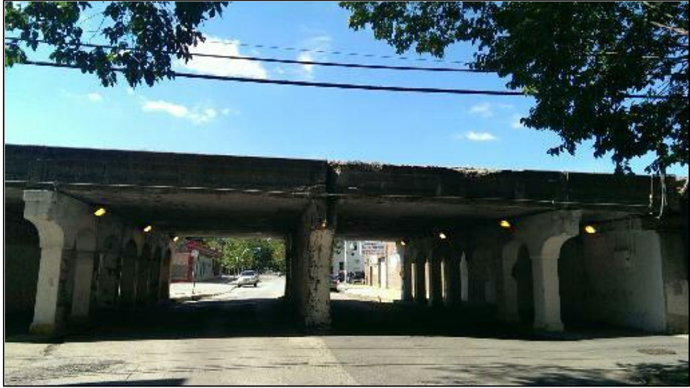
Figure 2-7: Photo Showing Existing Viaduct at Balmoral Avenue with Piers in the Roadway and Sidewalks
