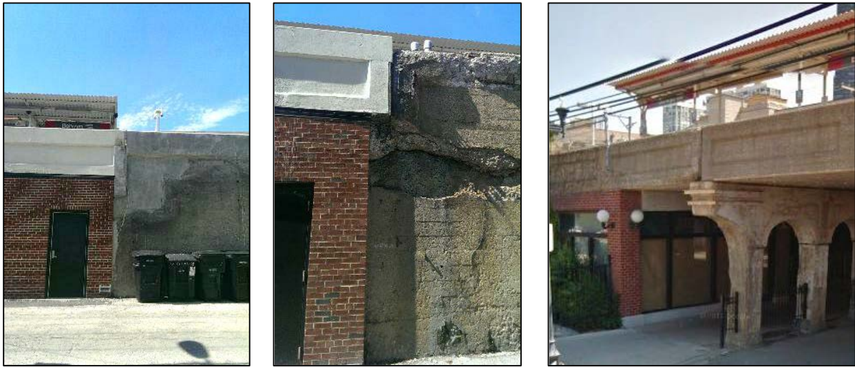
Figure 4-9: Photos of Deteriorating Embankment Walls and Viaduct Adjacent to Newer (2012) Structures at Argyle (left) and Berwyn (middle and right) Stations
