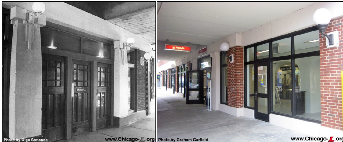
Figure 6-3: Views of Argyle Station Circa 1985 and 2012
