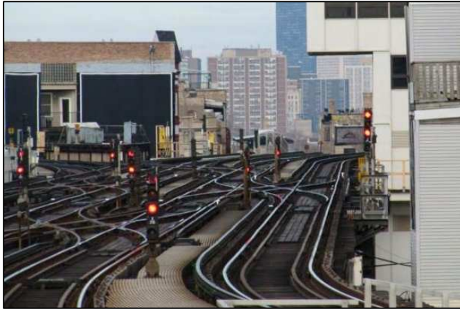
Figure 1-6: Photo of Clark Junction
