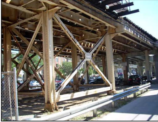
Figure 5-2: CTA Elevated Track Structure
