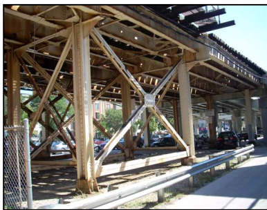
CTA Elevated Track Structure -
