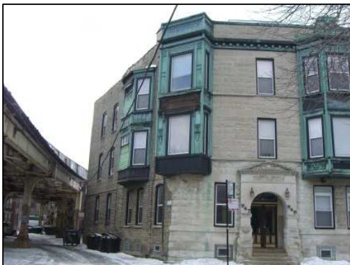
Figure 5-3: Vautravers Building (Facing South)
