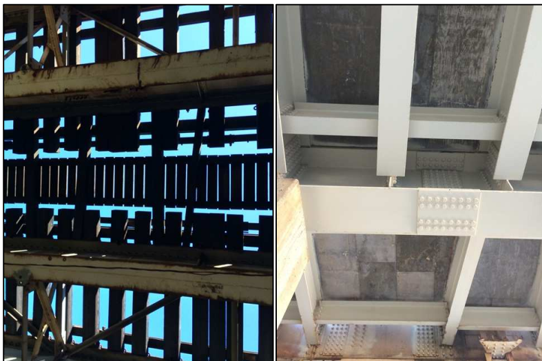
Figure 3-9: Photos of Open-Deck Track Structure (Left) and Closed-Deck Track Structure (Right), Viewed from Below
