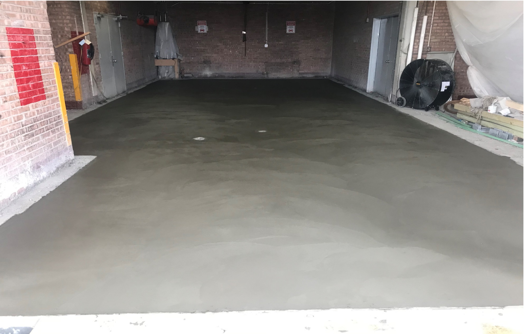
Penthouse Floor Slab
