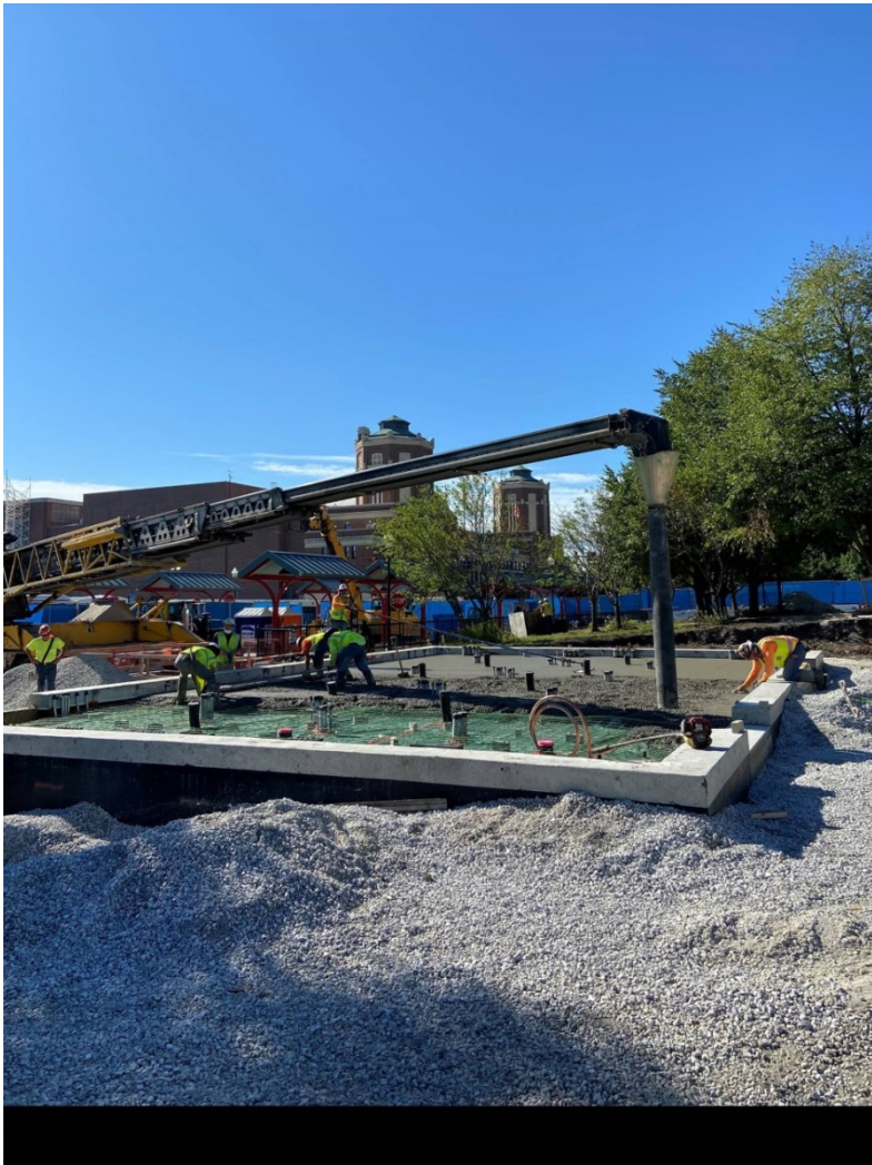
Building Foundation Installation
