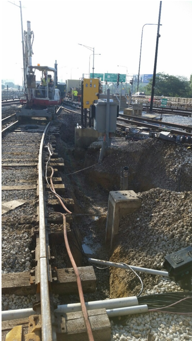
Excavation and Foundation Installation at Rosemont
