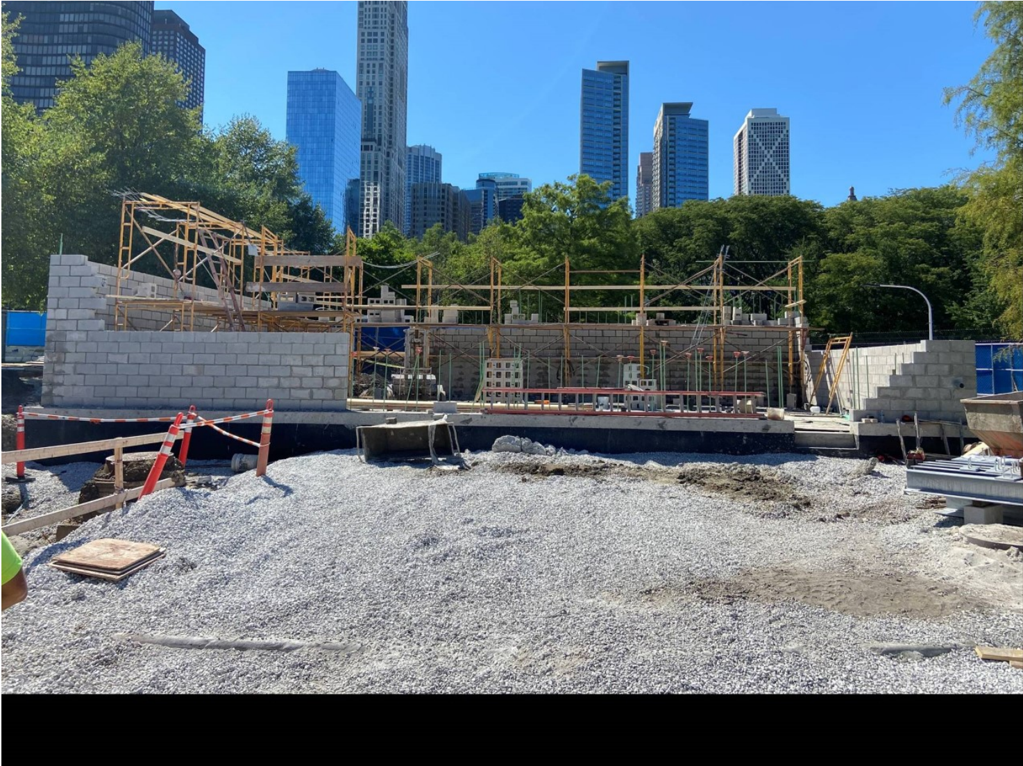
Exterior Building Construction
