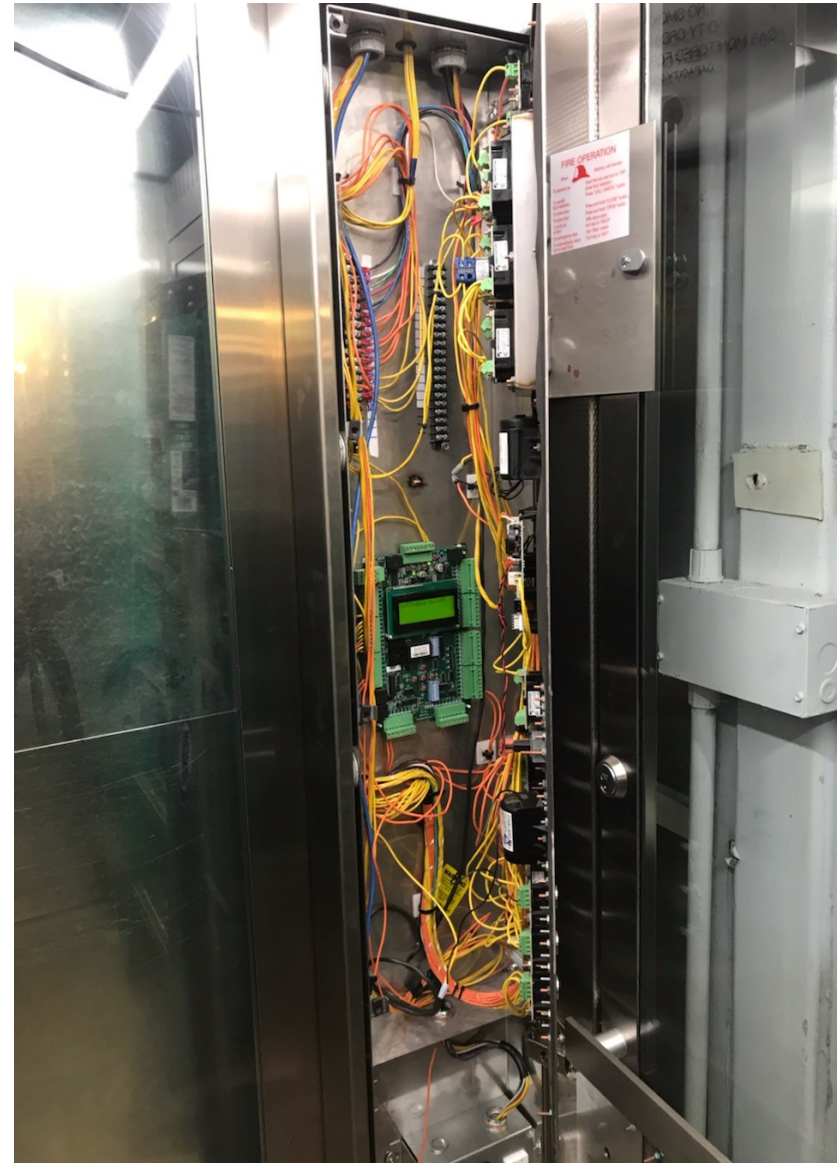
Elevator #1 - New elevator controller and cab wiring installation
