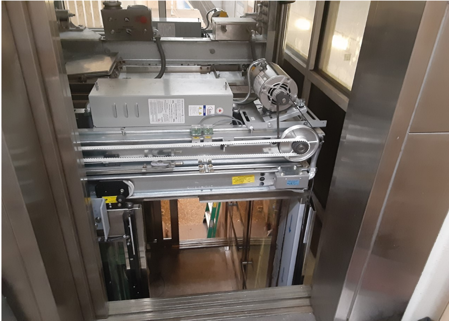
Elevator #1 - New elevator cab equipment/hardware installation
