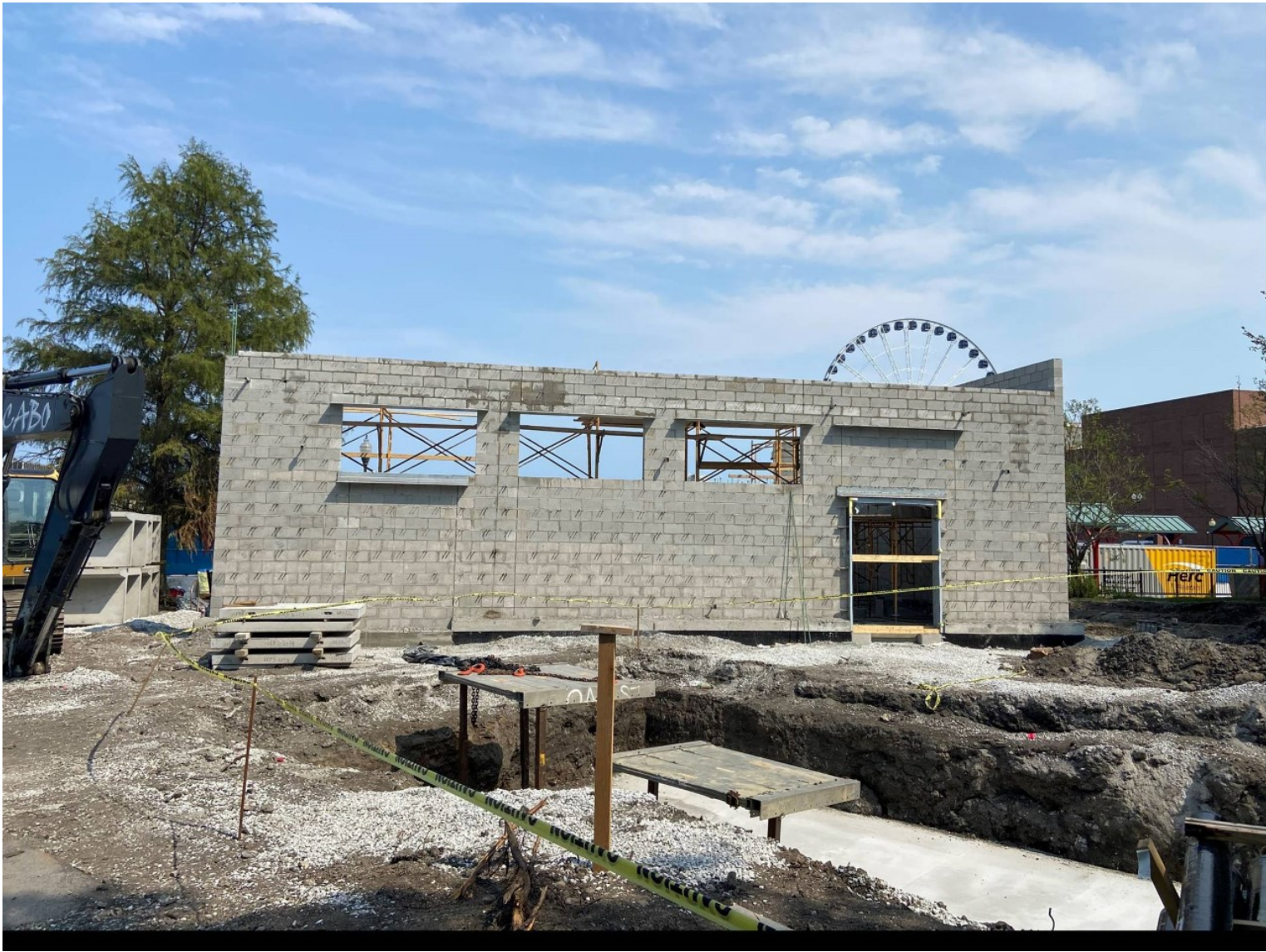
West wall of the new facility
