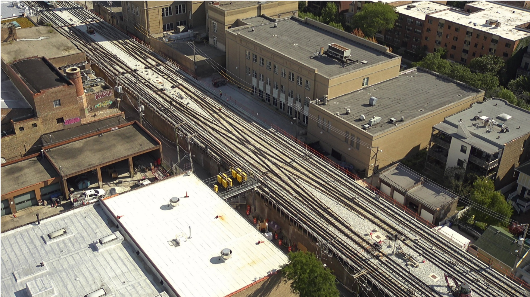
Lawrence to Bryn Mawr Modernization – Completed Trackwork at Thorndale Interlocking
