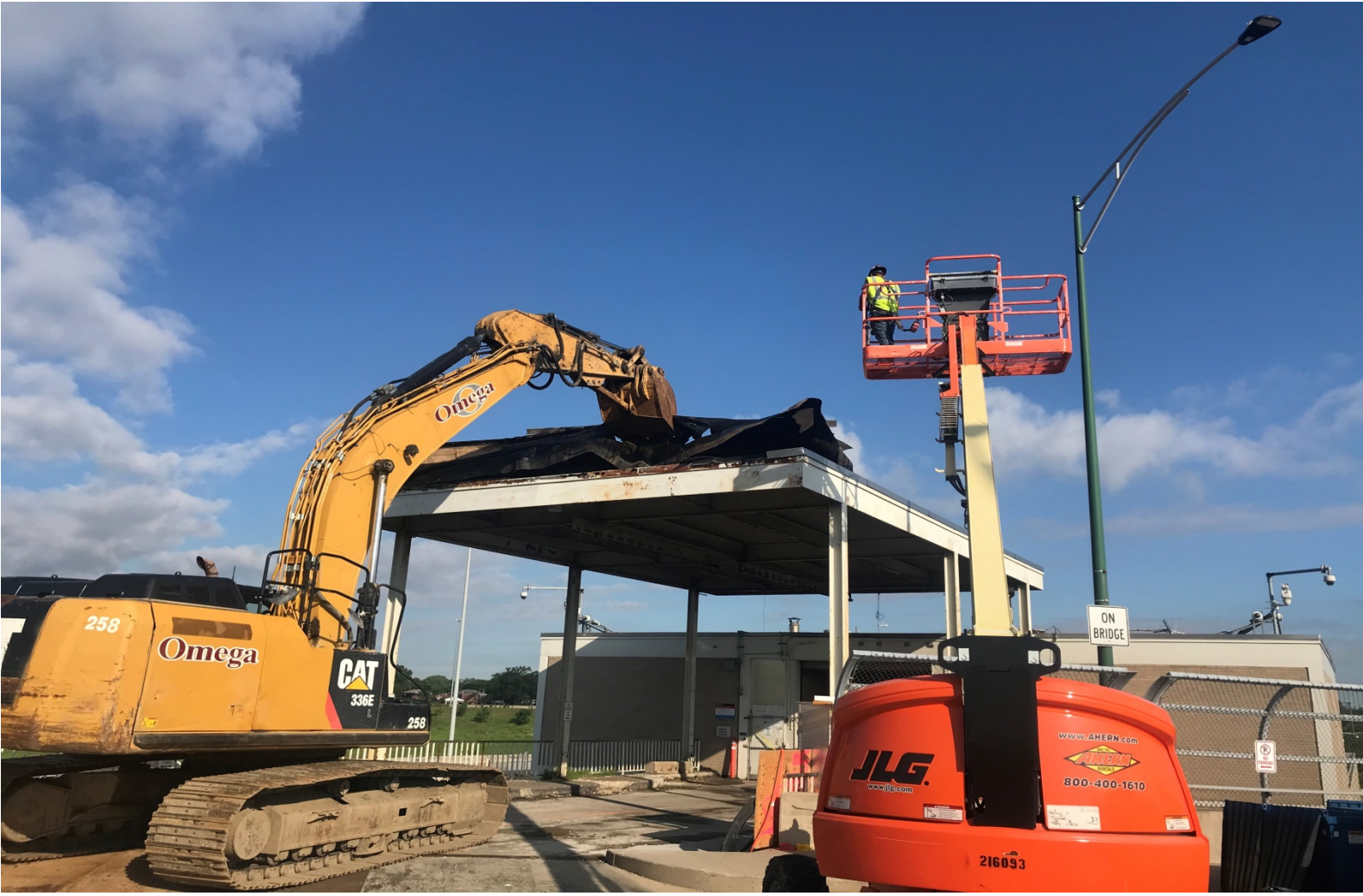
98 th Rail Shop Canopy Demolition
