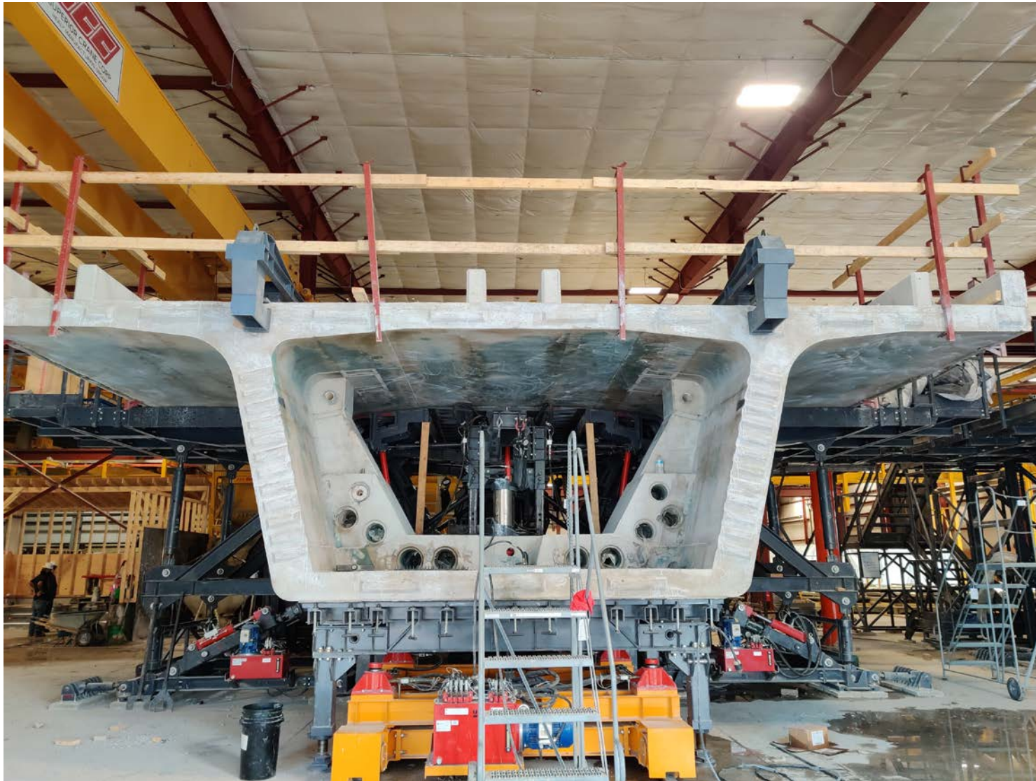
Lawrence to Bryn Mawr Modernization - Pre-cast Box Girder Production
