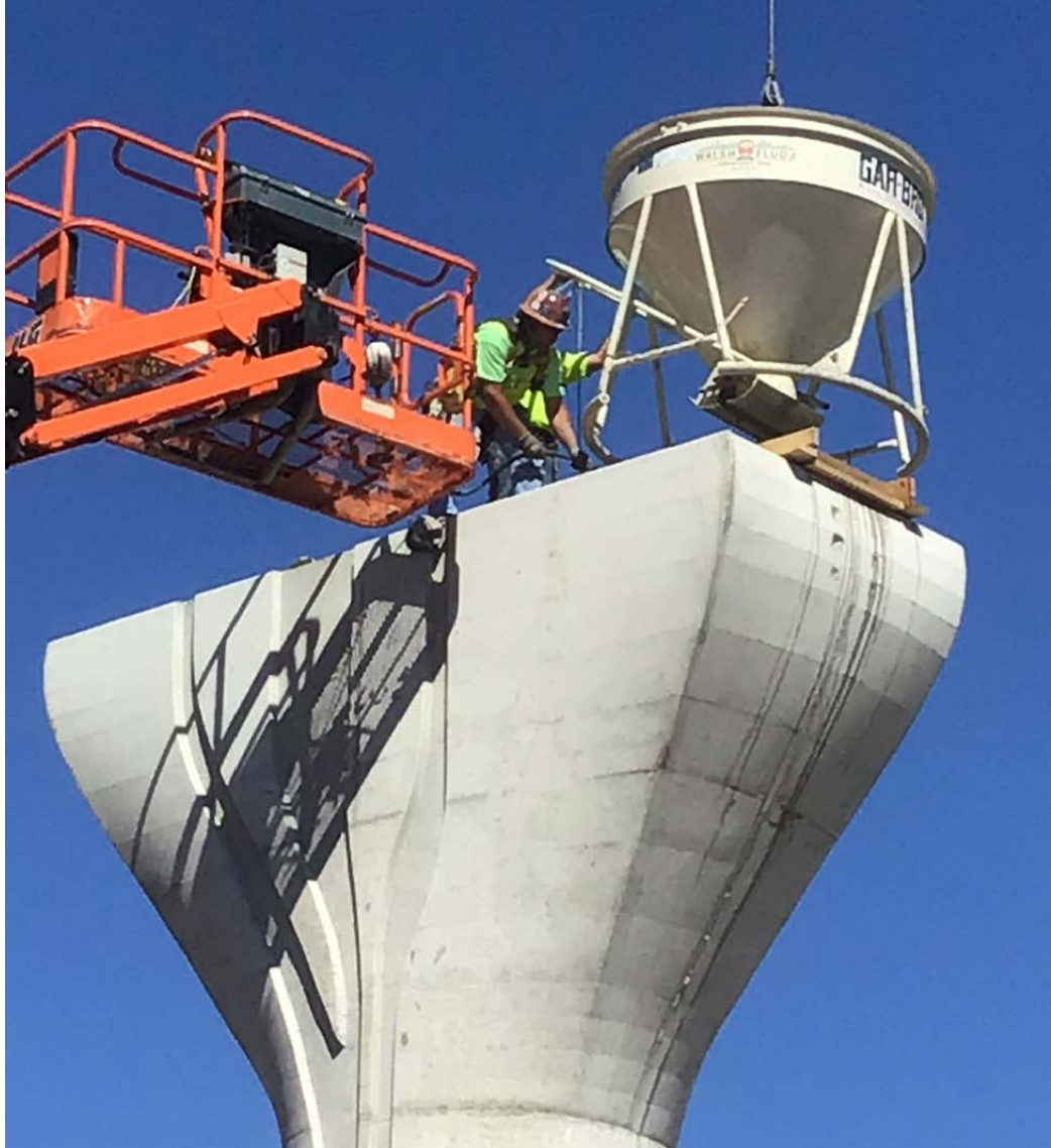
Red-Purple Bypass – Pouring Beam Seats
