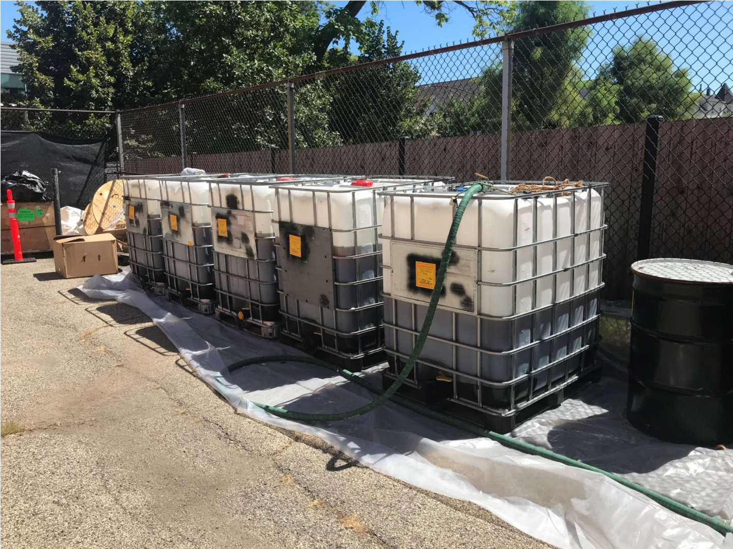
Draining Oil From Existing Transformer and Discharging it into Totes
