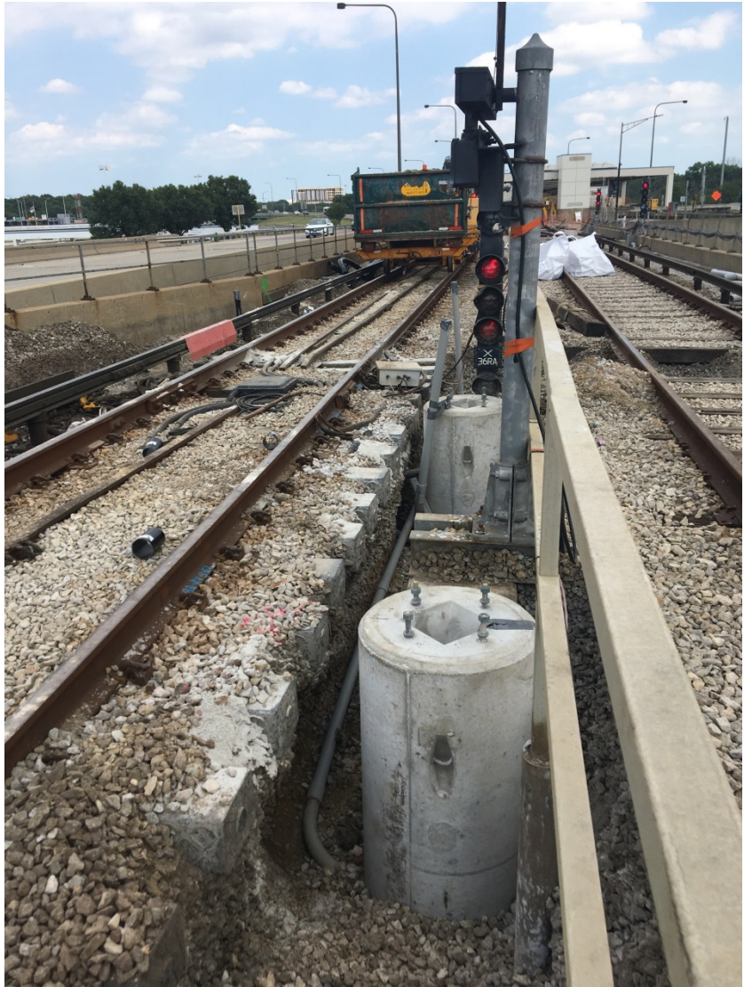
Excavation and Foundation Installation at Rosemont
