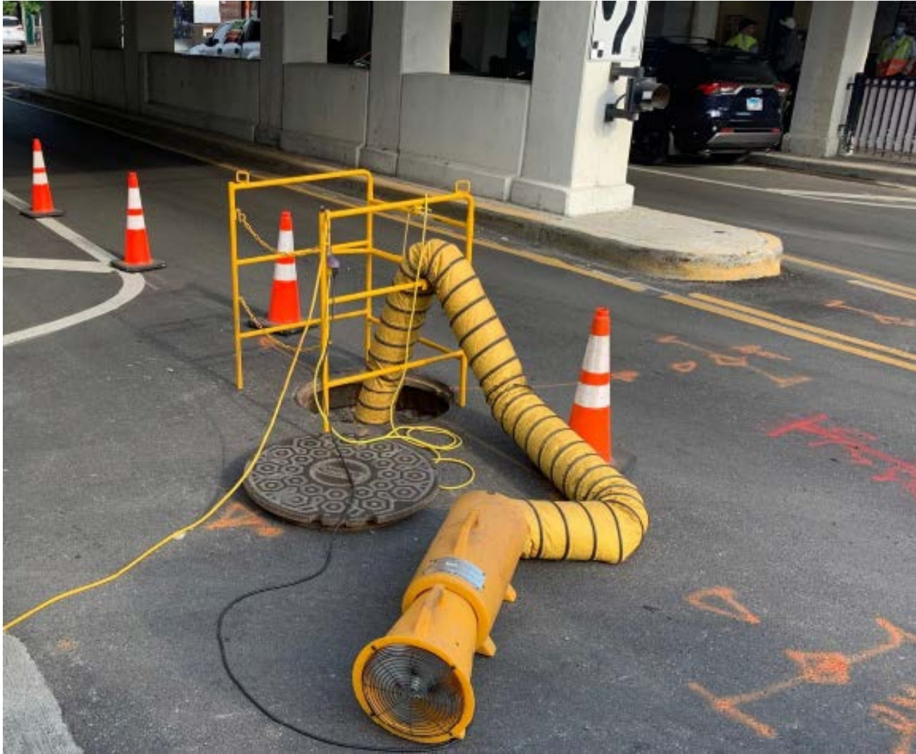
AT&T Splicing Copper at Argyle Manhole
