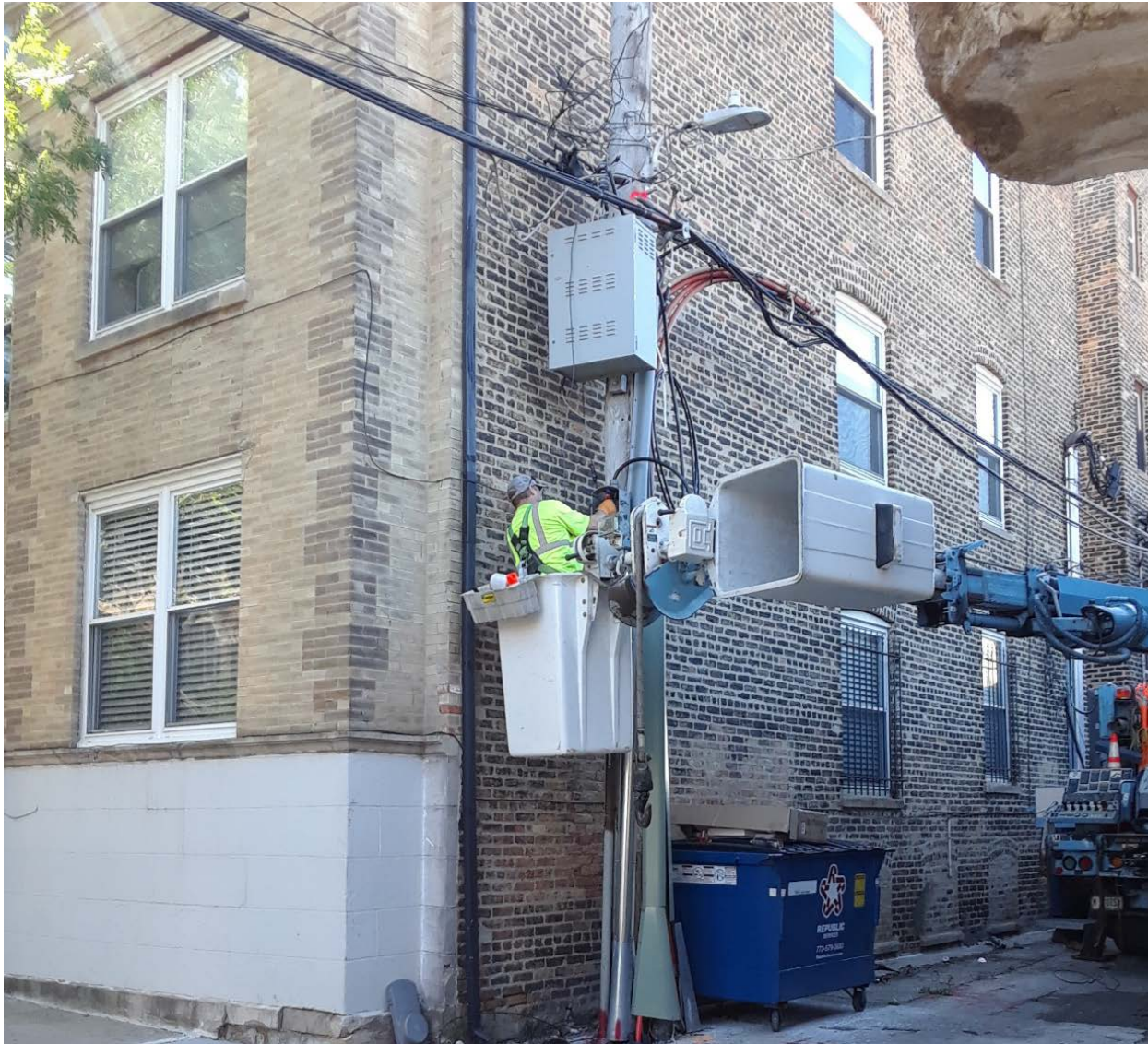
DEO work at Winona Street
