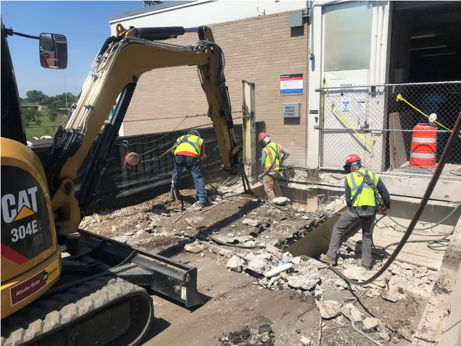
98 th Rail Shop Bridge Deck Demolition
