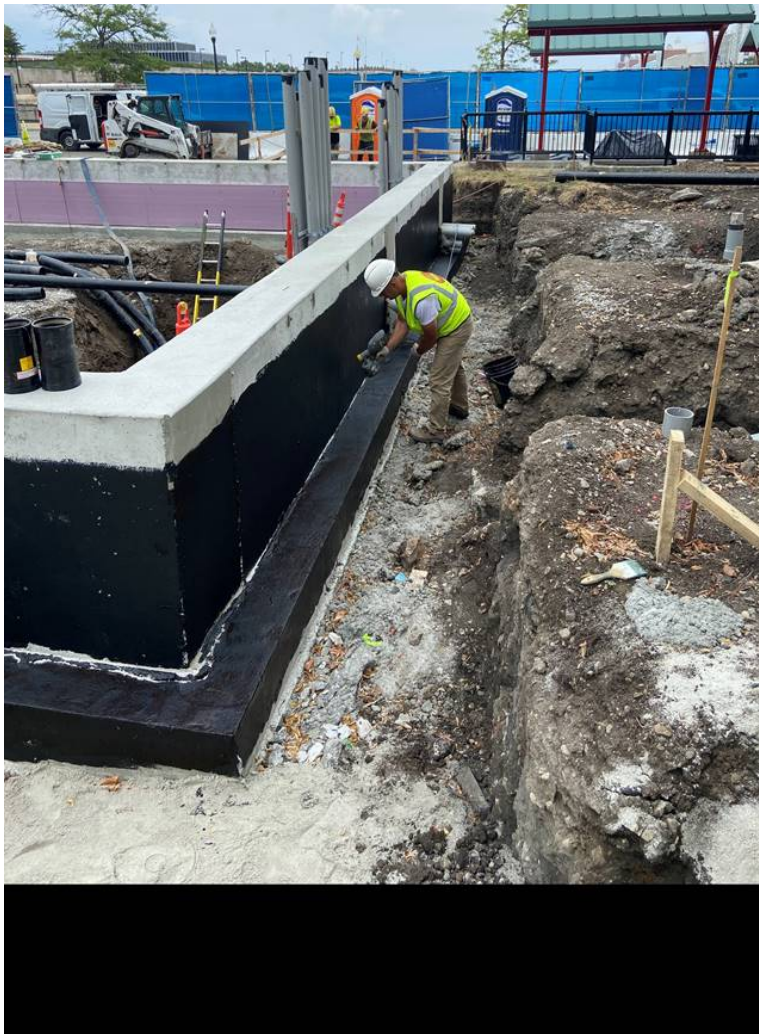
Building Foundation and Waterproofing
