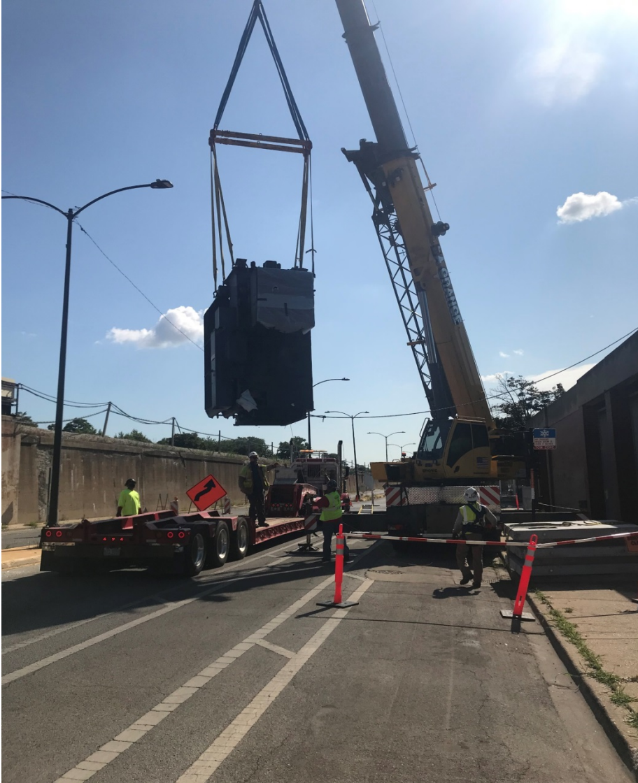
Removal of Transformer 1 at Lotus Substation
