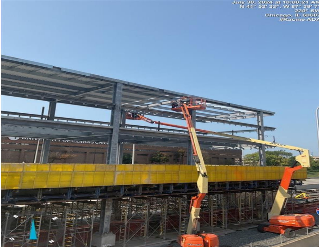
Morgan Substation Installing Roofing Panels
