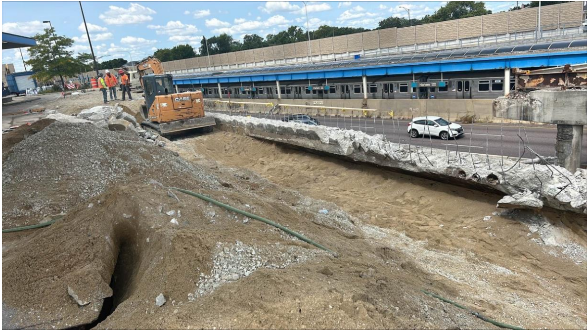
Demolition South Approach Slab Near Bus Canopy
