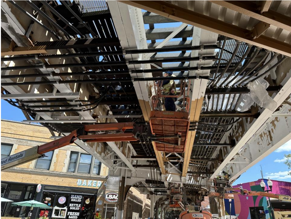
Painters Applying Prime Coat over Lincoln Avenue
