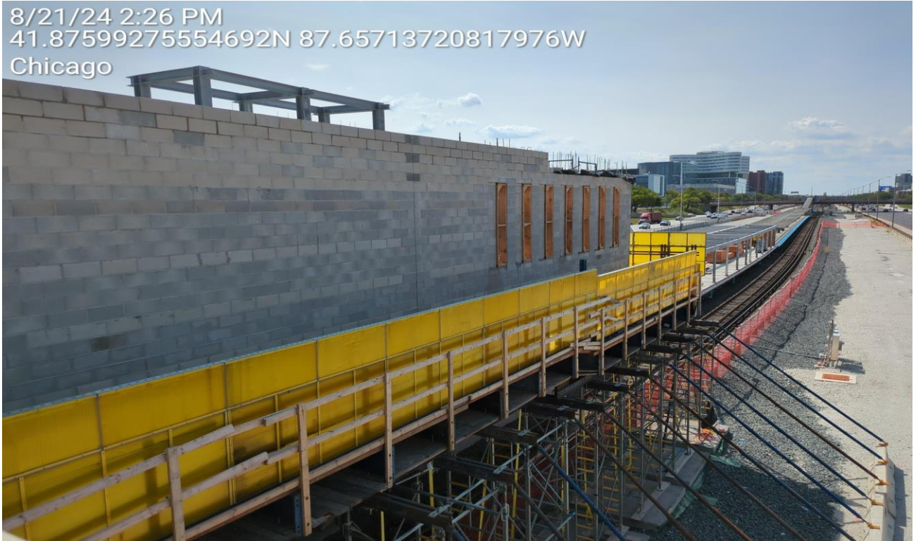
Racine Stationhouse North CMU Wall
