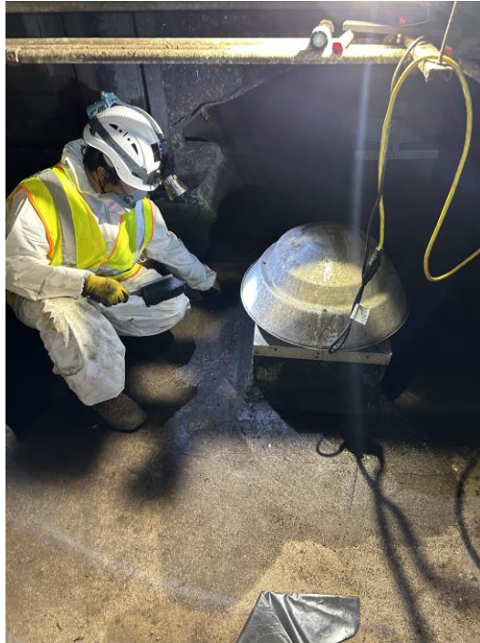
Environmental Mitigation on Roof of Station House
