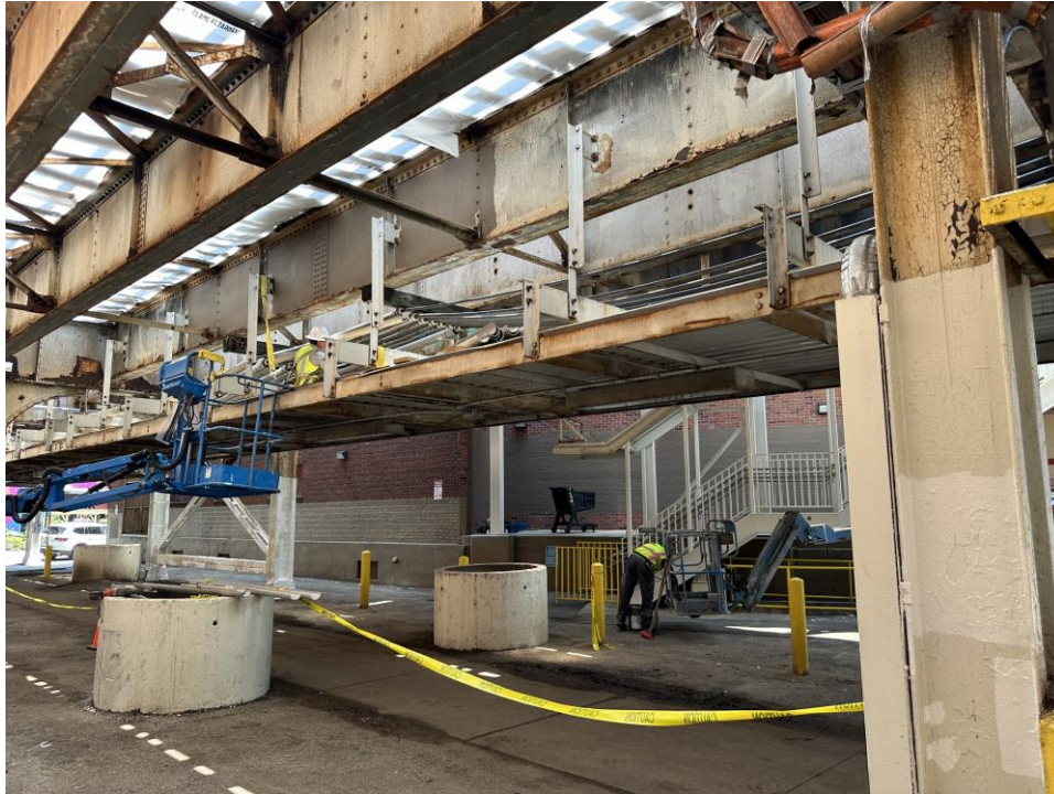
Insulating Traction Power Cables Ahead of Painting
