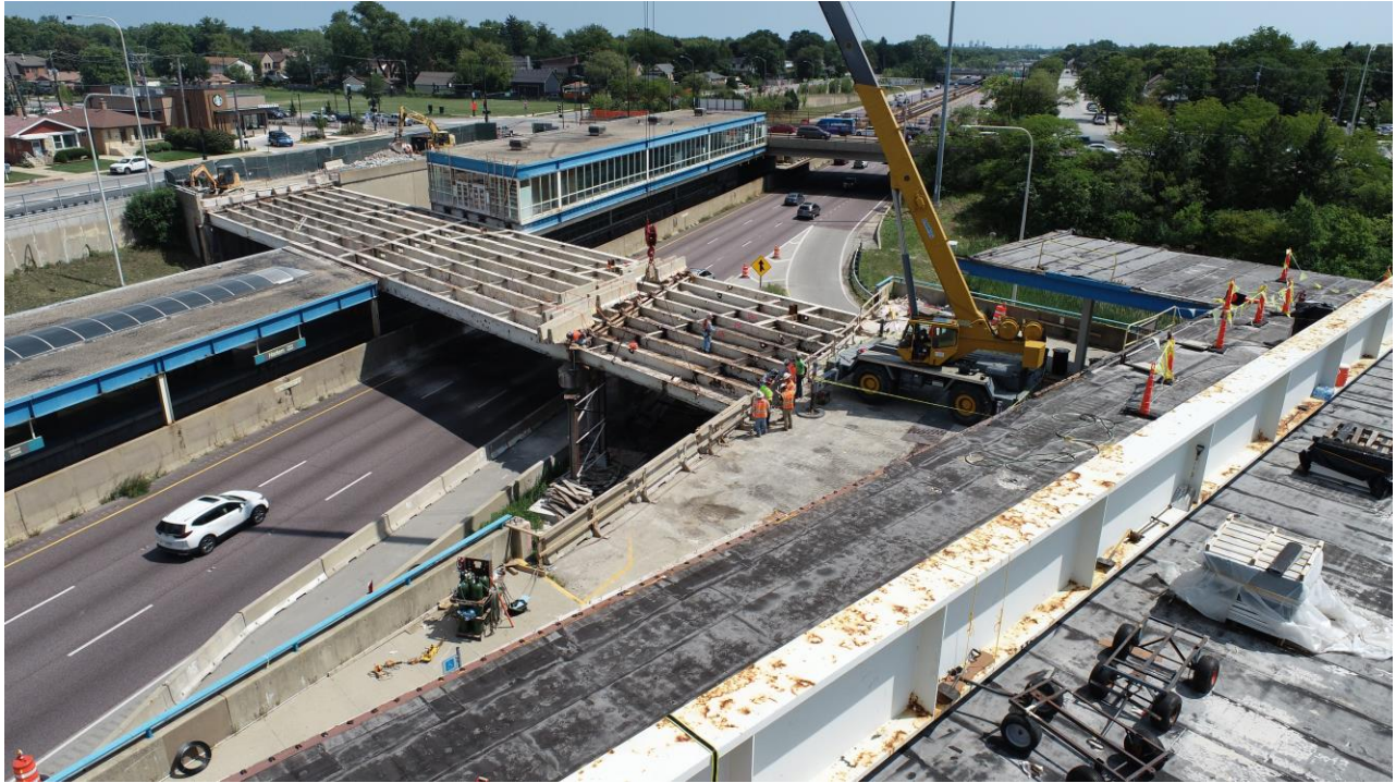
Aerial View of Bus Bridge Steel
