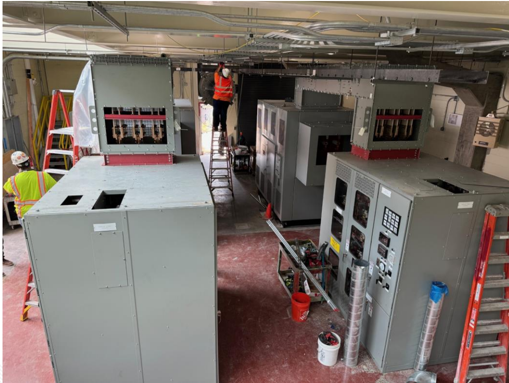
Traction Power Equipment Installation at Damen
