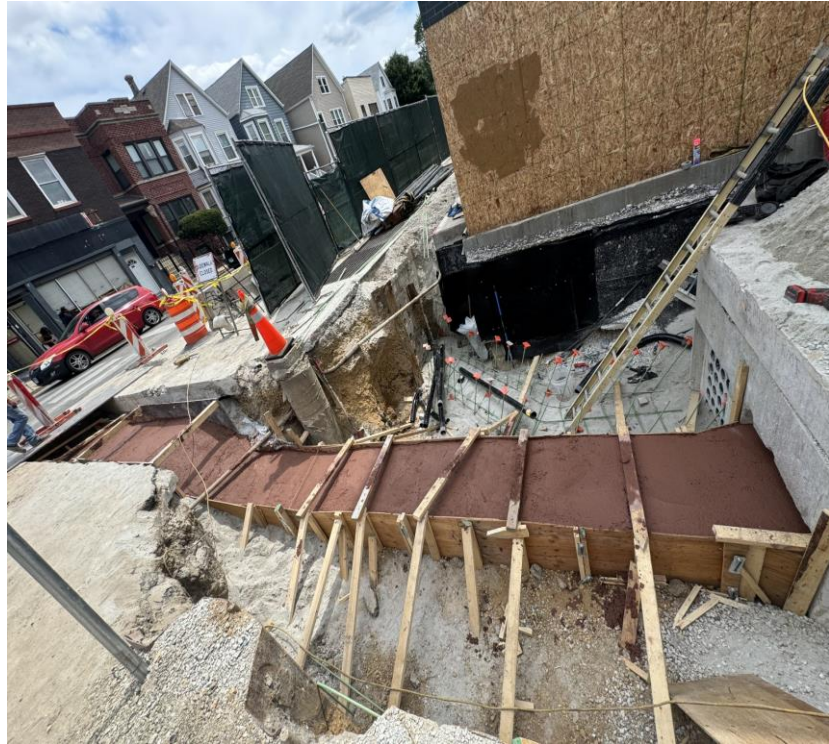
Ductbank Installation at Barry
