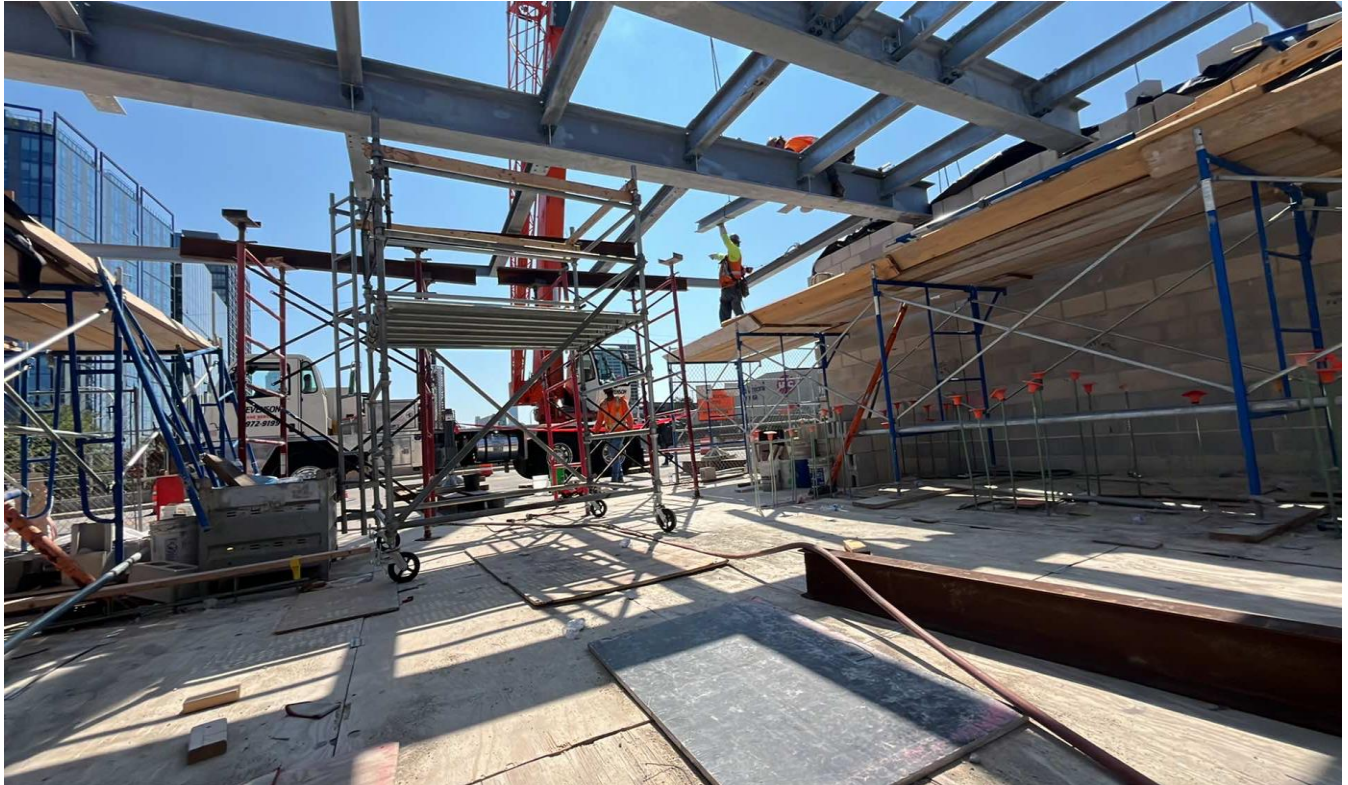
Racine Stationhouse Steel Beams Roofing
