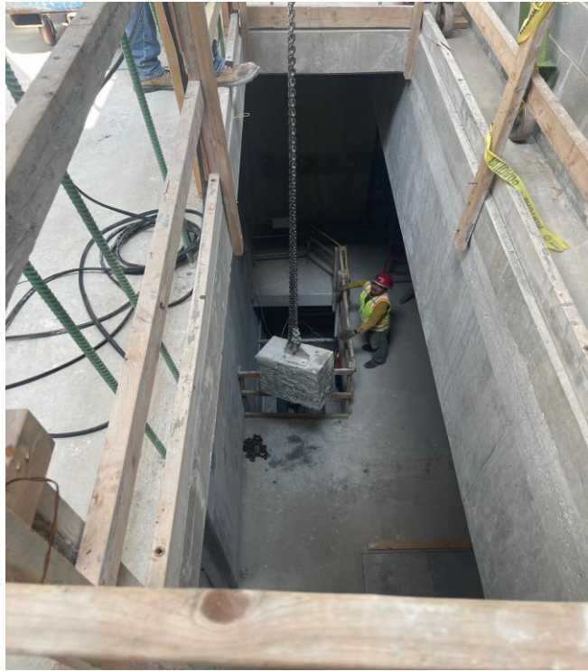
Sub-Vault Floor Demolition at Barry
