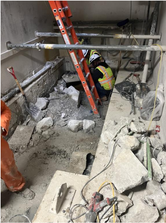
Sub-Vault Floor Demolition at Barry
