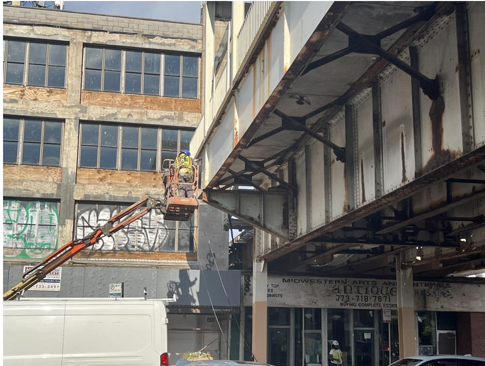
Painters preparing steel over Western Avenue
