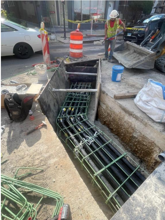
Ductbank Installation at Barry
