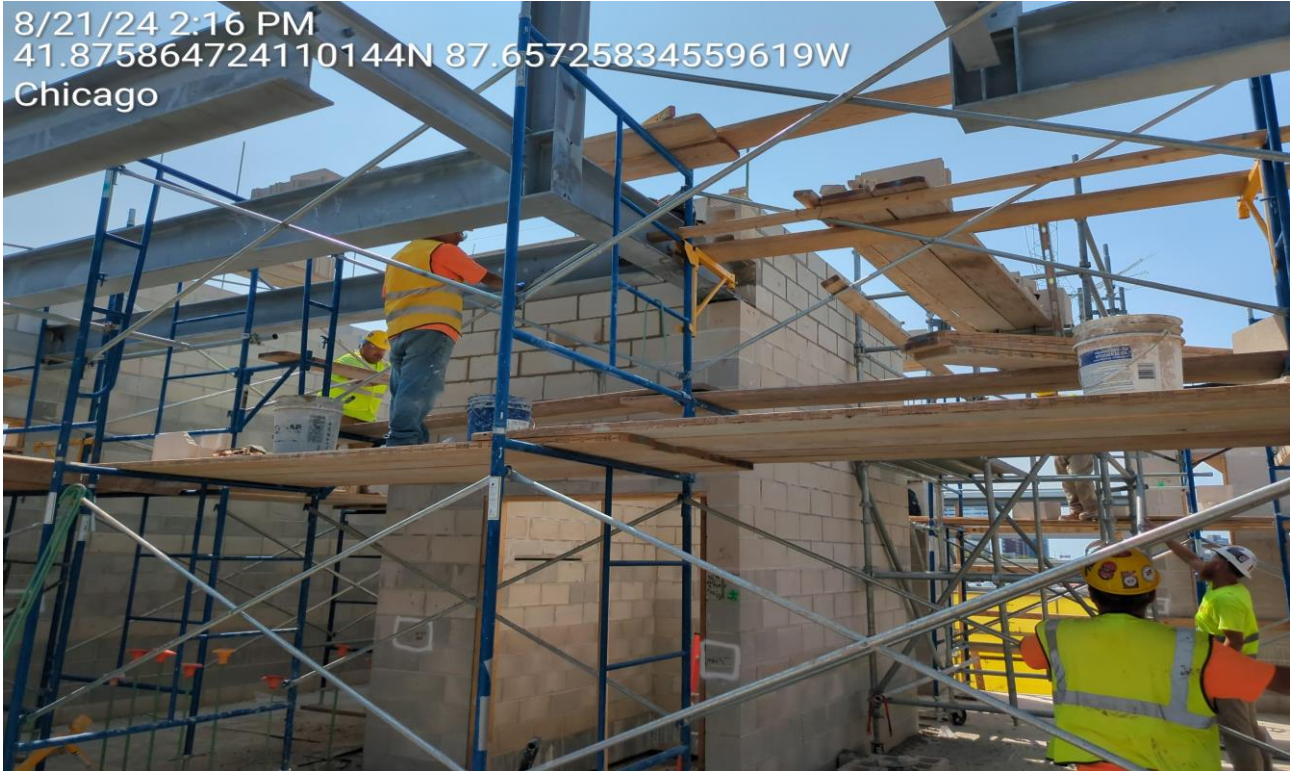
Racine Stationhouse Interior Elevator Core Walls
